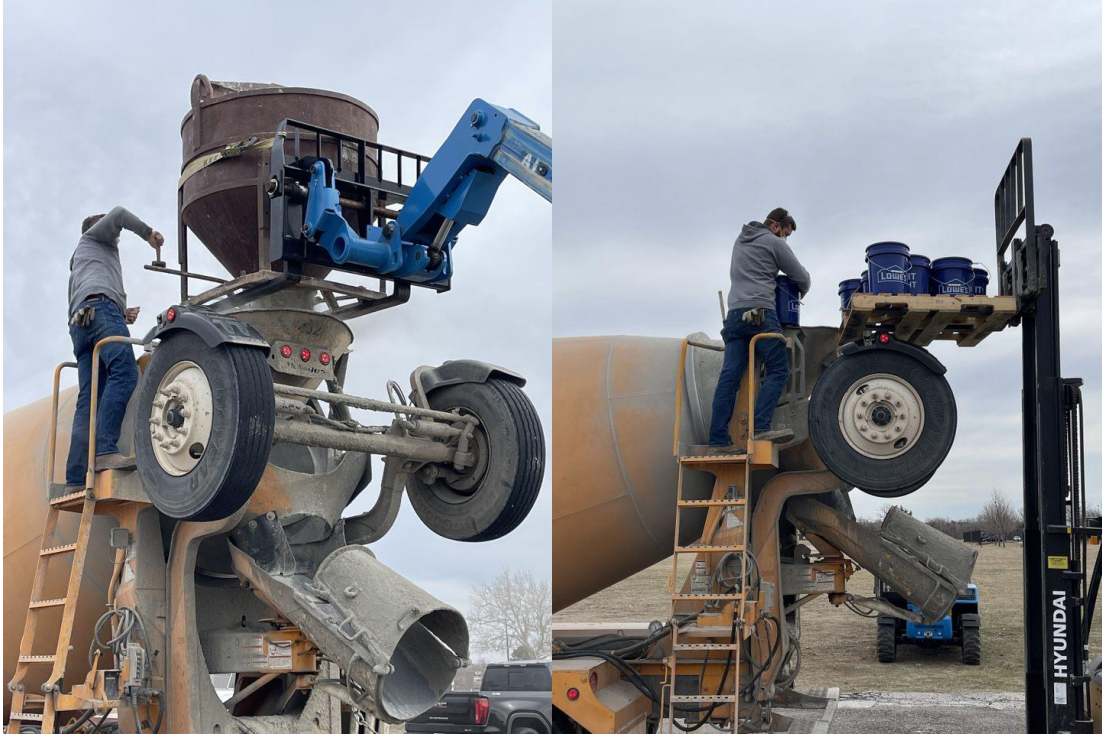
Figure 100: Addition of the Expansive BCSA Cement (left) Followed by Buckets of the Remaining Water, Dosed with Second Half of the Citric Acid and HRWR (right)
