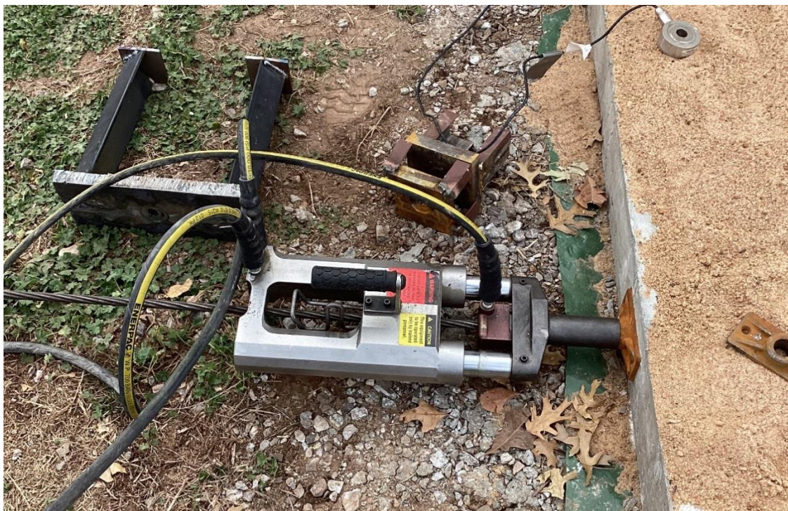
Figure 30: Post-Tensioning of Standard Single Anchorages
