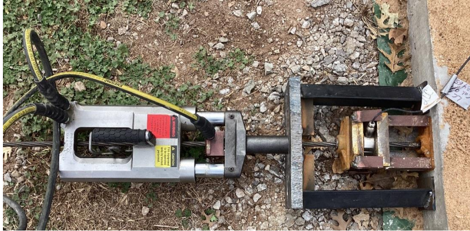
Figure 29: Post-Tensioning Jack Bearing Against Unloading Frame Used to Remove Load Cell
