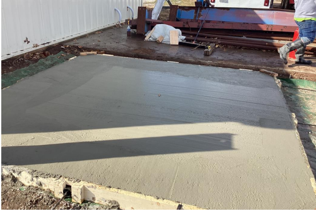
Figure 106: Final Finish of Slab after Bull Floating
