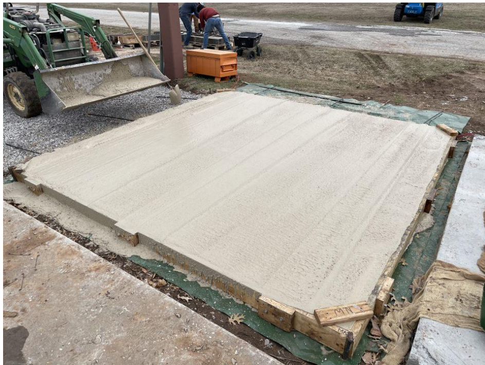
Figure 105: Rough Finish of Slab after Screeding
