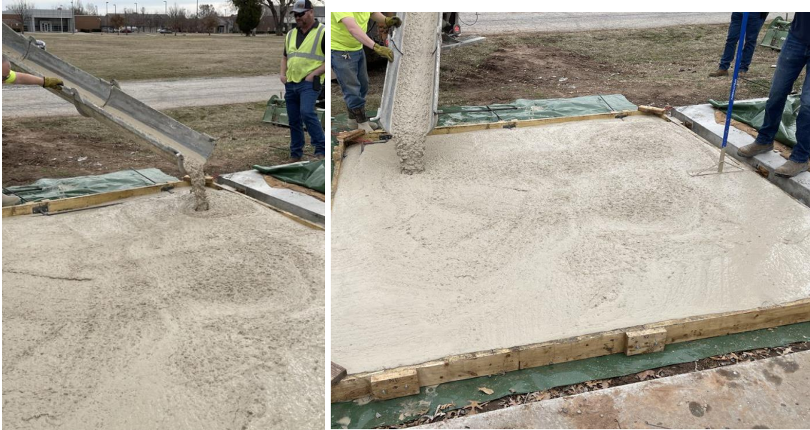
Figure 102: Slowly Using the Mixer Truck Chute to Fill the Slab Forms
