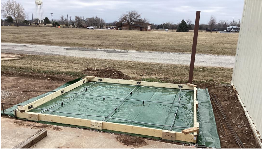
Figure 26: Final Site Preparation with Formwork and Vapor Barrier Laid Out.
