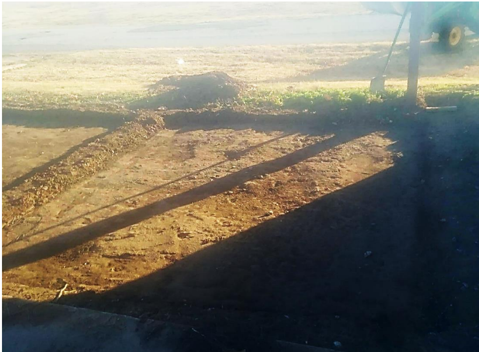
Figure 23: Site Graded to -9" with Embankments Around the Edges Added to -5"
