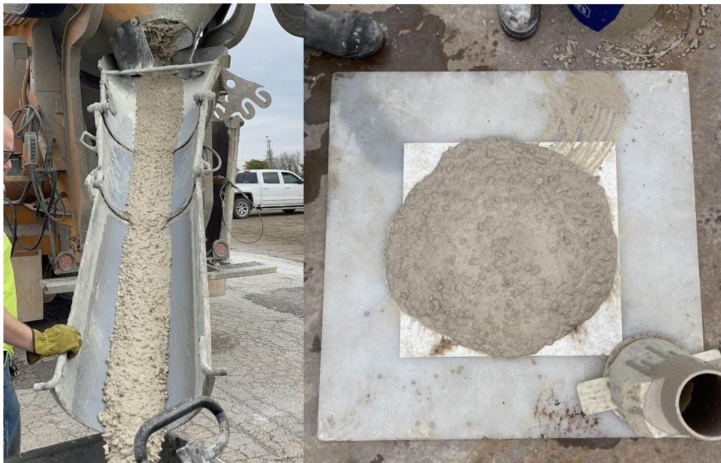
Figure 101: Filling a Buggy with Final Expansive BCSA Mix and Taking a Slump Measurement
