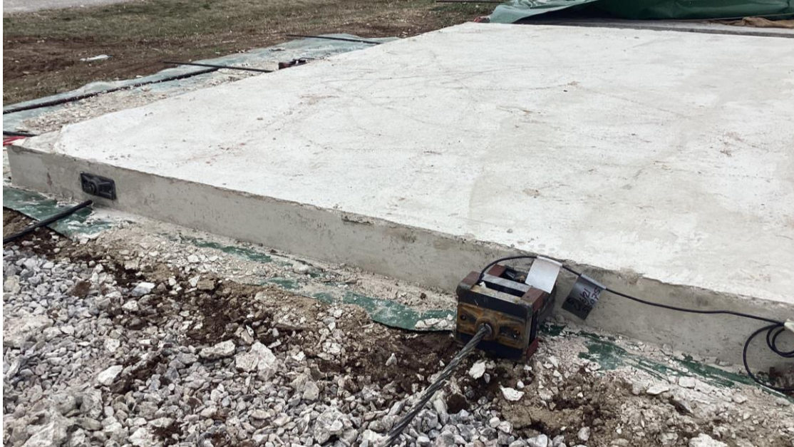
Figure 108: Loaded Post-Tensioning Double Anchorage used for Placement of the Load Cell
