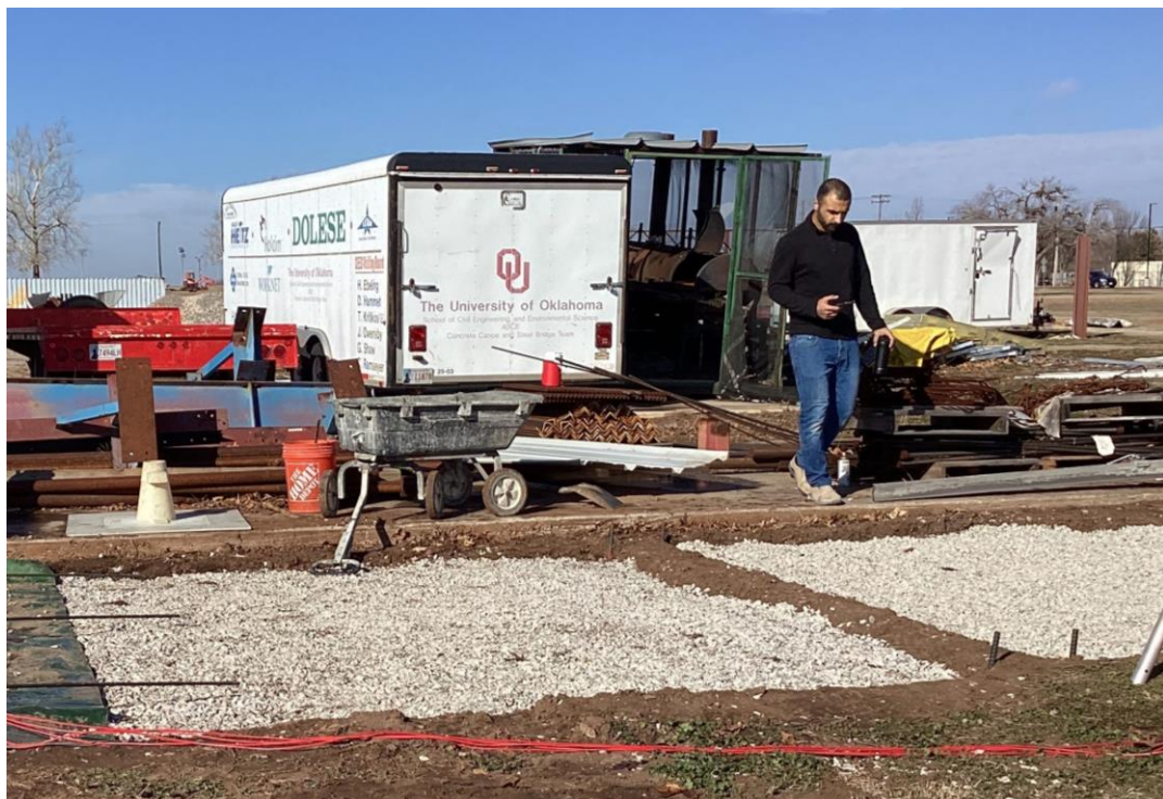
Figure 25: Final Compacted Site Material
