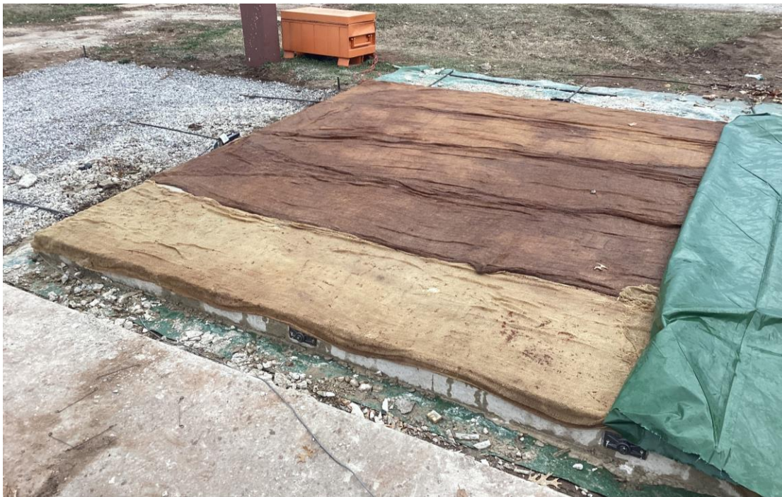
Figure 109: Wet Curing of Slab after Post Tensioning Using Wet Burlap Covered with Plastic
