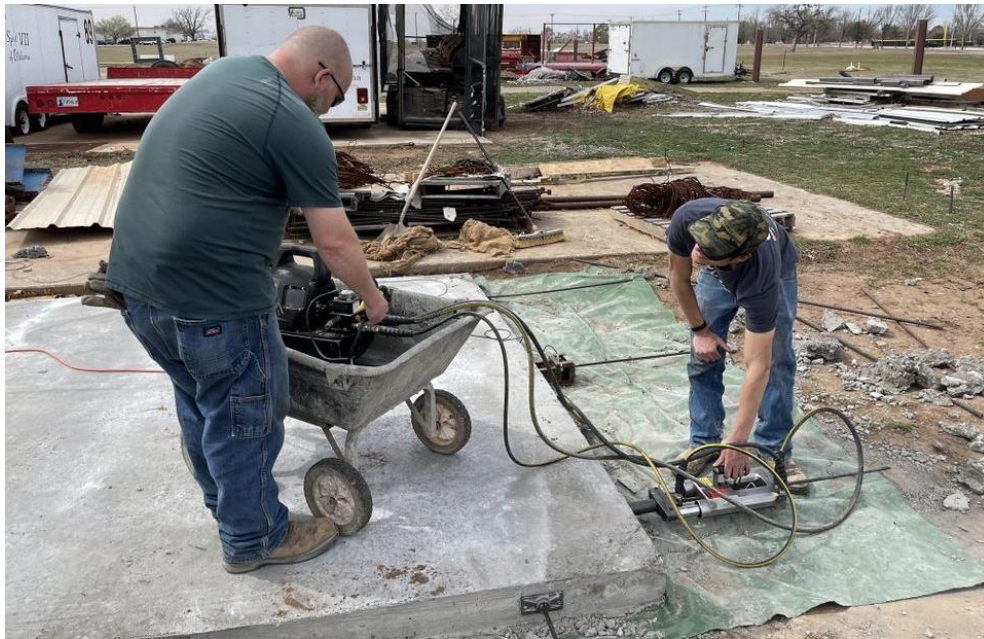
Figure 107: Post-Tensioning the Slab
