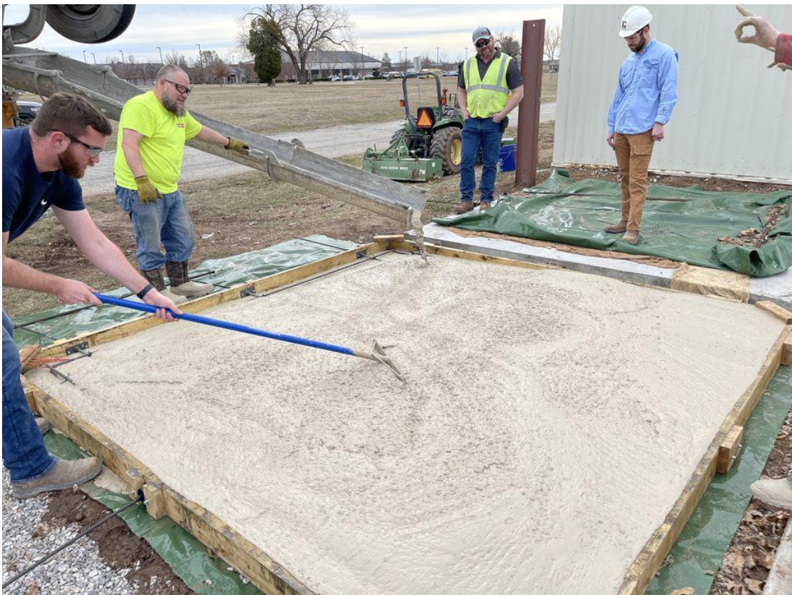
Figure 103: Raking the Concrete as it Comes Out of the Chute to the Approximate Slab Elevation
