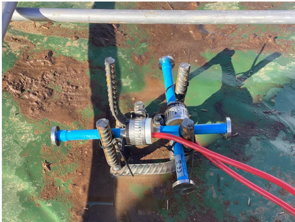
Figure 22: Rebar Tree used to Place and Mount VSWG Gauges Instrumenting the Slabs
