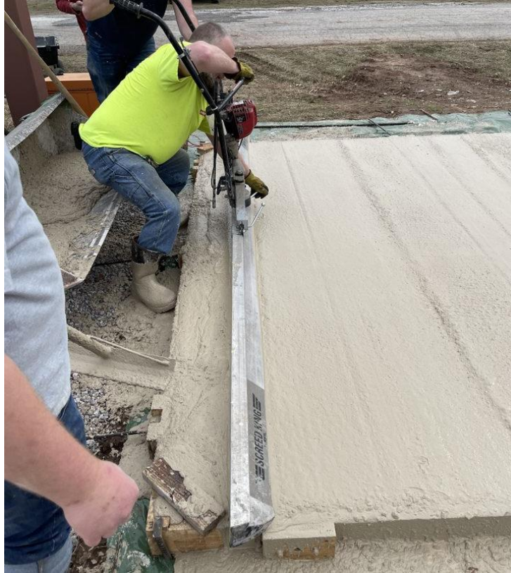
Figure 104: Using a Power Screed to Roughly Finish the Slab to the Proper Slab Elevation
