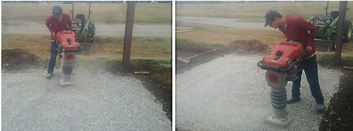
Figure 24: Compaction of the #67 Coarse Aggregate Base
