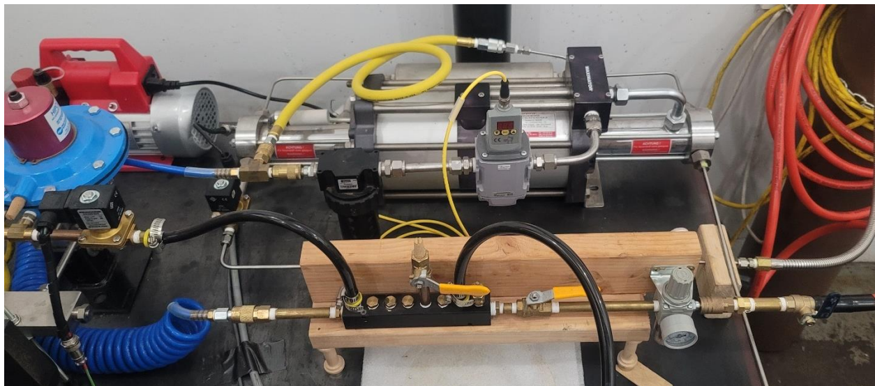
Figure 35: As-Built Test Stand Control Air Manifold and Intensifier
