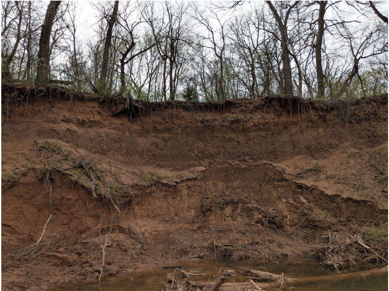
Figure 6.29. Sandy Creek Cutbank Two.
