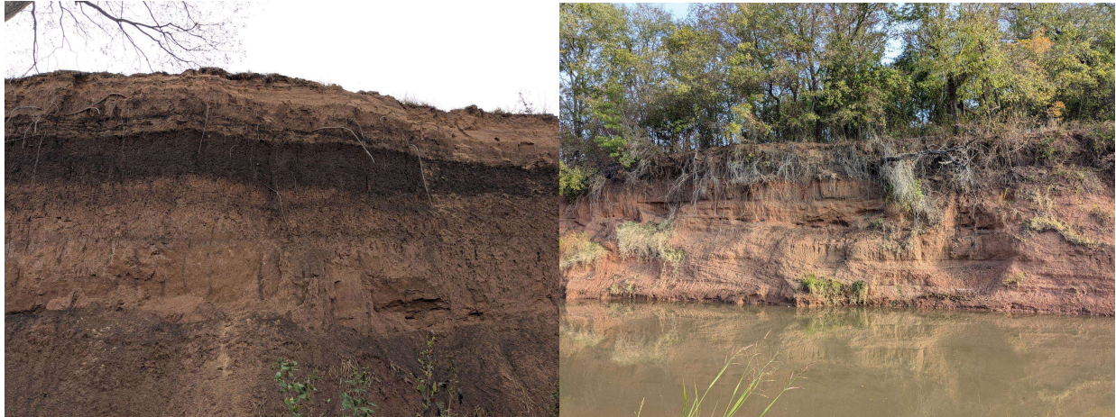
Figure 6.15. Overviews of the Wildhorse Three cutbank and surrounding locale
