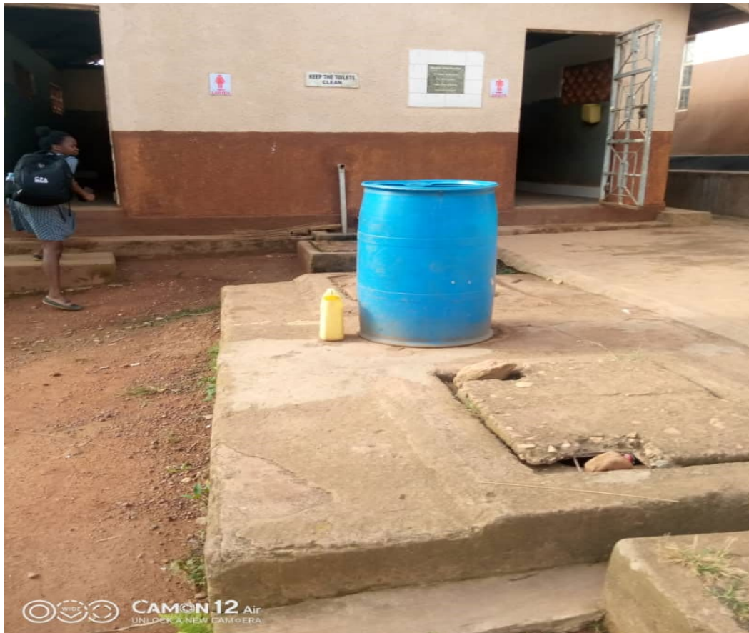
Figure 4: A yellow 3-liter jerrycan used to scoop water from a 100L water barrel beside it for flushing the toilet
