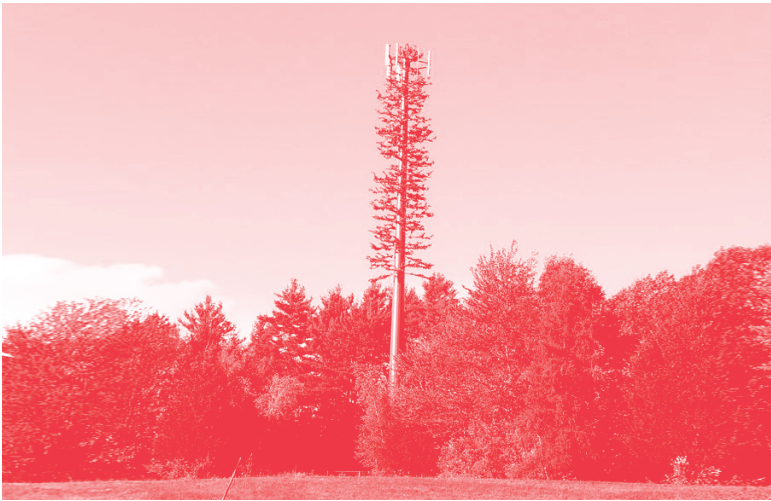
Image courtesy of 99% Invisible Cell tower disguised as a tree
