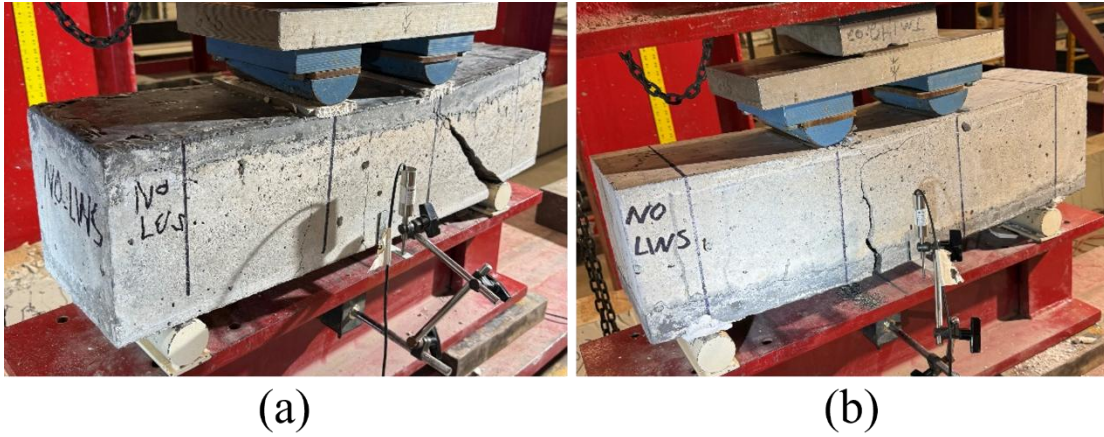
Figure 3.23: Failure of 8 in. x 8 in. x 30 in. UHPC-0LWS overlay beams with (a) overlay in compression and (b) overlay in tension
