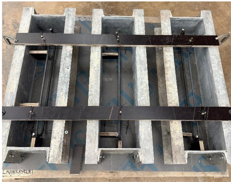
Figure 3.9: Overlay beam formwork with the reinforcement and spacers in place
