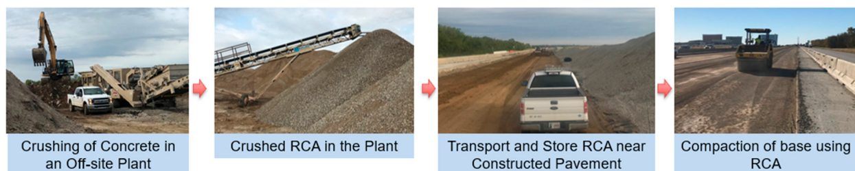
Figure 2. Overview of operation used to produce RCA from highway concrete pavement.
