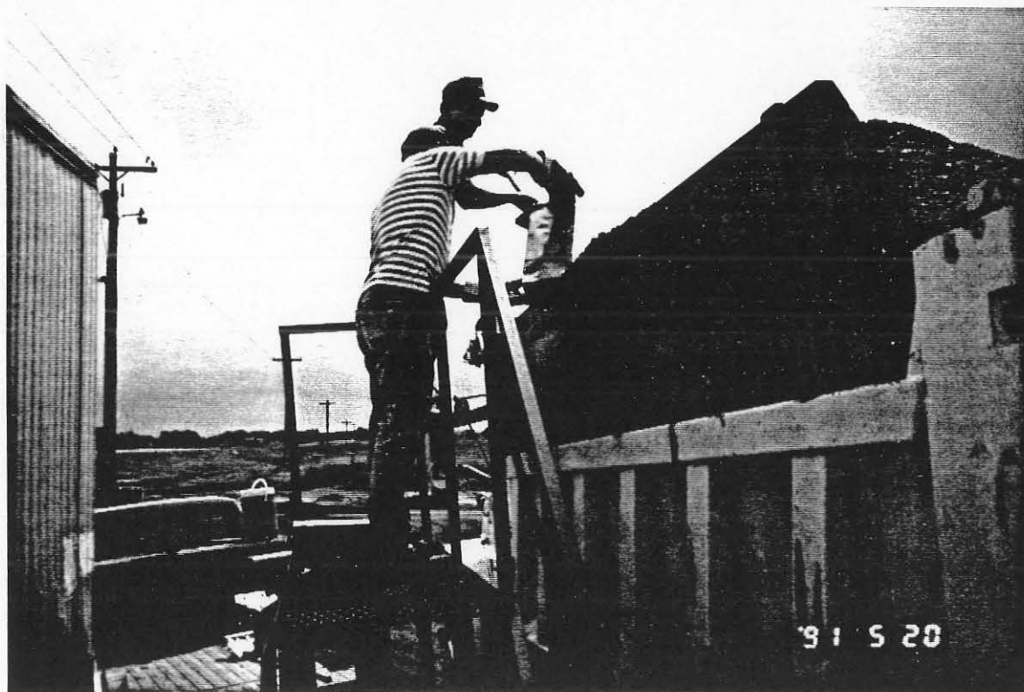
Figure 7. Another Photograph of Sampling Fresh Mixture
