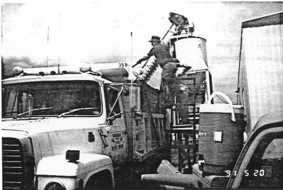
Figure 6. Sampling Fresh Mixture from Hauling Truck
