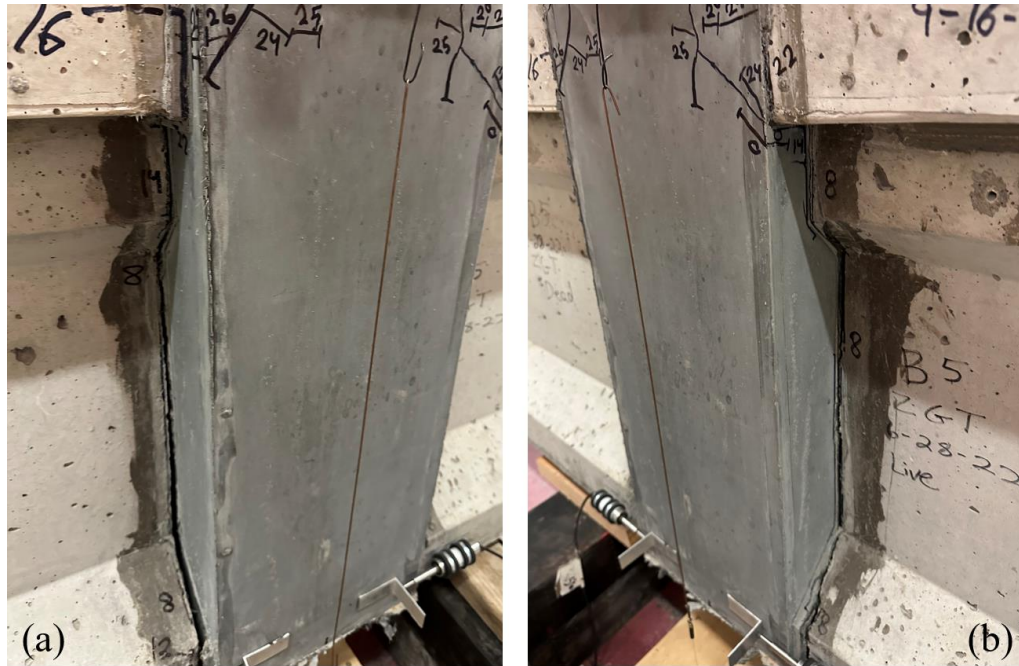
Figure 74: Southeast (a) and northeast (b) side of joint SSDU-1 showing cracking along the interfaces under final positive moment test loading
