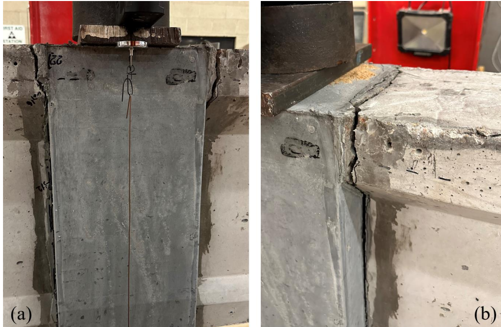
Figure 62: East (a) and southeast (b) side of joint HSDU-2 showing cracks at the interface before negative moment testing
