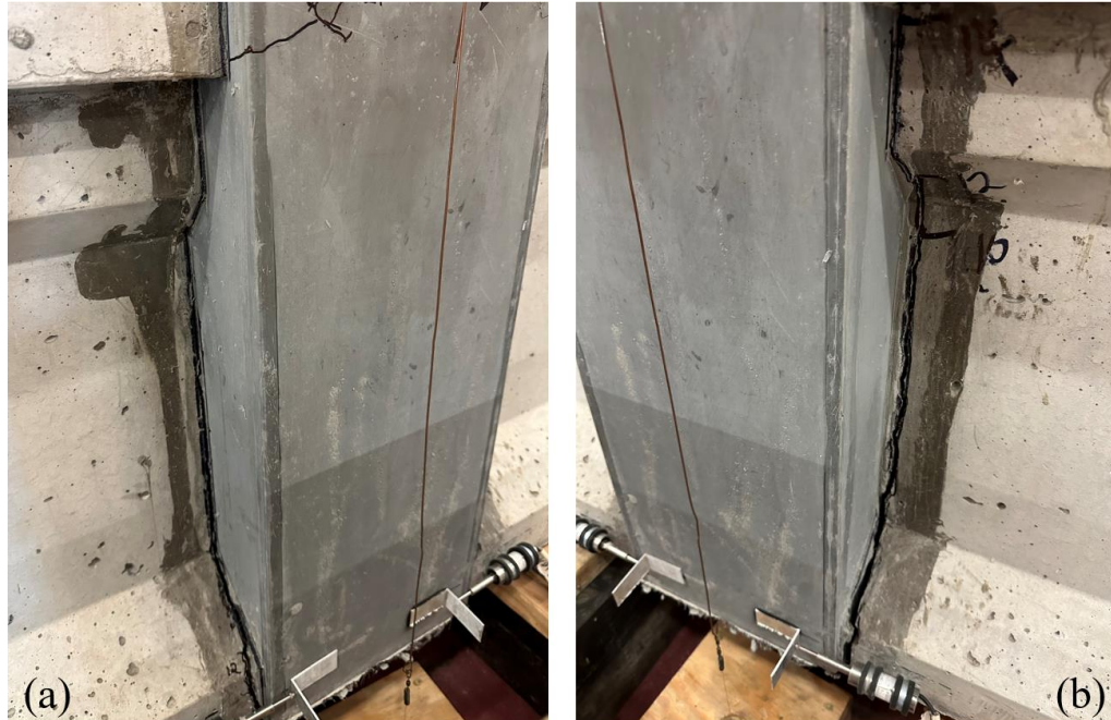
Figure 75: Northwest (a) and southwest (b) side of joint SSDU-1 showing cracking along the interfaces under final positive moment test loading
