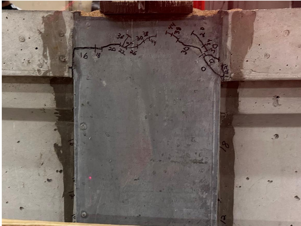
Figure 58: Cracking on the west side of HSDU-2 near the as-cast top surface of the joint
