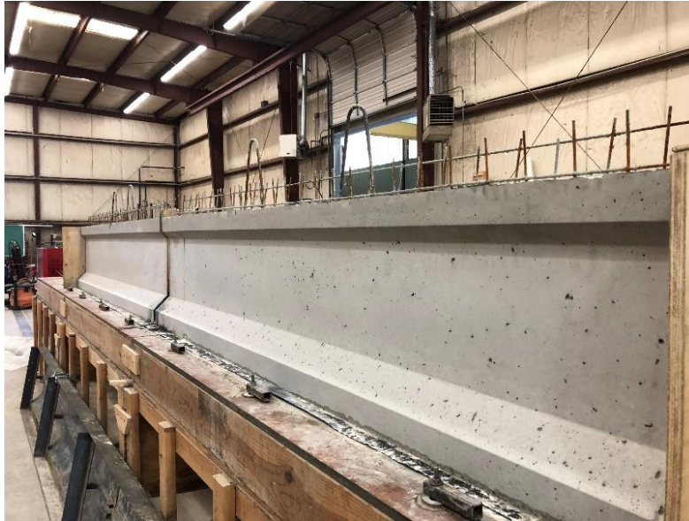
Figure 10: Two prestressed girders simultaneously cast on the prestressing bed
