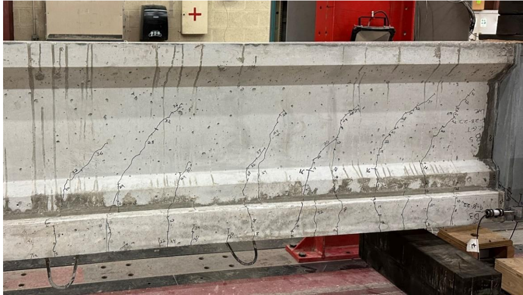
Figure 84: West side of north girder SSDU-1 showing flexural cracks as after negative moment test
