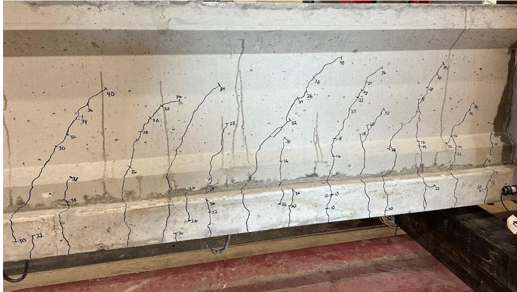
Figure 94: West side of north girder of SSDU-2 showing flexural cracks under final negative moment test loading
