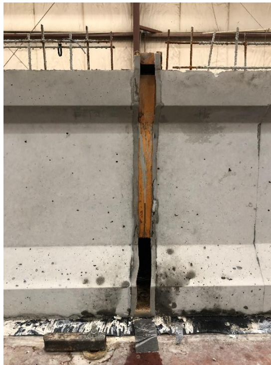
Figure 11: Wooden divider between adjacent girders
