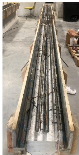
Figure 14: Deck reinforcement placed in formwork
