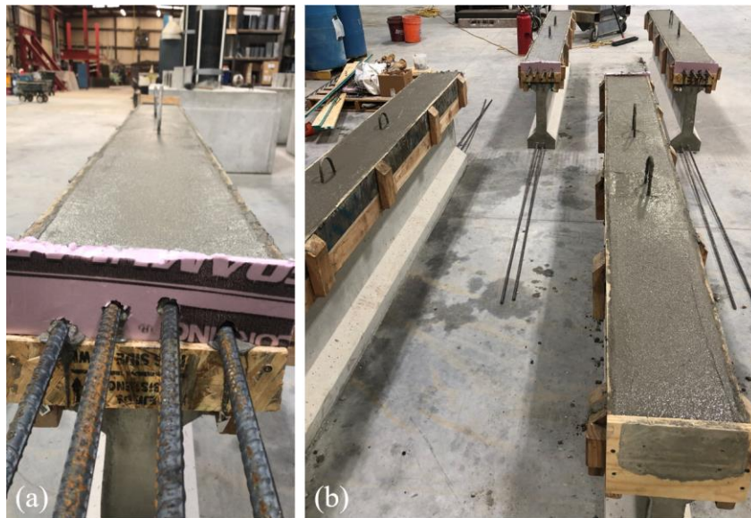
Figure 15: Freshly placed deck concrete showing a close-up of the forms around the lap splice (a) and an entire set of specimens (b)
