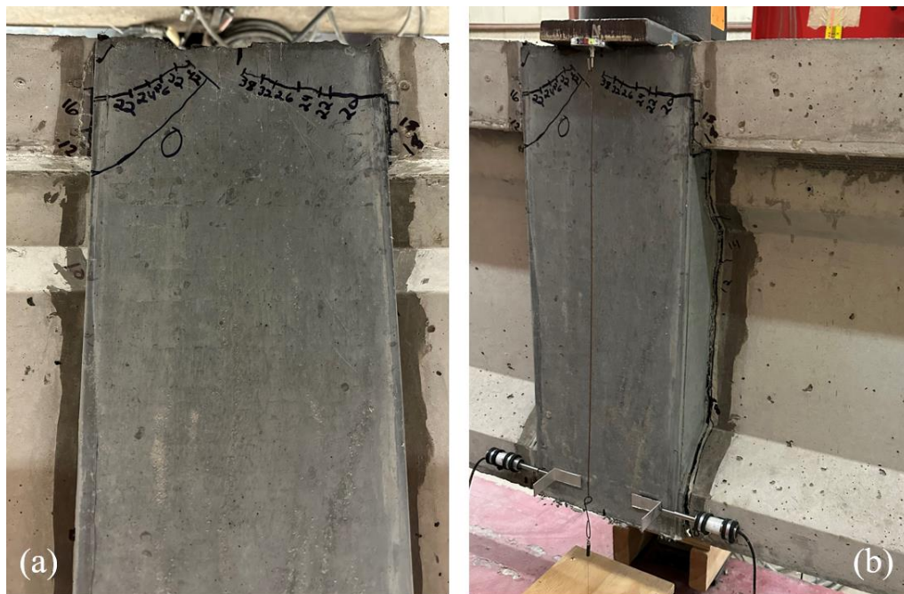
Figure 46: East side of joint (a) and northeast interface (b) of HSDU-1 after positive moment test
