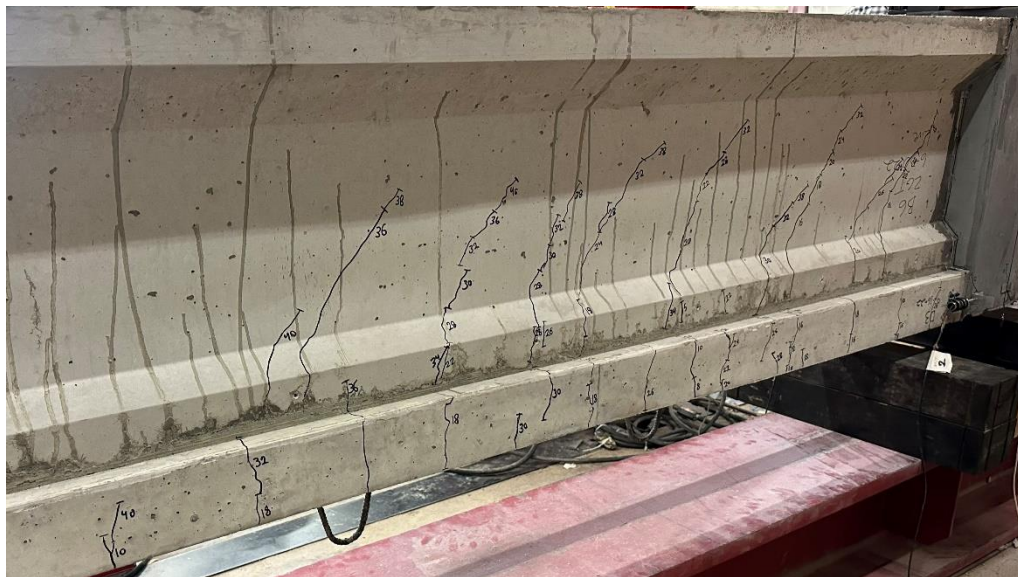
Figure 93: East side of south girder of SSDU-2 showing flexural cracks under final negative moment test loading
