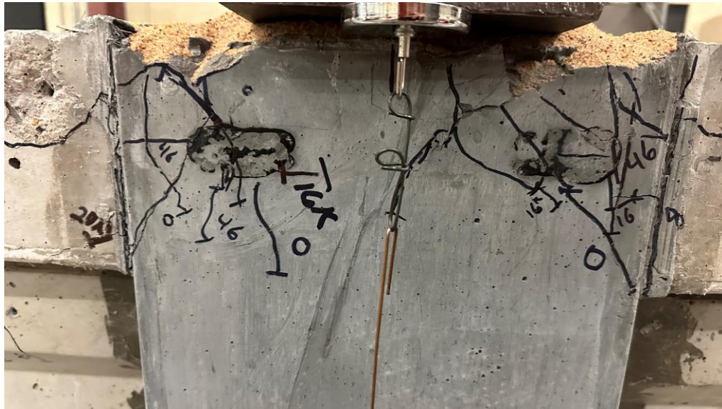
Figure 104: West side of joint SSDU-2 showing cracks near as-cast top face after final positive moment test loading
