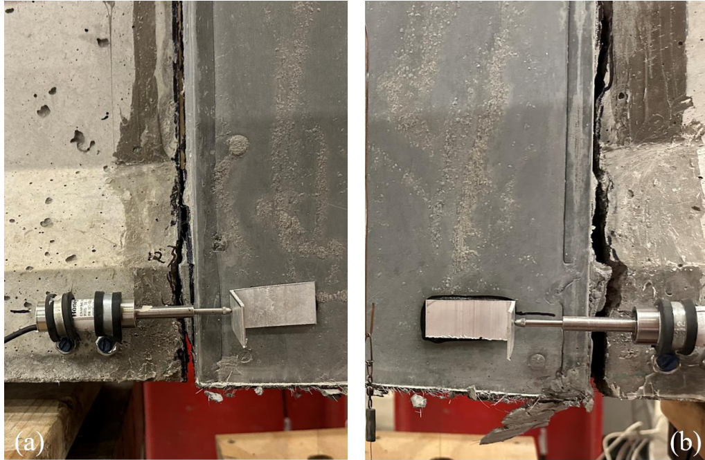
Figure 77: Northwest (a) and southwest (b) side of joint SSDU-1 showing separation at the interface near the as-cast bottom face under final positive moment test loading
