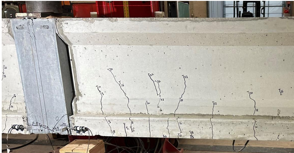
Figure 51: Flexural cracking on northeast side of specimen HSDU-1 under final negative moment test loading
