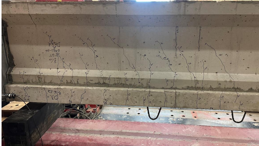
Figure 92: East side of north girder of SSDU-2 showing flexural cracks under final negative moment test loading
