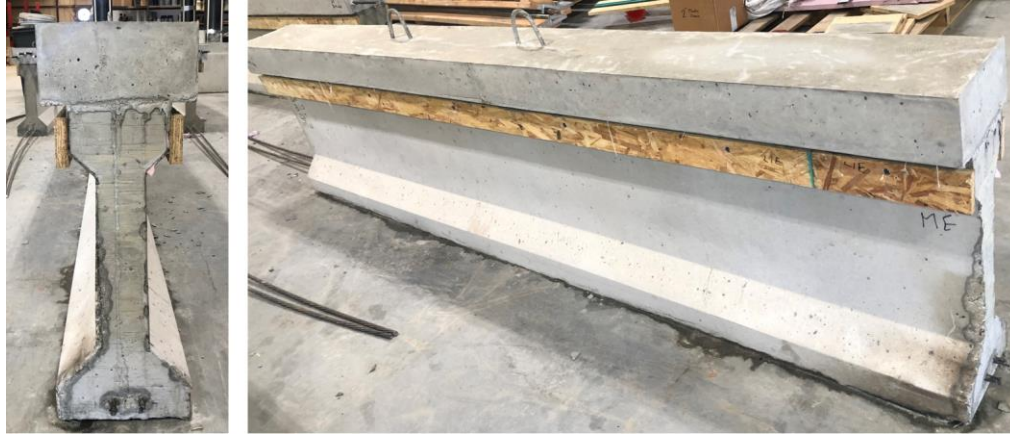
Figure 16: Finished concrete decks after form removal
