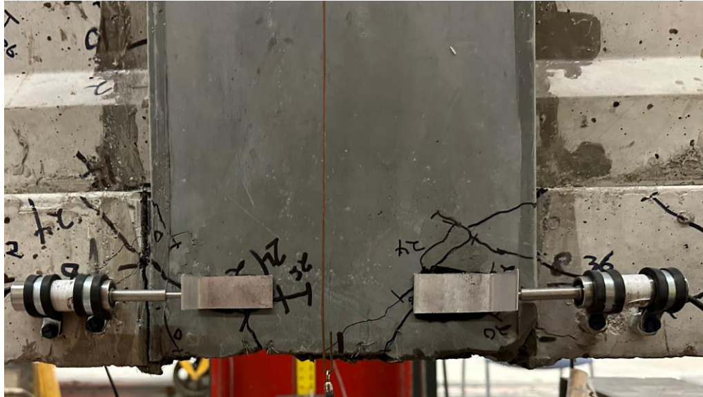
Figure 87: East side of joint SSDU-1 showing cracks near the as-cast top face of the joint under final negative moment test loading
