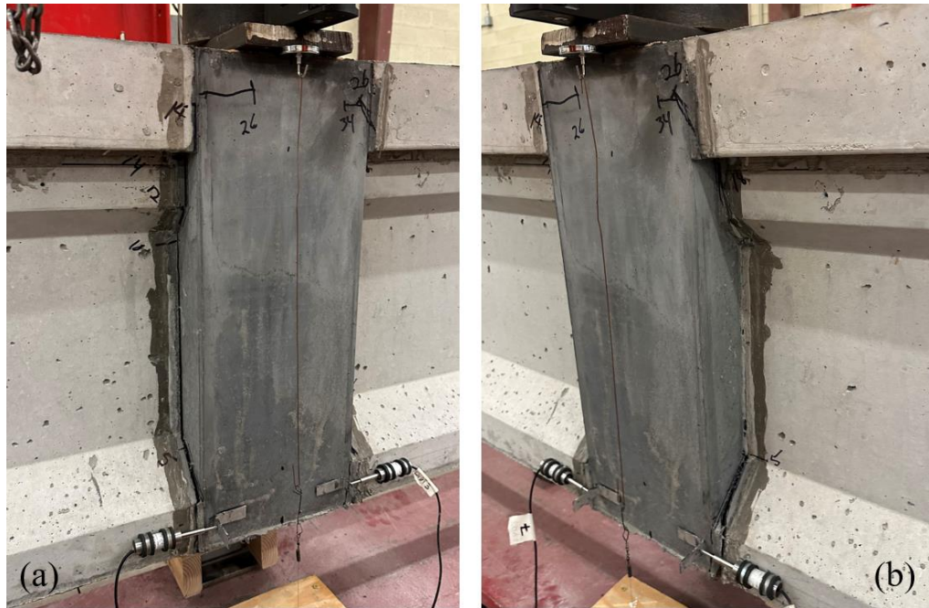
Figure 35: Northwest (a) and southwest (b) side of the joint HSJ3-2 after testing
