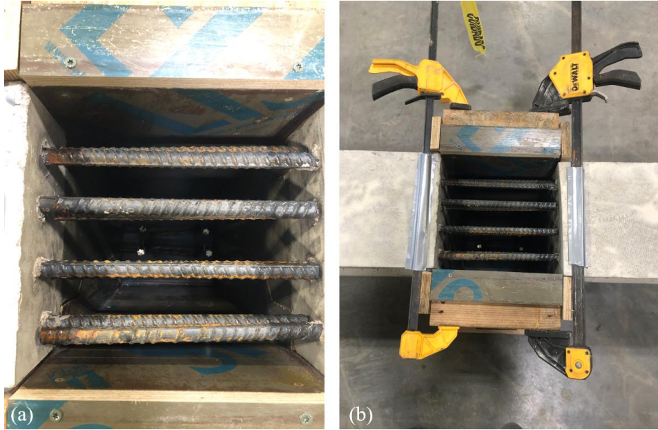
Figure 22: Plan views of joint formwork secured in place showing a close-up of the reinforcement (a) and zoomed-out view of the restraints (b)
