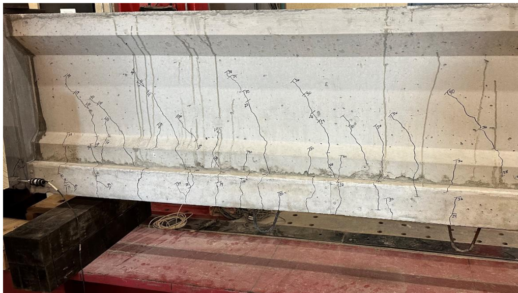
Figure 95: West side of south girder of SSDU-2 showing flexural cracks under final negative moment test loading
