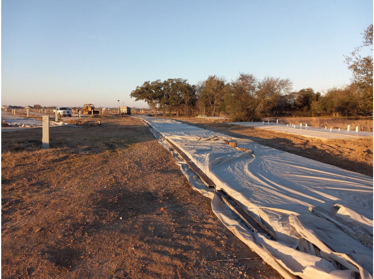
Figure 4-6 A concrete roadway that was cured with Pulp Cure and then covered with plastic.
