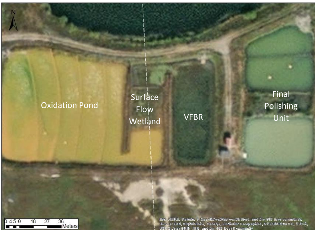
Figure 1.3: Southeast Commerce Passive Treatment System with Treatment Units Labeled
