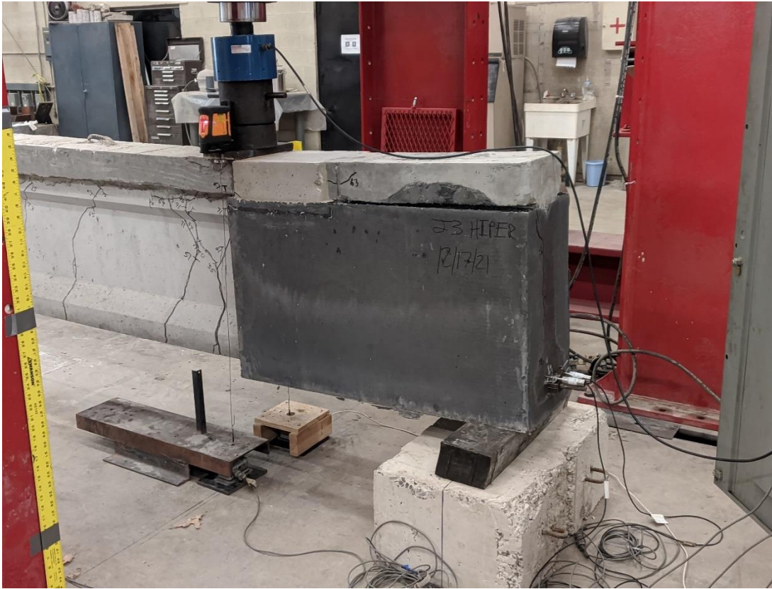
Figure 77. Repaired girder with cracks after loading to failure.
