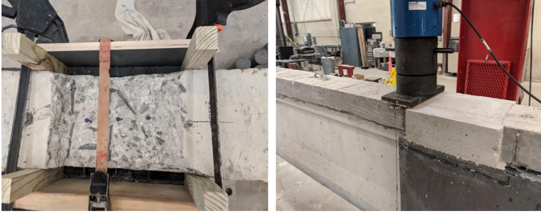
Figure 18. Repaired deck section using belitic calcium sulfoaluminate cement.
