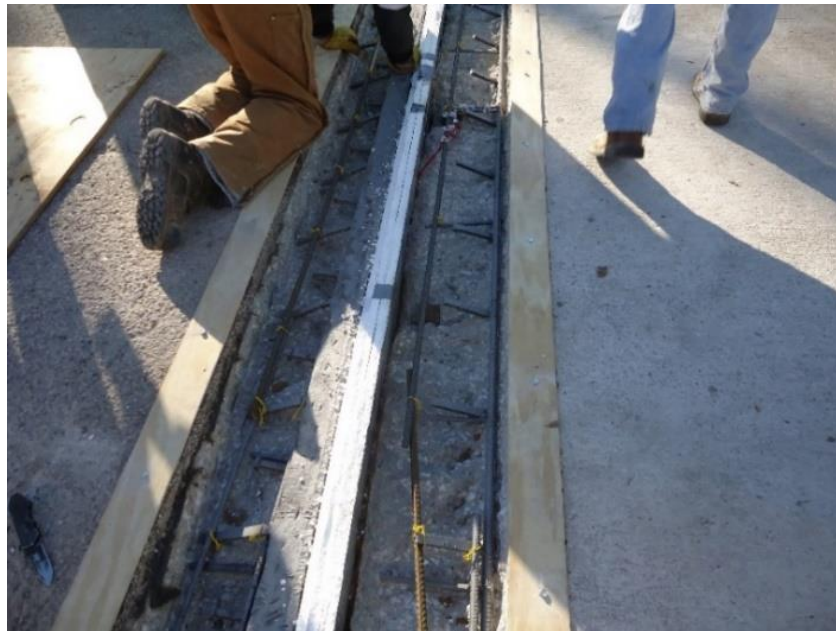
Figure 70. Joint after removal of existing concrete and before placement of the top form
