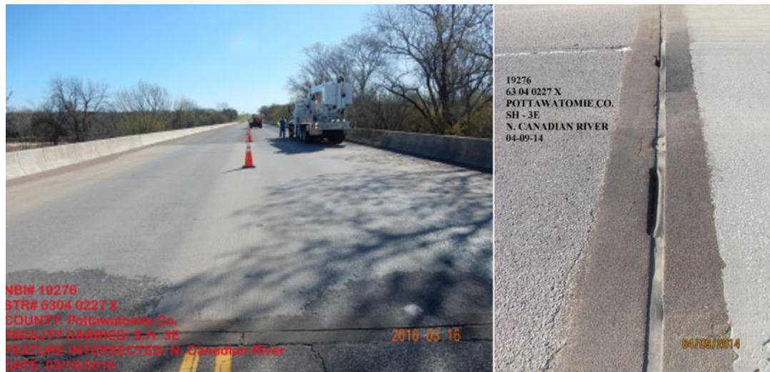
Figure 66. SH-3 bridge over N. Canadian River (left) and expansion joint to be replaced (right)
