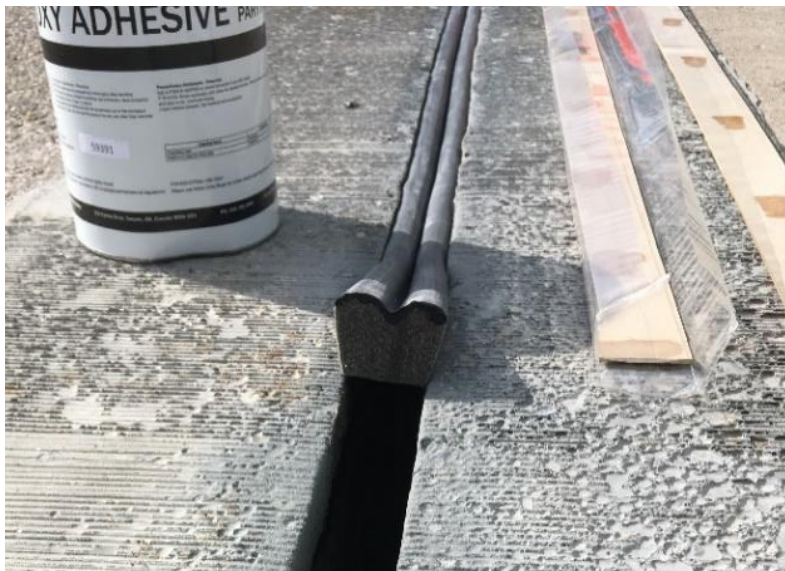
Figure 76. End of BEJS stick prepared for splicing
