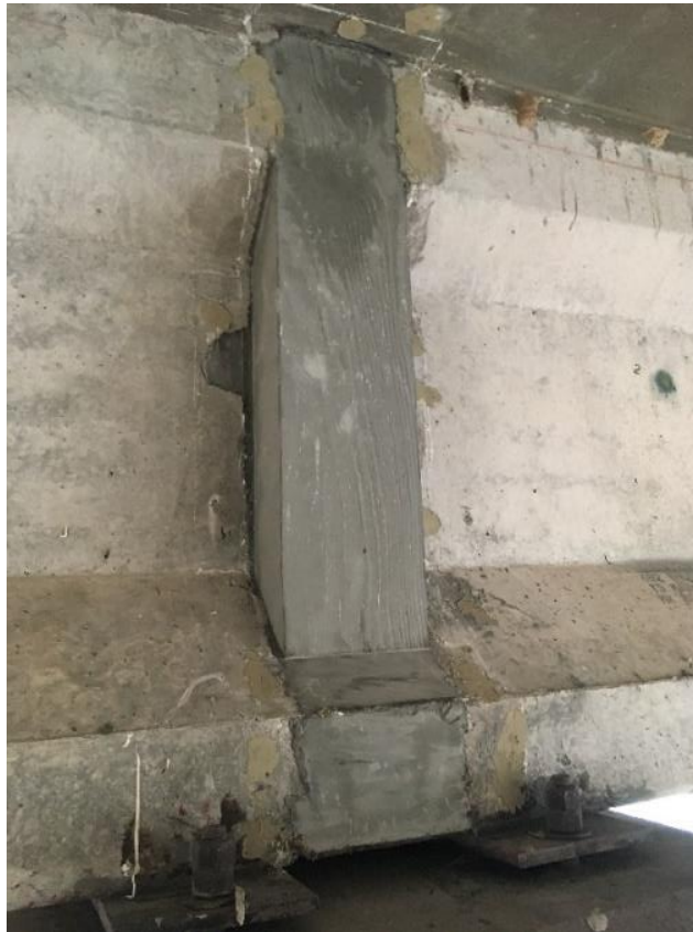
Figure 95. Completed UHPC continuity joint after form removal
