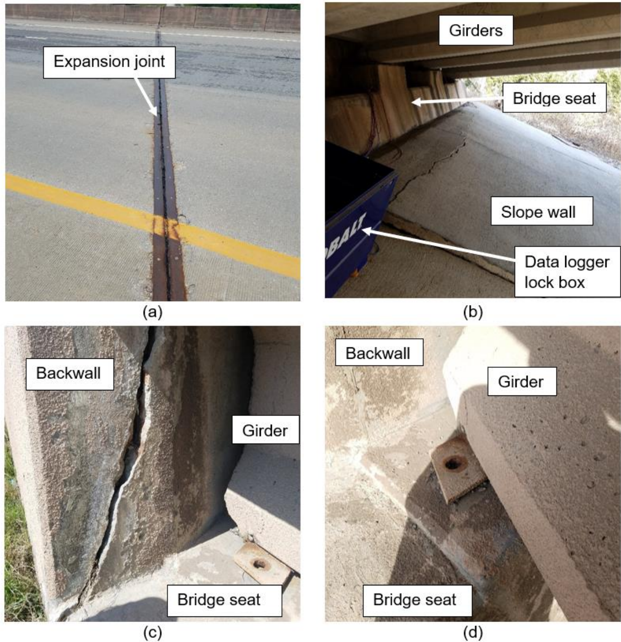
Figure 101. SH-3 over BNSF: Bridge distress (a) closed expansion joint, (b) buckled slope wall, (c) cracked backwall, (d) sheared anchor bolt
