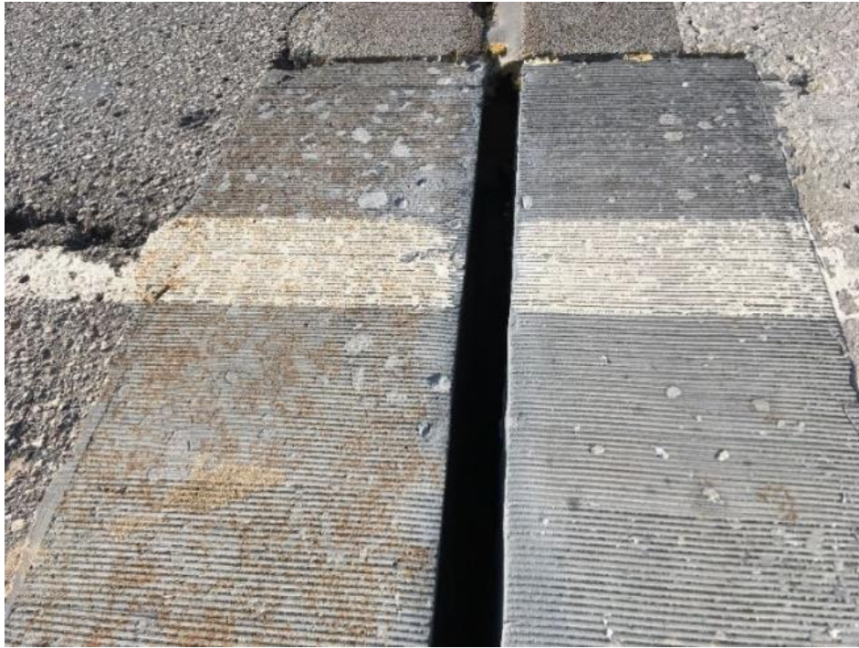
Figure 79. UHPC joint headers on SH-3E bridge before joint sealant was placed and showing surface rusting of the exposed steel fibers
