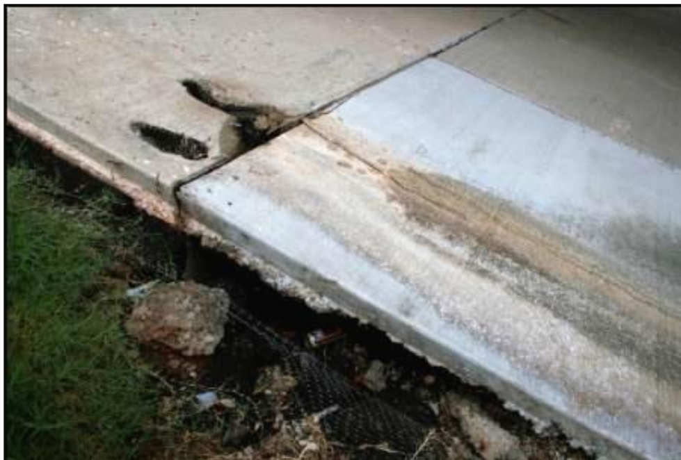
Figure 122. Water flowing from underdrain outlets onto slope wall, Tecumseh Rd. over I-35. (note large void under slope wall)
