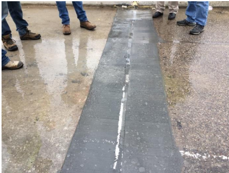
Figure 74. Entire Joint after grinding
