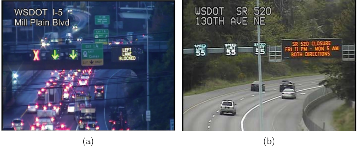
Figure 1.6: Examples of the ATDM system corridors installed by WSDOT along Washington Highways [24]. a) Along Interstate 5 in Vancouver, the implementation of four DMS can be observed, with three of them displaying lane availability and the last one showing text information. b) On Highway 520 between Seattle and Bellevue, the implementation of four DMS can be observed, with three of them functioning as VSLs and the last one displaying text information.
