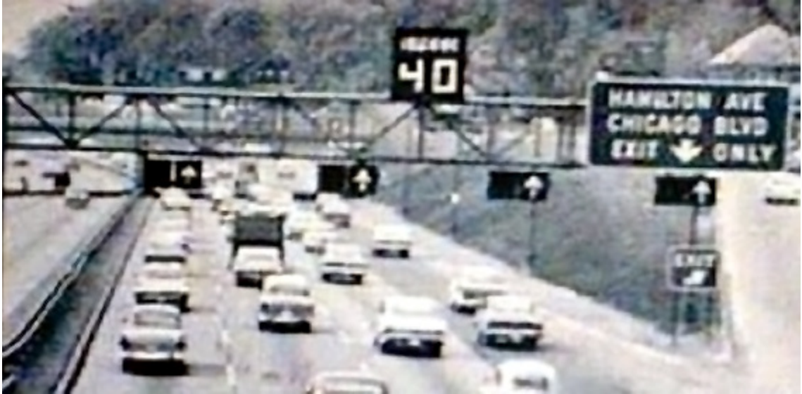
Figure 1.3: One of the earliest implementations of a VSL system in the United States occurred on The Lodge Freeway in Michigan during the 1960s [17].
