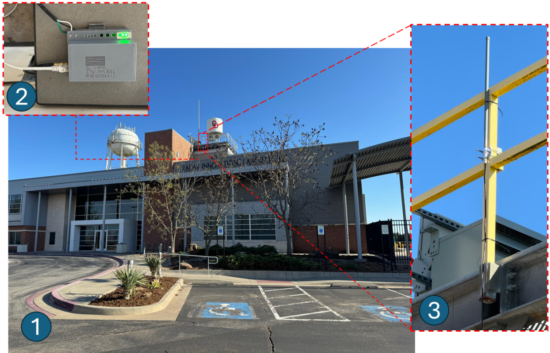
Figure 5.5: Installation of the BS for range tests: 1. The ARRC facilities were used to mount the BS. 2. The BS was placed on a table on the top floor where ethernet connections and power outlets were available. 3. The antenna was mounted on the terrace, with fiberglass handles serving as the mounting structure.
