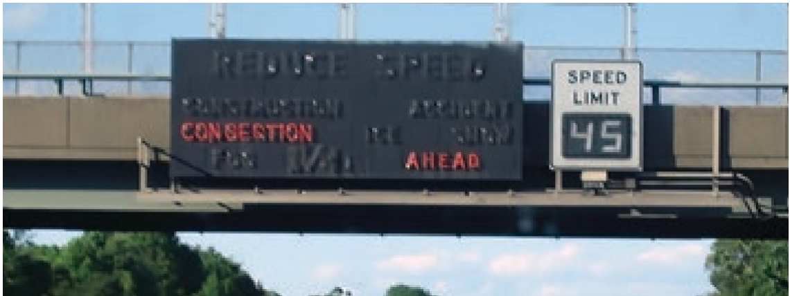
Figure 1.5: A VMS and a VSLS installed on the New Jersey Turnpike in the late 1960s [16]. The picture clearly shows the use of neon lights for the VMS and mechanical parts for the VSLS, which were two of the most common technologies of that time.
