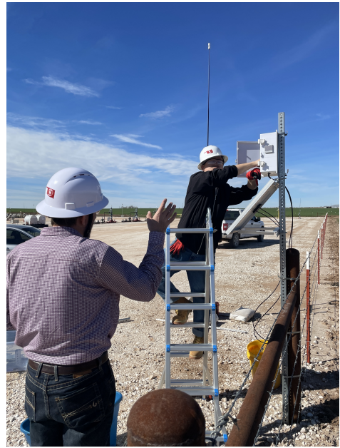
Fig. 4.1: A field installation of the NDIR sensor instrument
