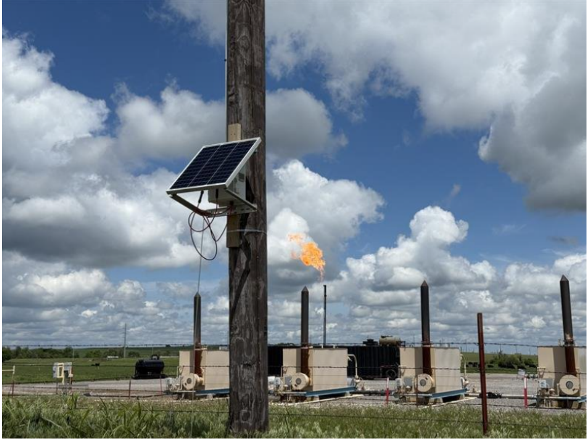
Fig. 5.1: Field Installation of Field Monitoring System
