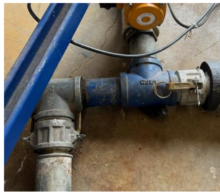
Figure 4.3. Fluid Mixing at Tee
