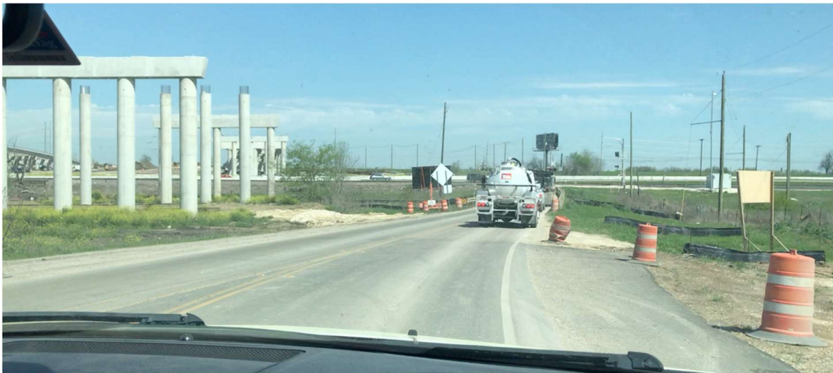
Figure 12. New traffic patterns in construction: This photo was taken at the intersection of a four-lane State Highway 79 and a farm-to-market road. Prior to Samsung and the construction of a rail depot directly to the right of the photo’s view, this was a backroads connection for farmers to travel N-S in between the two major E-W routes in the area. At one time, farmers and residents could turn right or left or drive straight at the intersection. Now, a cloverleaf fly over is being developed to accommodate truck traffic into the railyard and commuter traffic into Samsung (Maness, 2025a). Photo taken by author in March of 2024.
