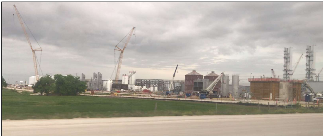
Figure 21. Samsung water reclamation facility under construction: This water treatment plant is just one part of the massive infrastructure that been added at the Samsung site. Photo taken by author.
