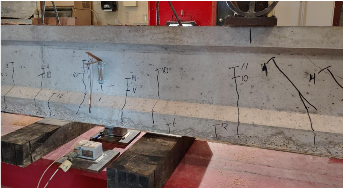
Figure A-16: Flexural cracking in RC-B1 W side near max load
