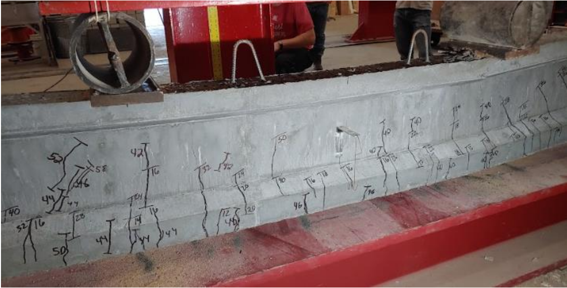
Figure A-31: Flexural cracking in UHPC-B3 E side
