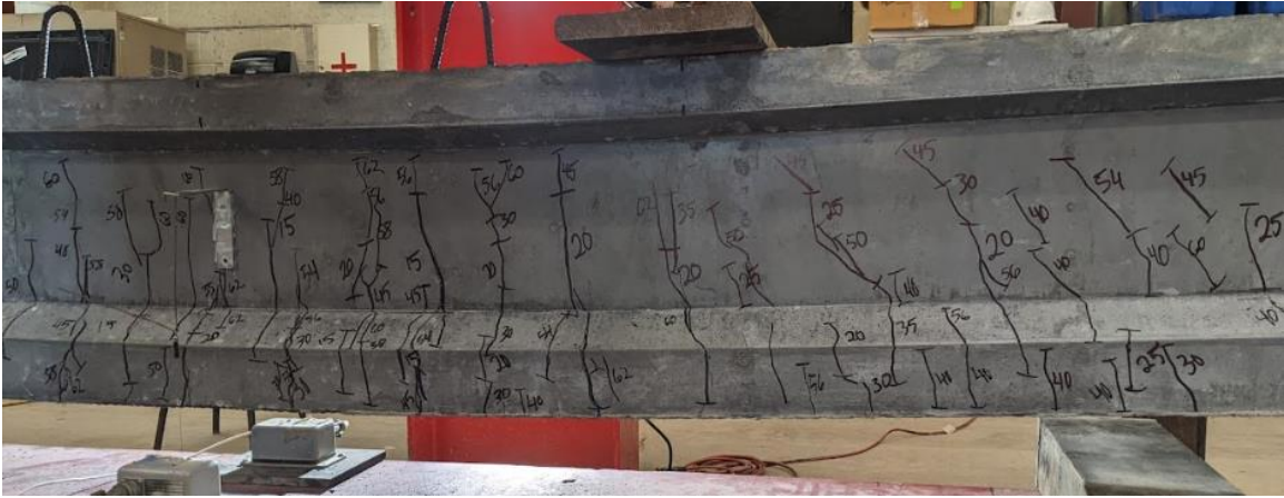
Figure A-49: Cracking in UHPC-B5 SW side
