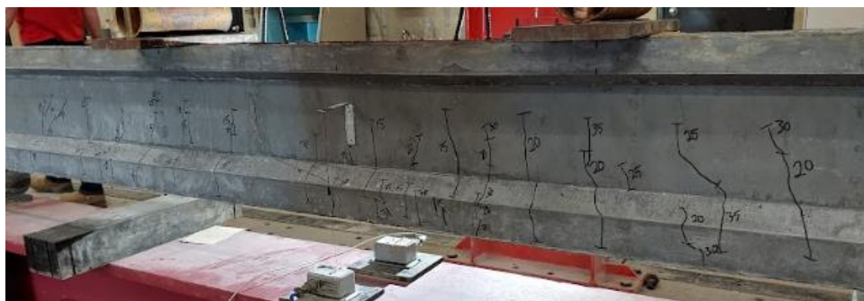
Figure 4-10: Flexural cracking of UHPC-B3 (a), UHPC-B4 (b), and UHPC-B5 (c)
