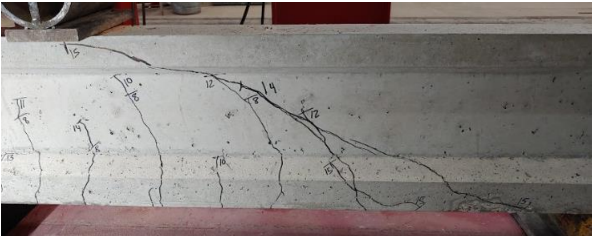
Figure A-22: Shear cracking in RC-B2 NE side
