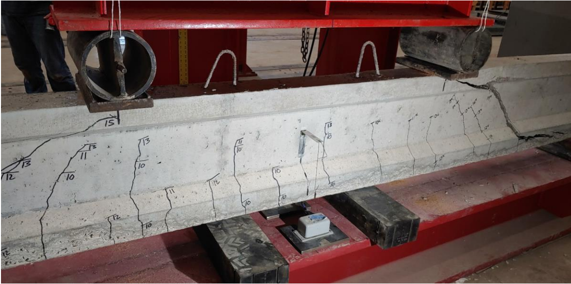
Figure A-17: Flexural cracking in RC-B1 E side after buckling
