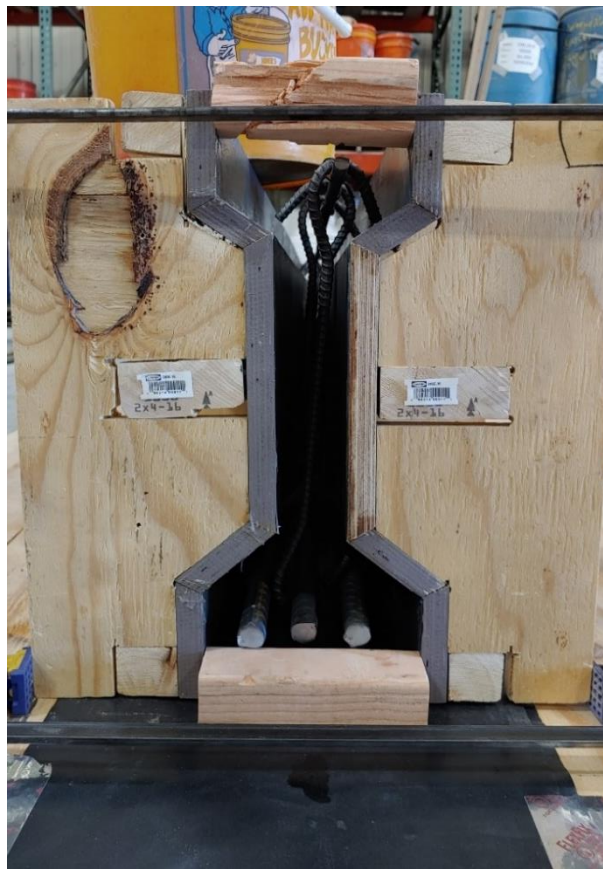
Figure 3-12: Cage between both walls of formwork
