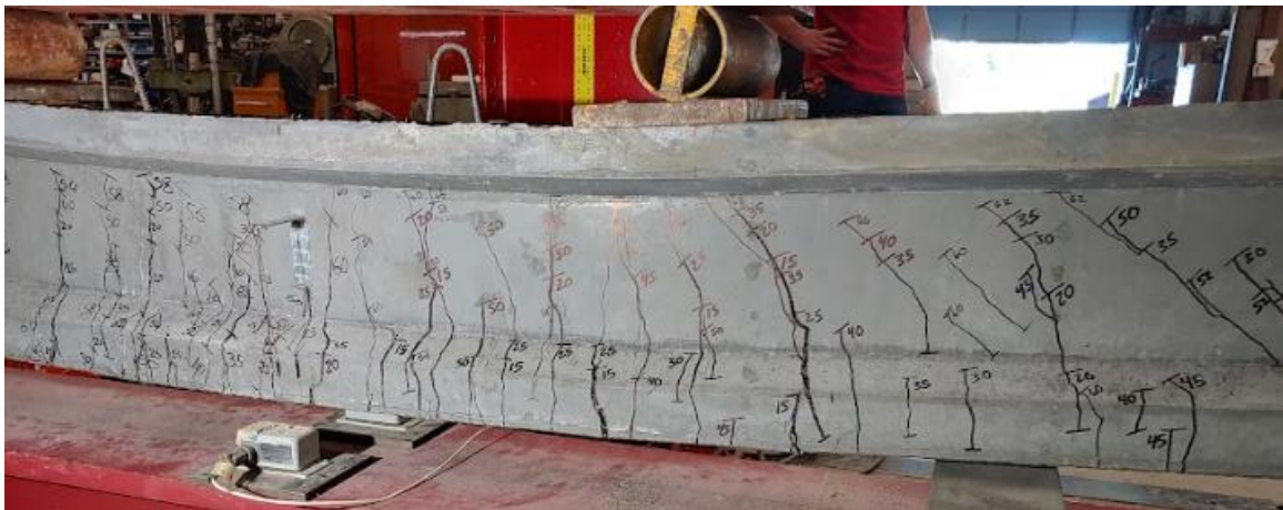
Figure A-46: Cracking in UHPC-B5 NE side
