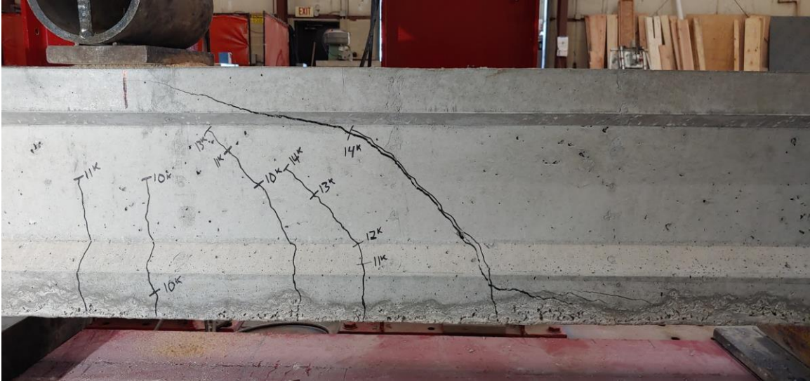
Figure A-13: Shear cracking in RC-B1 NE side
