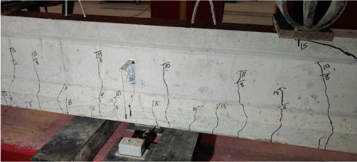
Figure A-25: Flexural cracking in RC-B2 E side
