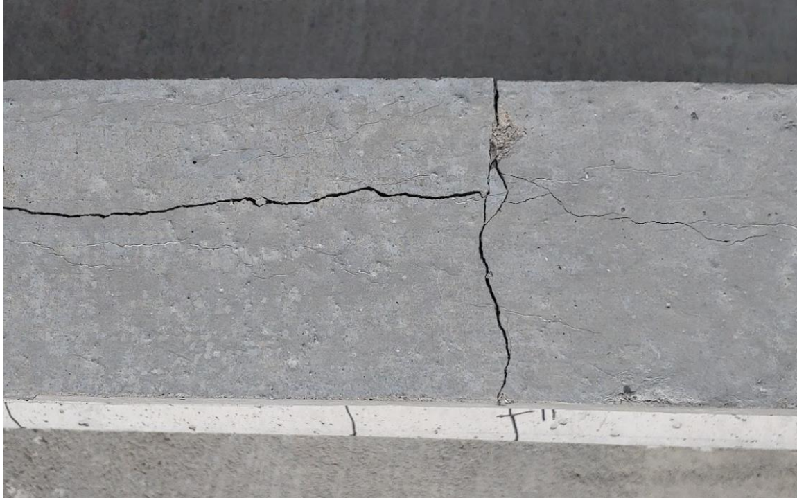
Figure A-19: Buckling of top flange in RC-B1 top view
