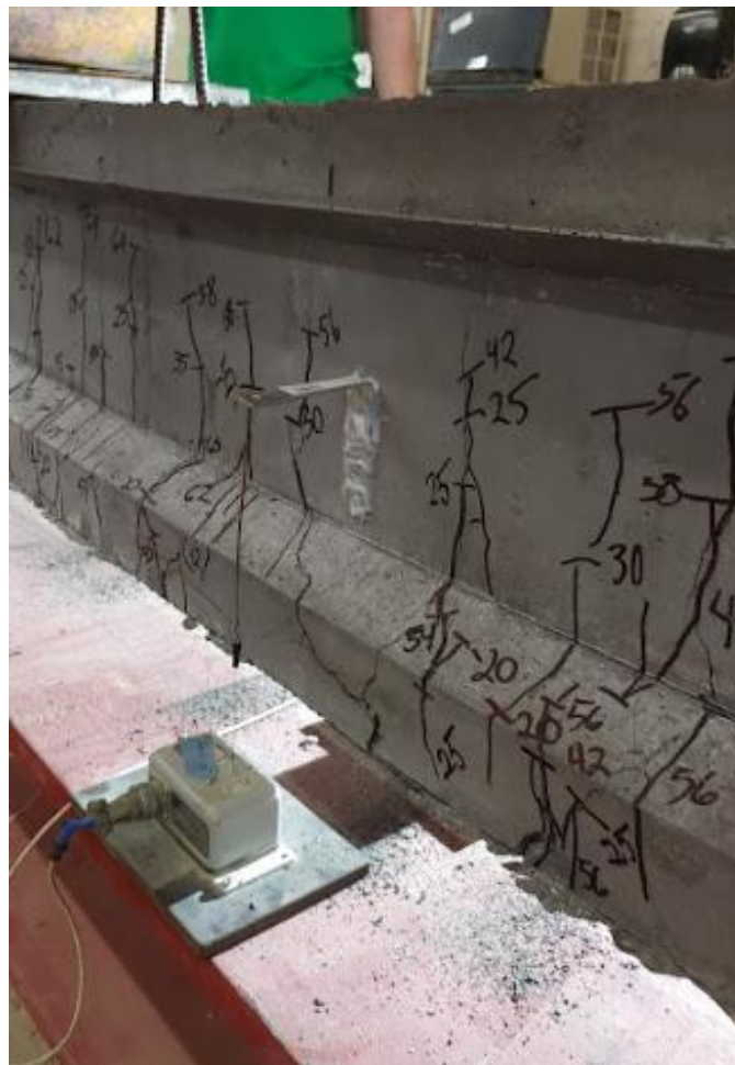
Figure A-42: Flexural cracking in UHPC-B4 W side
