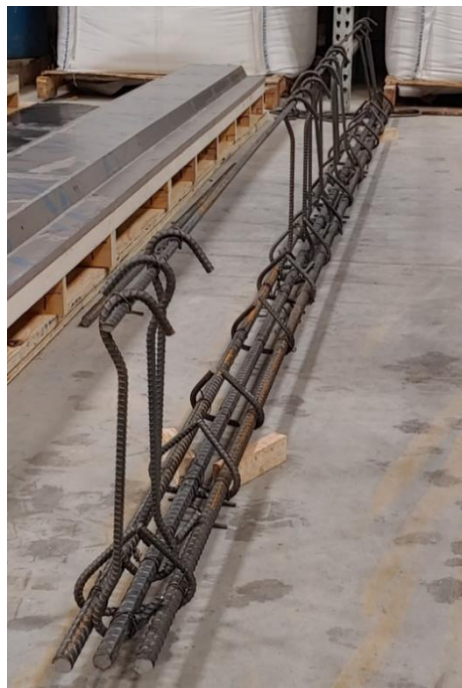
Figure 3-9: Completed reinforcing cage
