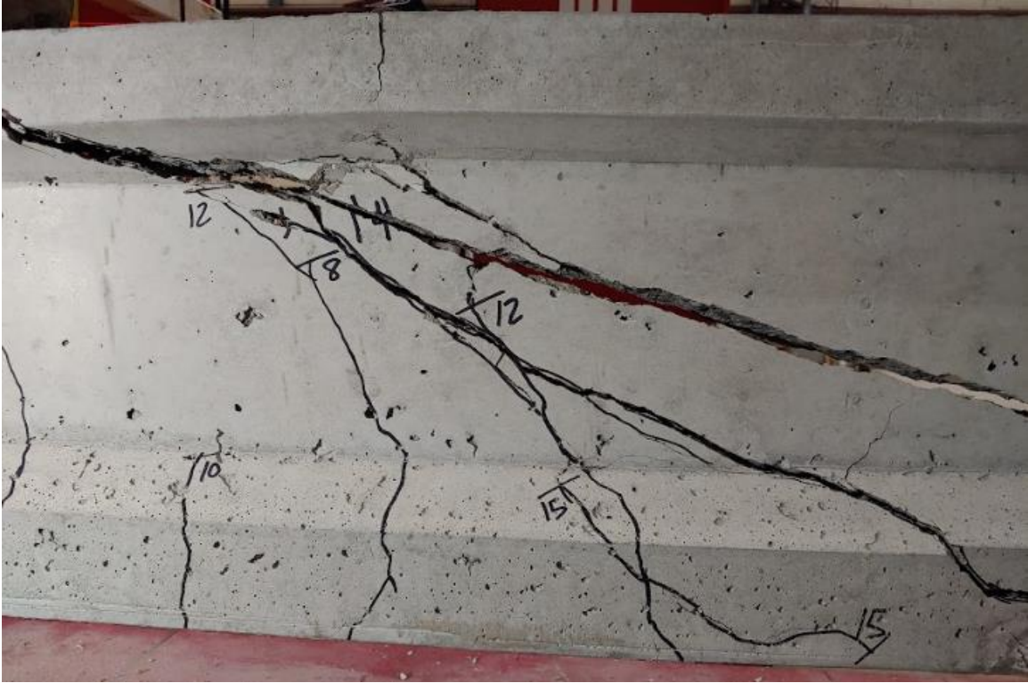
Figure A-23: Shear cracking in RC-B2 NE side after buckling
