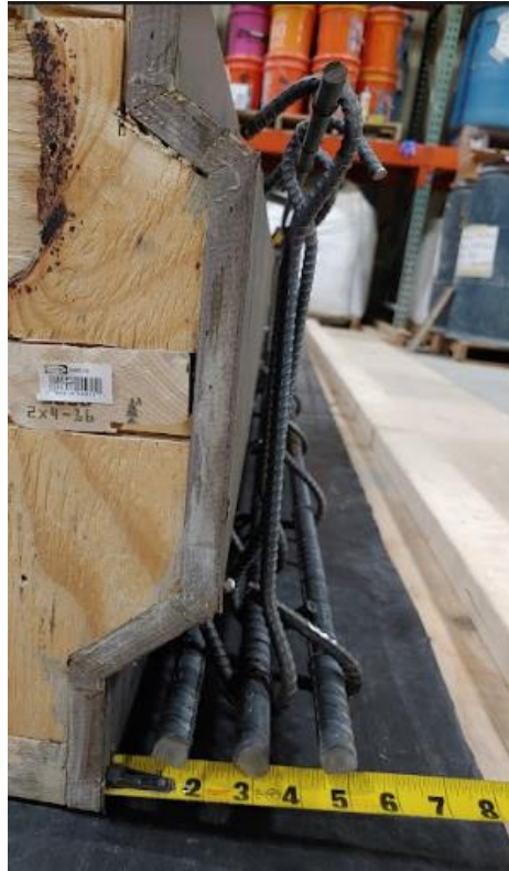
Figure 3-10: Horizontal placement of cage
