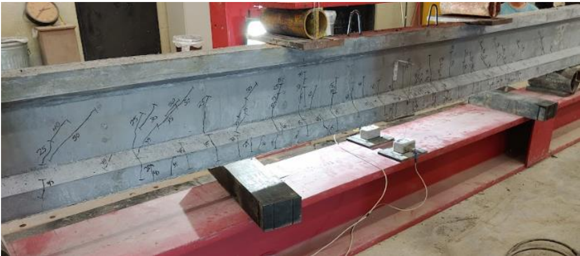
Figure A-48: Cracking in UHPC-B5 NW side
