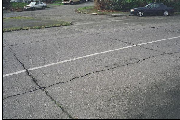
Figure 4: Reflective Cracking
