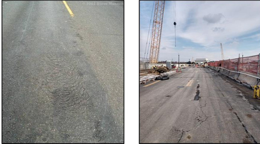
Figure 3: Slippage Failure [34]
