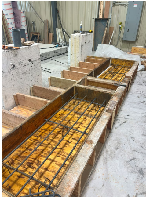
Figure 18: Reinforcement for Continuously Reinforced Specimens in Formwork
