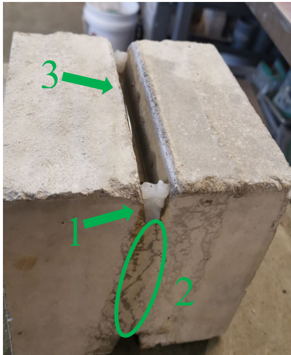
Figure 6: Product applied on flat crack
