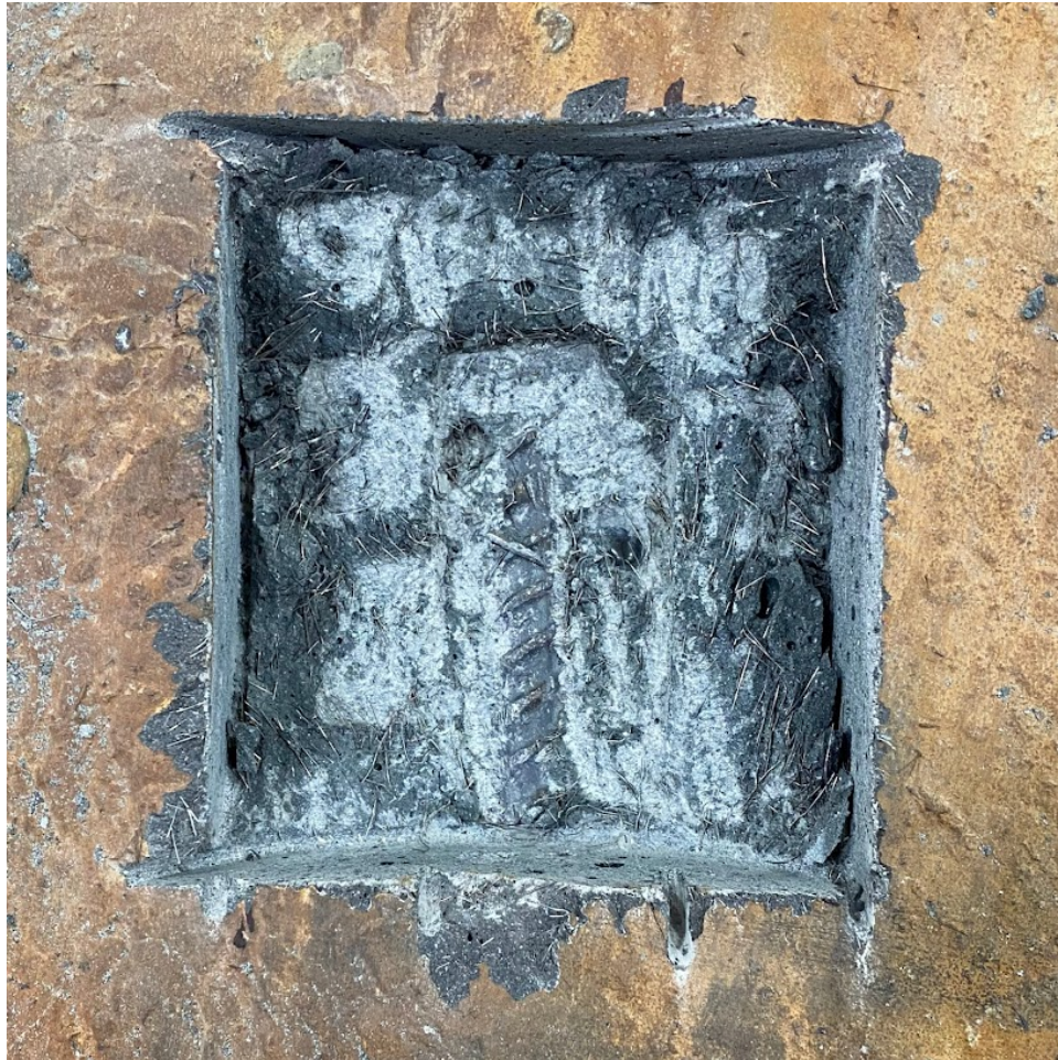
Figure 5-32: CU-N observed rebar C, 65 days tested
