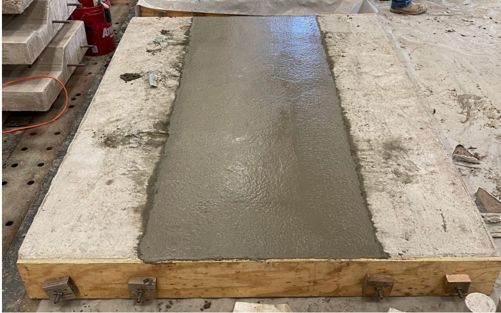
Figure 3-24: Class AA link slab after pouring, leveling
