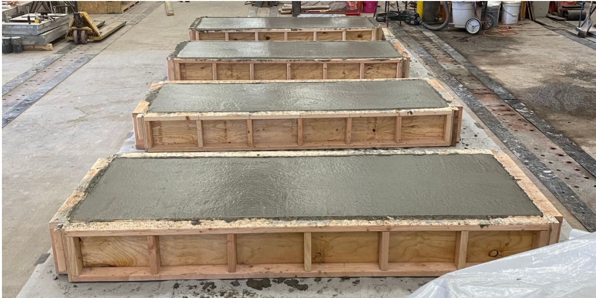
Figure 3-15: Set of slab sections after pouring, screeding
