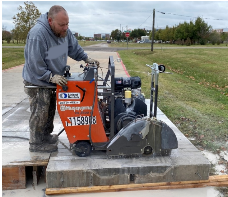
Figure 4-1: Cutting specimen sections from link slab
