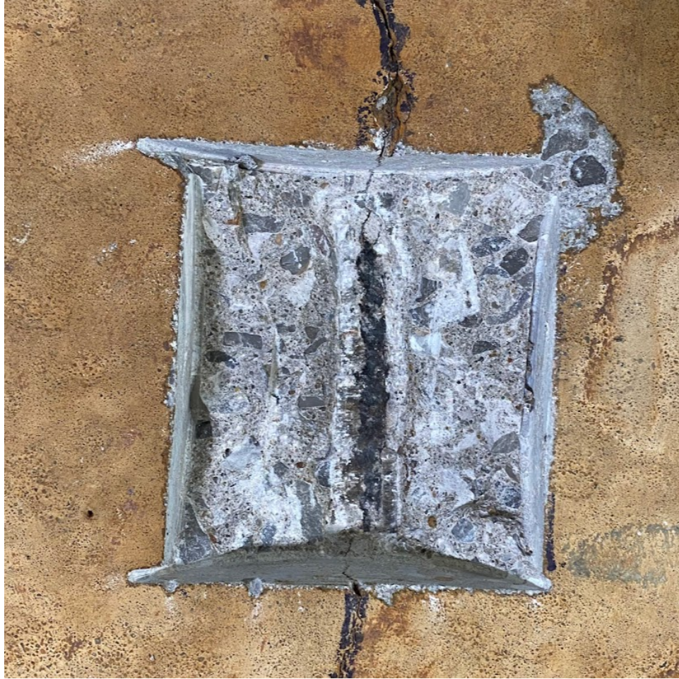
Figure 5-24: CAA-L observed rebar D, 65 days tested
