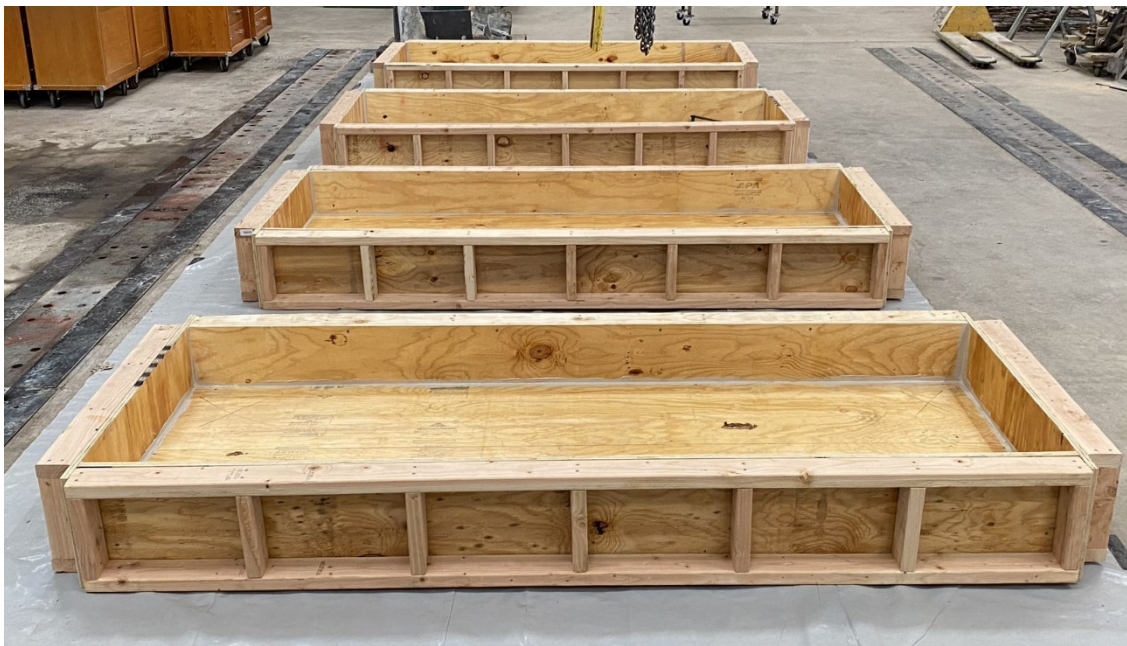
Figure 3-5: Formwork for four slabs
