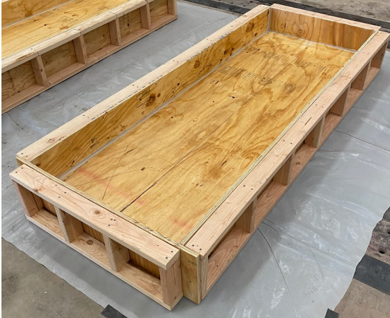
Figure 3-4: Formwork for one slab
