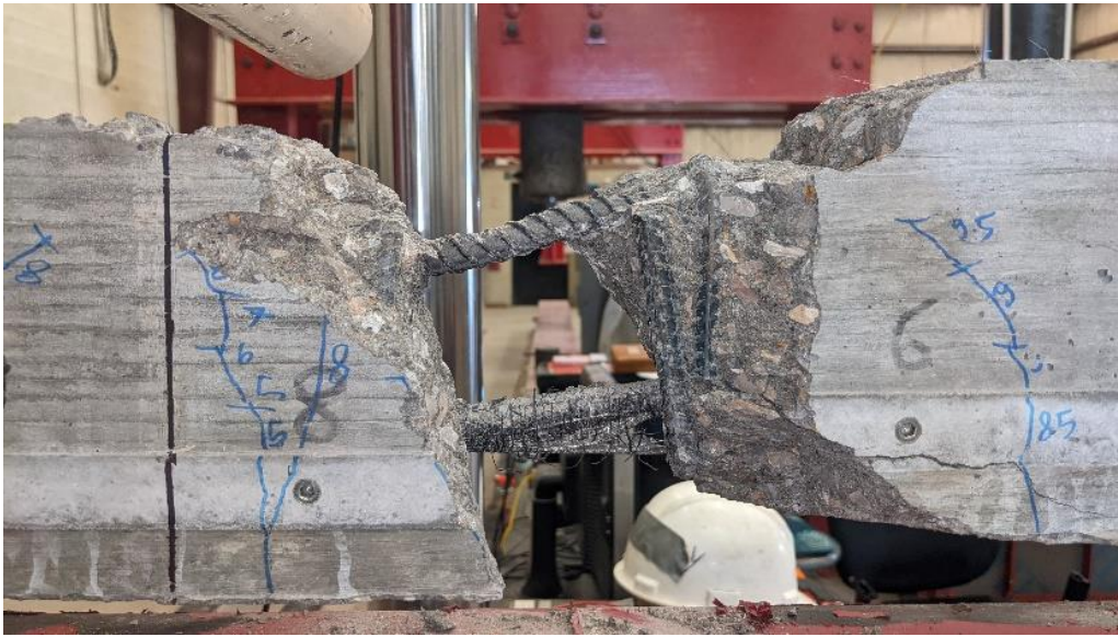
Figure 5-16: Photograph of the failed section of PB2
