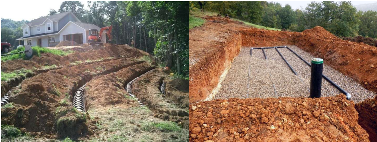
Fig. 5.1 (a) Trench drain field, [septic-tank-care.net] (b) excavated drain field, [CREDO]
