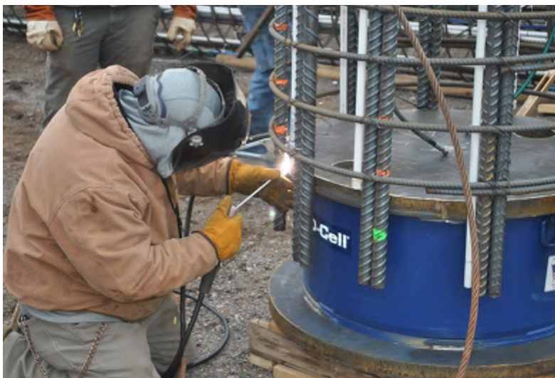
Figure 4.6 – Attachment of bi-directional loading device to bottom of shaft reinforcement.
