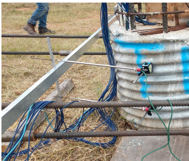
Figure 7.11 – Vibrating wire LVDTs attached to the reference beam.
