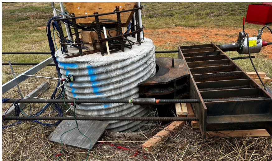
Figure 7.16 – Minco T1 in contact with isolation casing near the end of testing.
