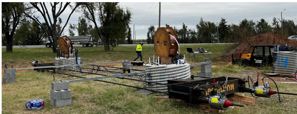
Figure 7.3 – One side of lateral load test frame in place at the Minco site.
