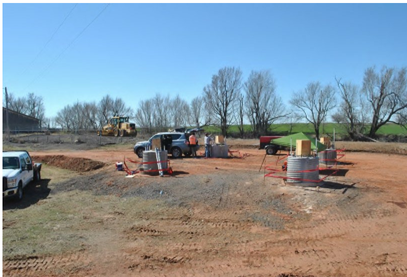
Figure 4.12 – Complete test shafts at the Minco site.
