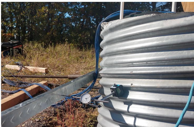
Figure 7.12 – Dial gage mounted to the CMP casing and connected to the reference beam.
