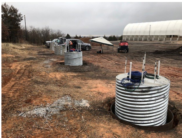
Figure 4.7 – Complete test shafts at the Edmond site.
