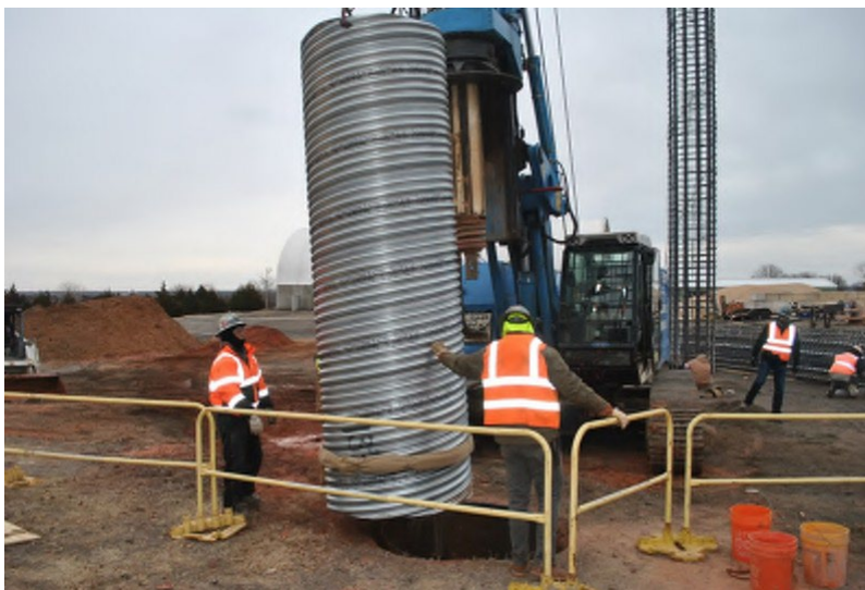
Figure 4.5 – CMP inner casing with burlap packing placed around tip.
