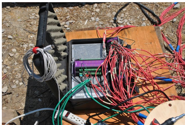
Figure 7.7 – DataTaker data acquisition system with vibrating wire strain gages and LVDTs connected to the multiplexer.
