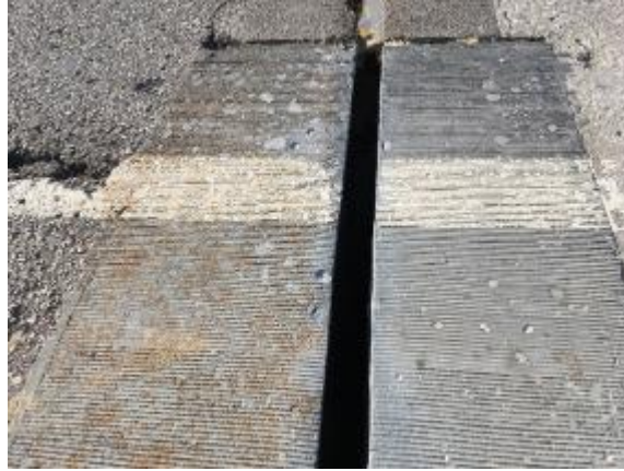
Figure 338. UHPC joint headers on SH-3E bridge before joint sealant was placed and showing surface rusting of the exposed steel fibers
