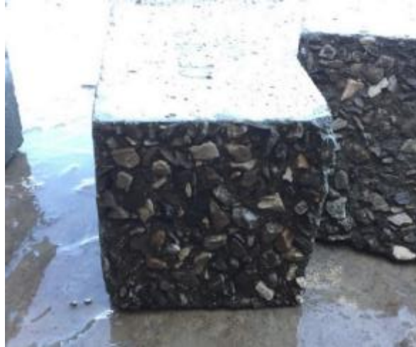
Figure 53. Exposed aggregate surface after power washing
