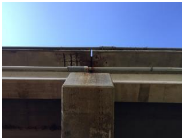
Figure 327. Underside of the SH-3 bridge over N. Canadian River at the candidate joint showing concrete deterioration
