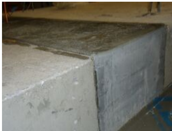
Figure 86. Completed Ductal® slab joint after formwork removal
