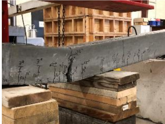
Figure 77. Crack pattern typical of SB-J5 with 2% fibers
