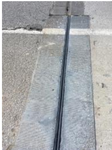
Figure 336. UHPC joint headers on SH-3E bridge immediately after joint sealant was placed
