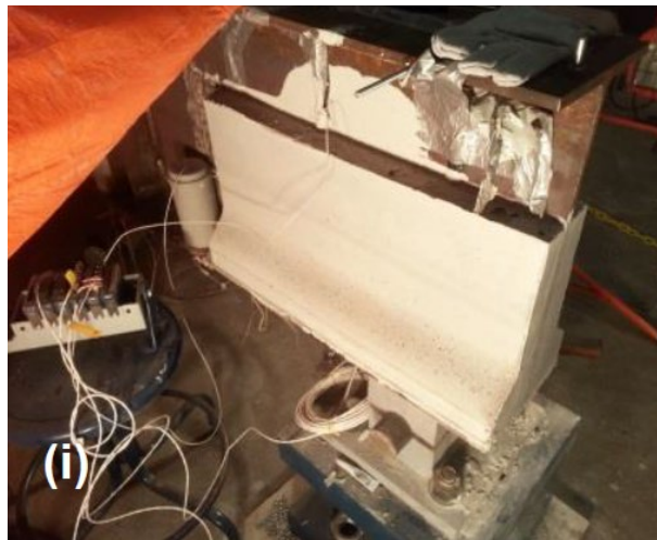
Figure 12. Final repaired girder (Zmetra 2015)
