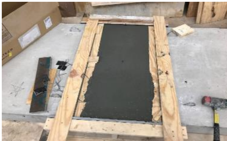
Figure 101. Self-consolidating UHPC filling the joints
