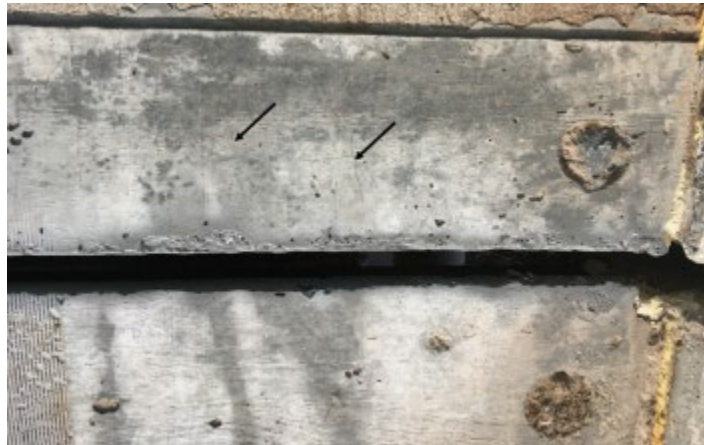
Figure 337. UHPC joint headers on SH-3E bridge before joint sealant was placed and showing hairline cracks
