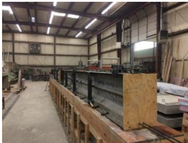
Figure 173. Prestressed beam formwork immediately before casting
