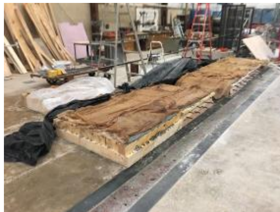
Figure 81. Conventional concrete slabs curing under wet burlap
