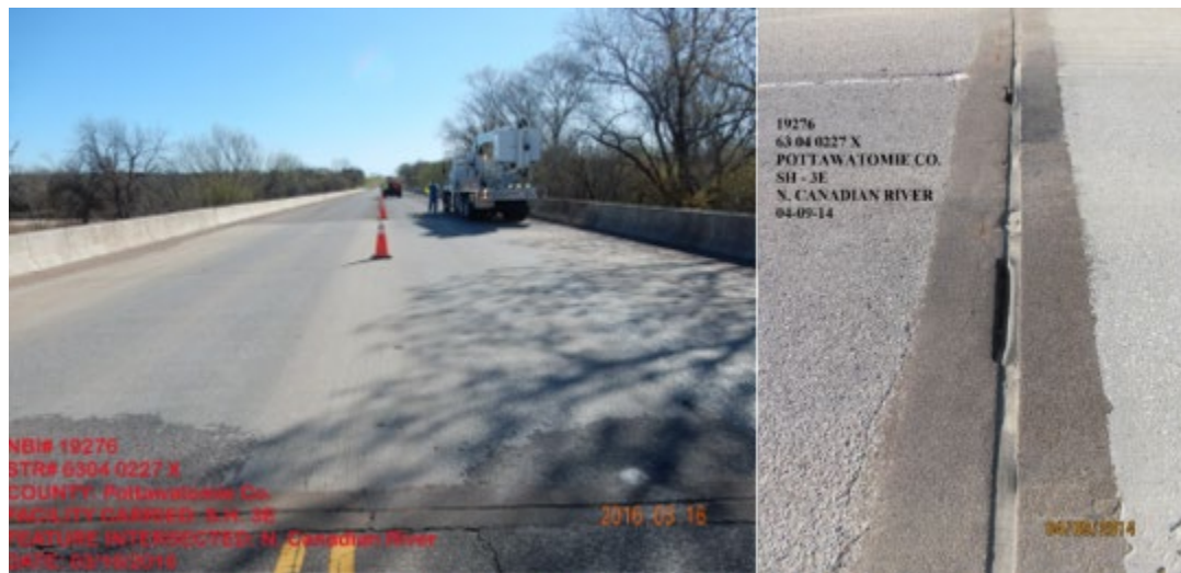
Figure 326. SH-3 bridge over N. Canadian River (left) and expansion joint to be replaced (right)
