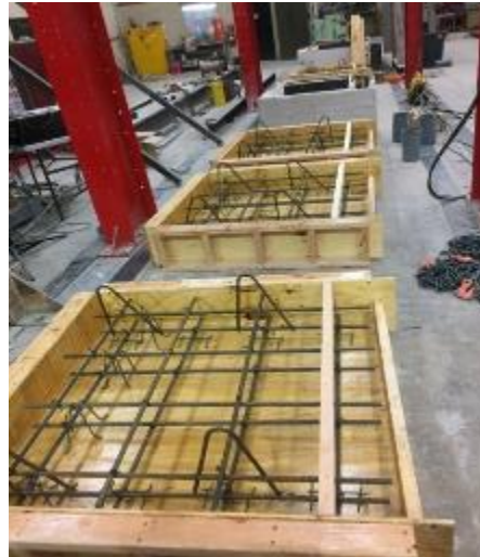
Figure 89. Formwork prepared for concrete casting
