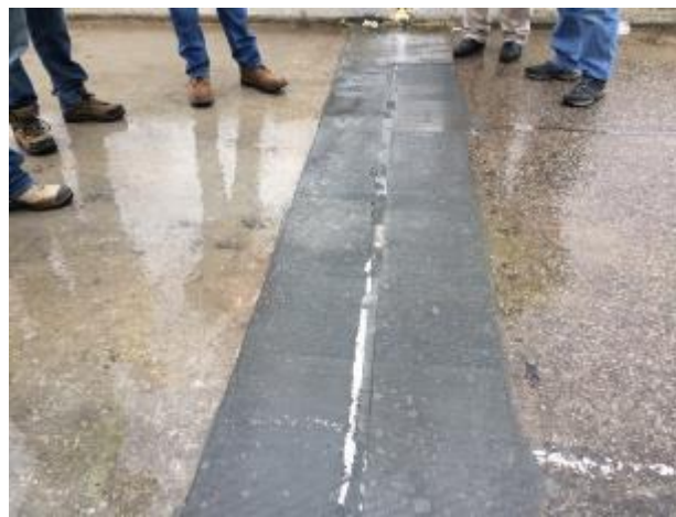
Figure 333. Entire joint after grinding
