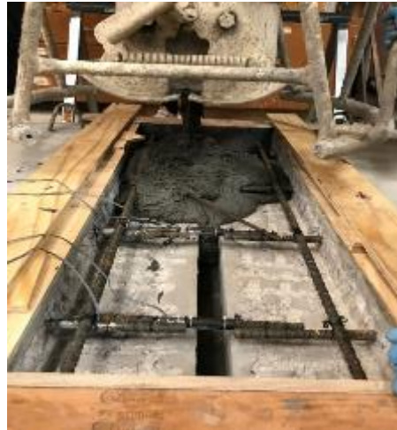
Figure 100. Placement of UHPC connecting two slab panels
