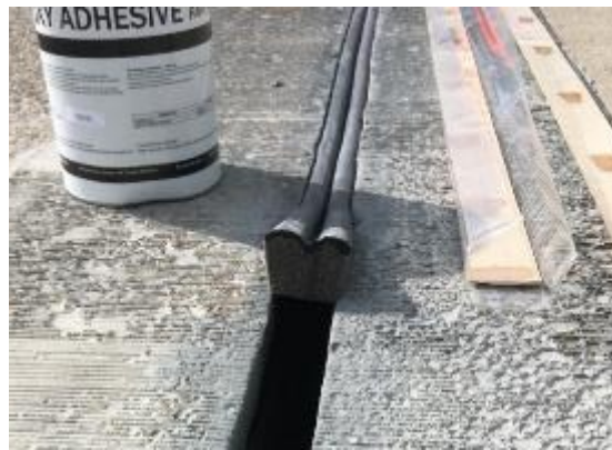
Figure 335. End of joint sealant prepared for splicing
