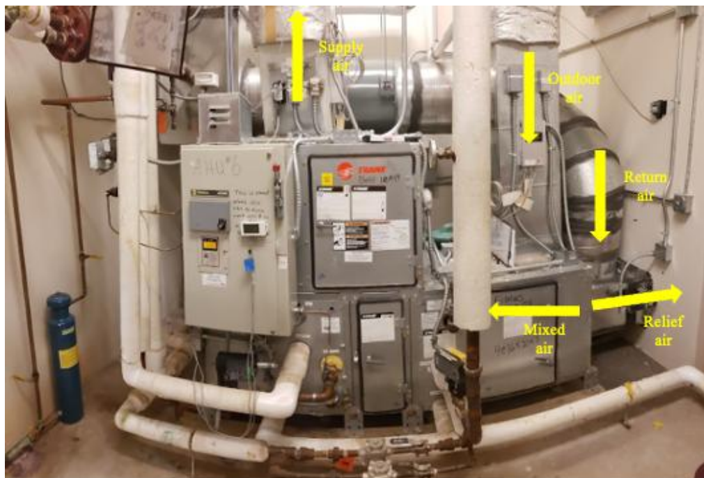
Figure 3.4: Single-duct VAV AHU system
