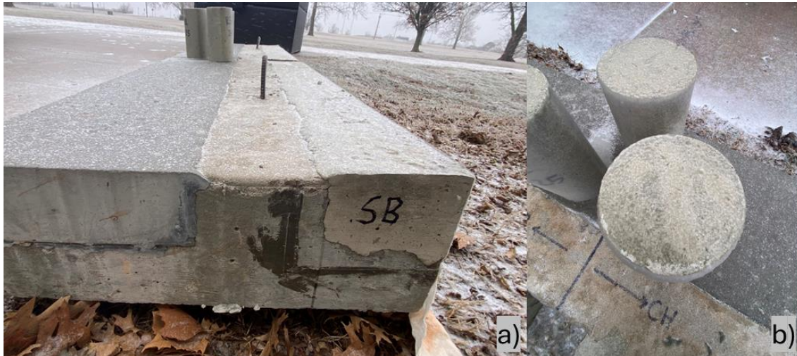
Figure 40: RS-SCC Large-Scale Repair Slab (a) and Compressive Strength Cylinders (b) with Ice Accumulation
