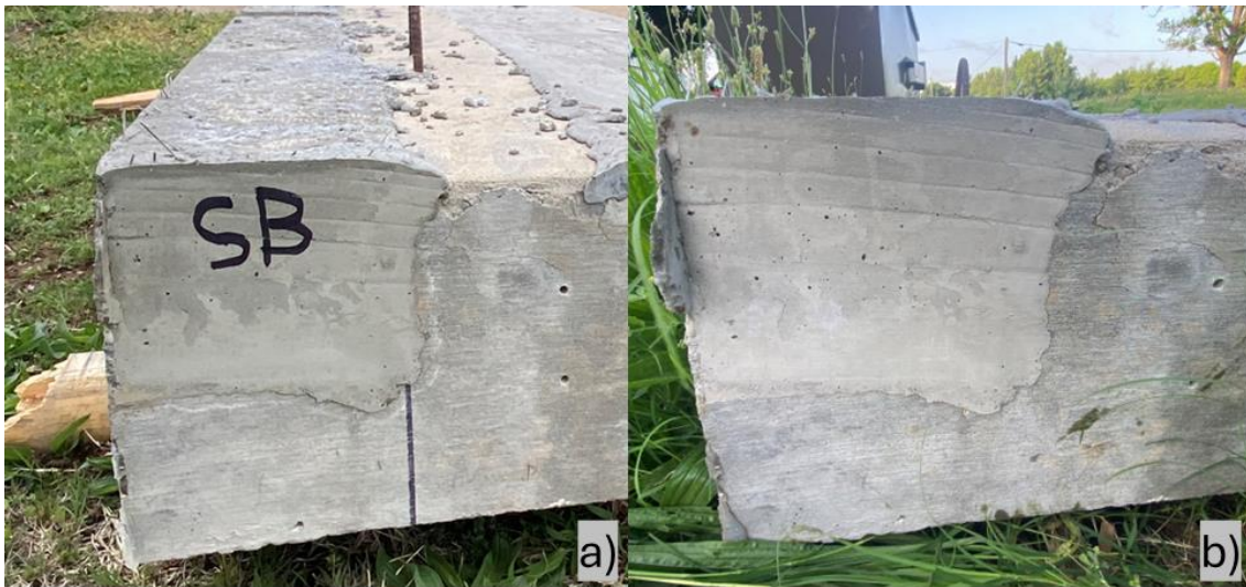
Figure 43: Comparison of FR-SCC Repair Material Before (a) and After (b) Exposure
