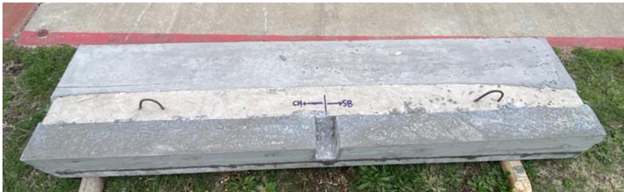
Figure 42: Large-Scale FR-SCC Repair Slab Before Exposure
