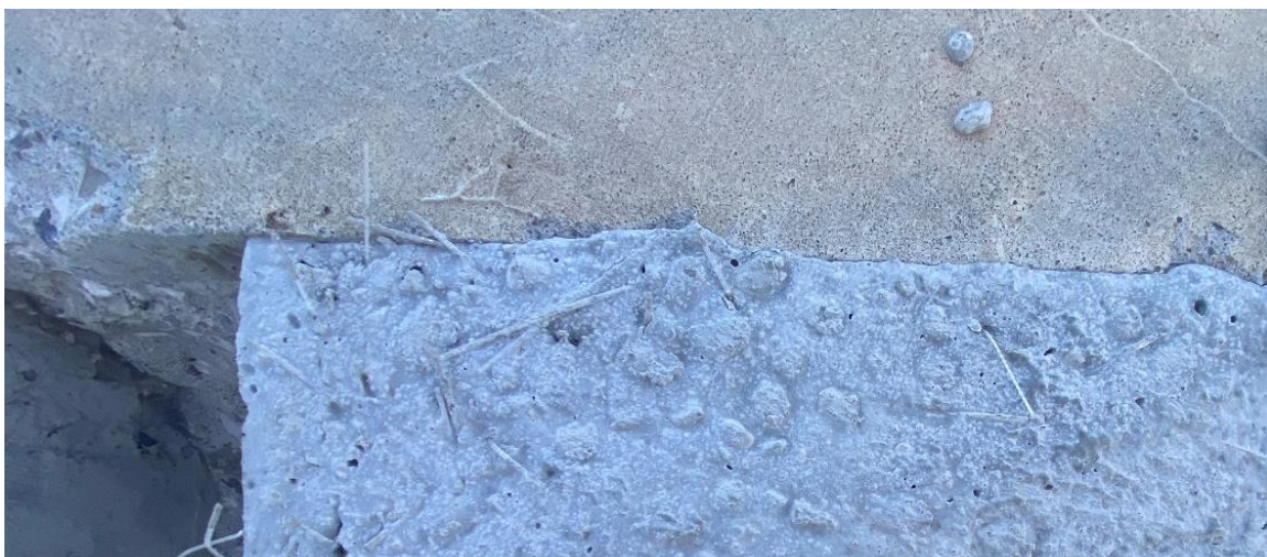
Figure 44: Interface Zone of FR-SCC Repair Slab
