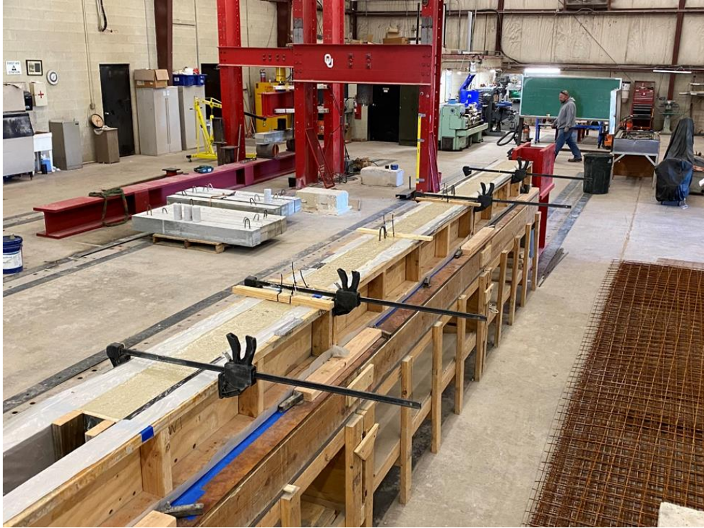
Figure 96: Trial beam B2 immediately after casting
