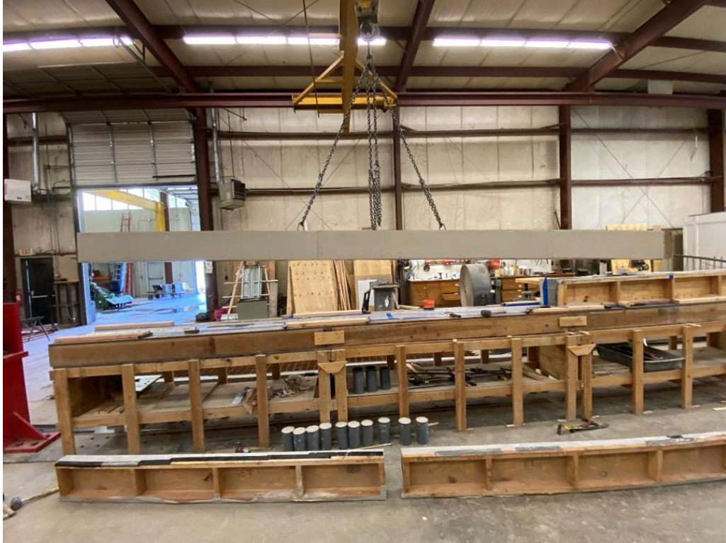
Figure 97: Trial beam B2 being removed from the prestressing bed after forms are stripped and prestress released at 3.5 hours of age
