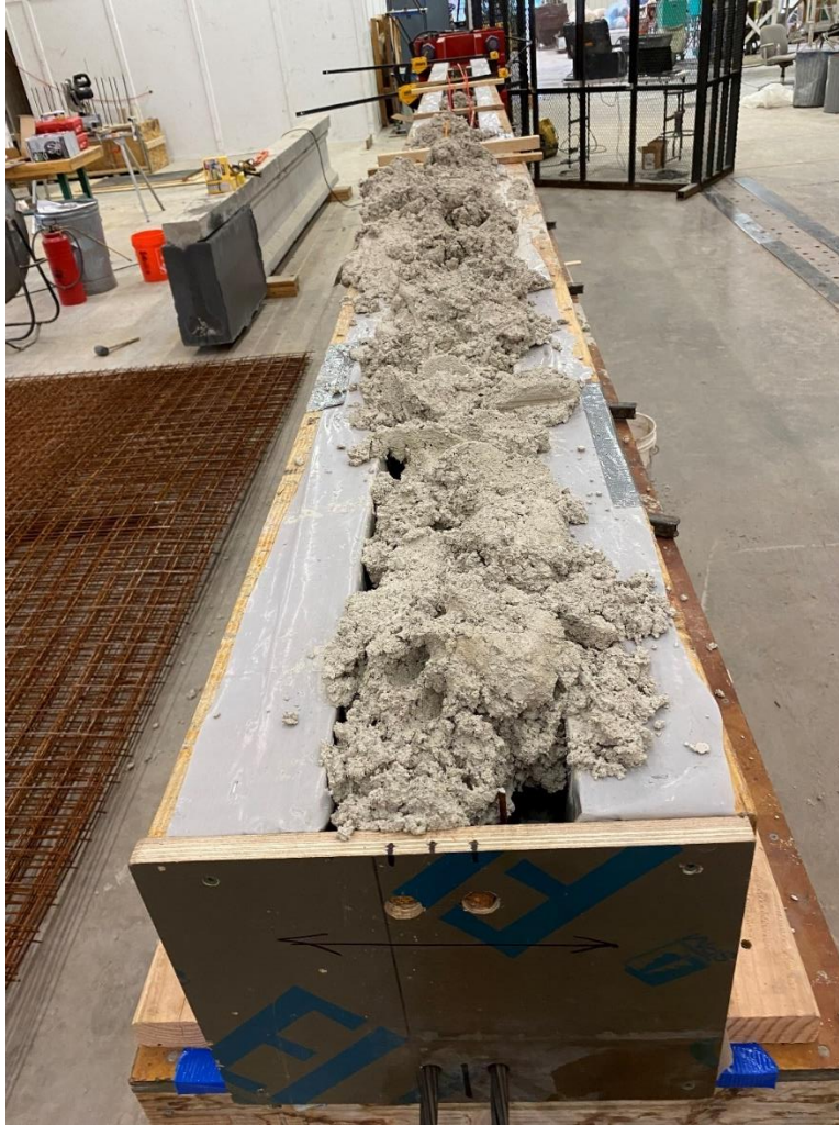
Figure 88: Trial beam B1 in the formwork after casting
