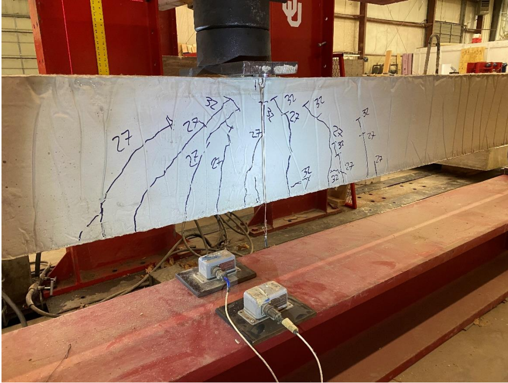
Figure 110: Cracking pattern at failure for B6-3DV with 4 ft embedment (live end)
