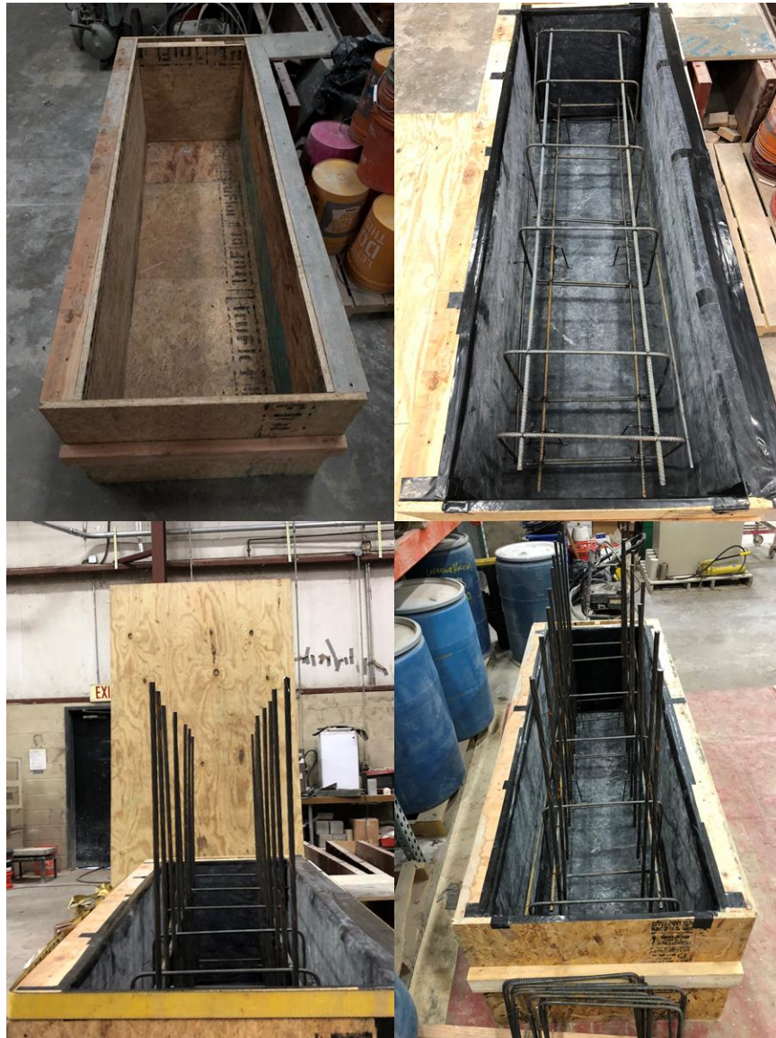
Figure 63: Full-scale LBPT specimen formwork, reinforcing bar cage, and tied strands (clockwise from top left)
