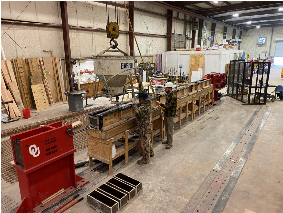
Figure 84: Filling beam formwork with concrete using a hopper and overhead crane
