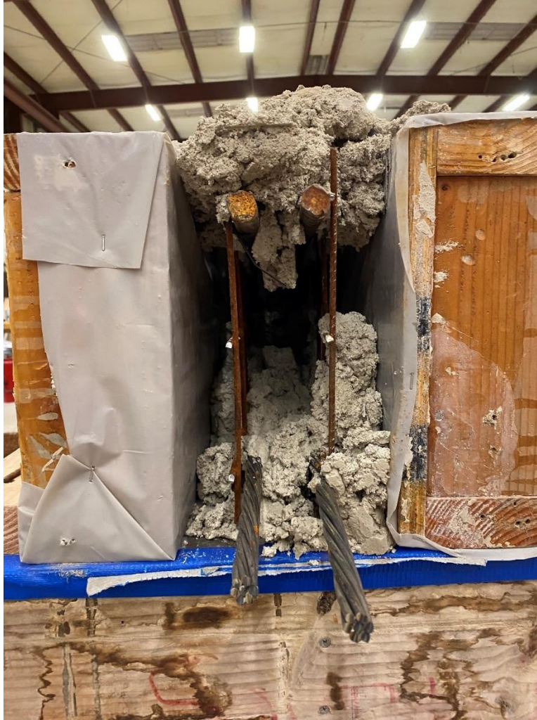
Figure 89: View of trial beam B1 from the end after prestress release and cutting of the strands
