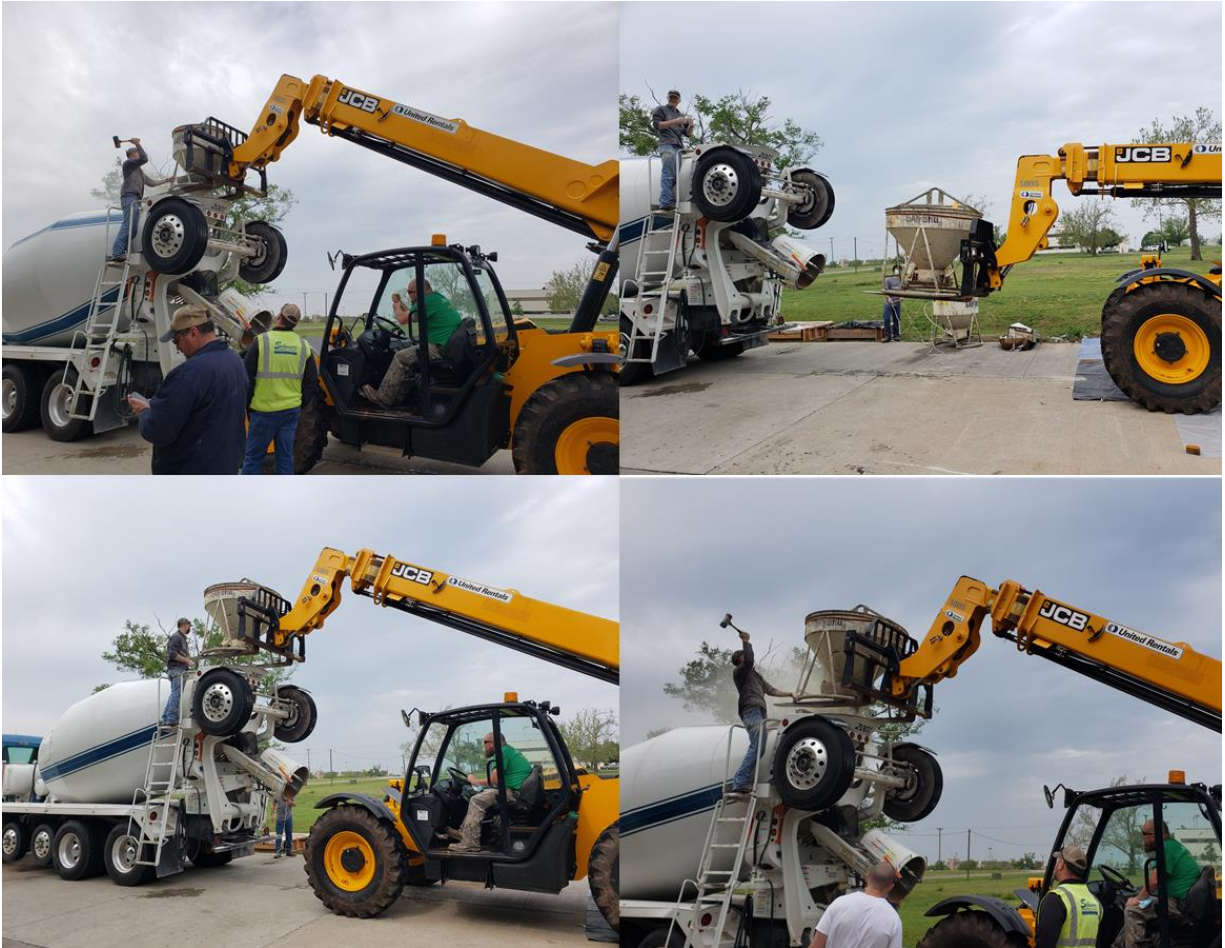
Figure 67: Charging concrete truck with BCSA cement at Fears lab using construction forklift and two separate hoppers
