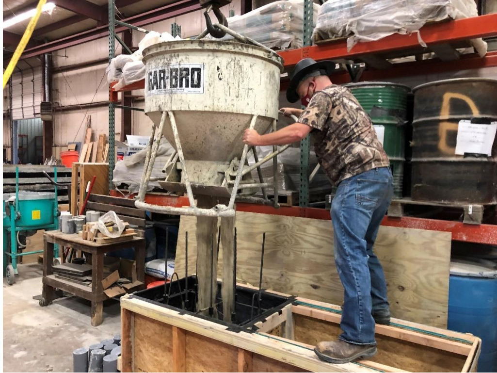
Figure 59: Placing RS-SCC with hopper and overhead crane
