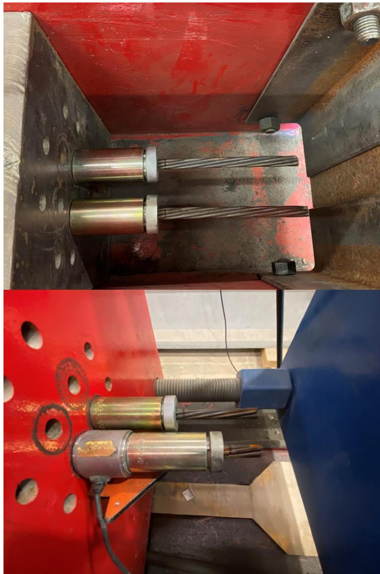
Figure 85: Strands chucked behind static bearing plate on dead end abutment (top) and strands chucked behind tensioning bulkhead on live end abutment with load cell (bottom)
