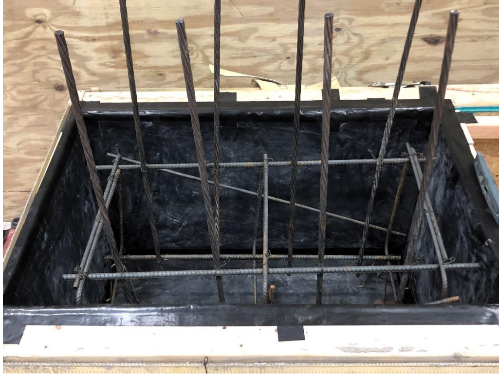
Figure 57: Strands tied in place for half-scale trial LBPT specimen
