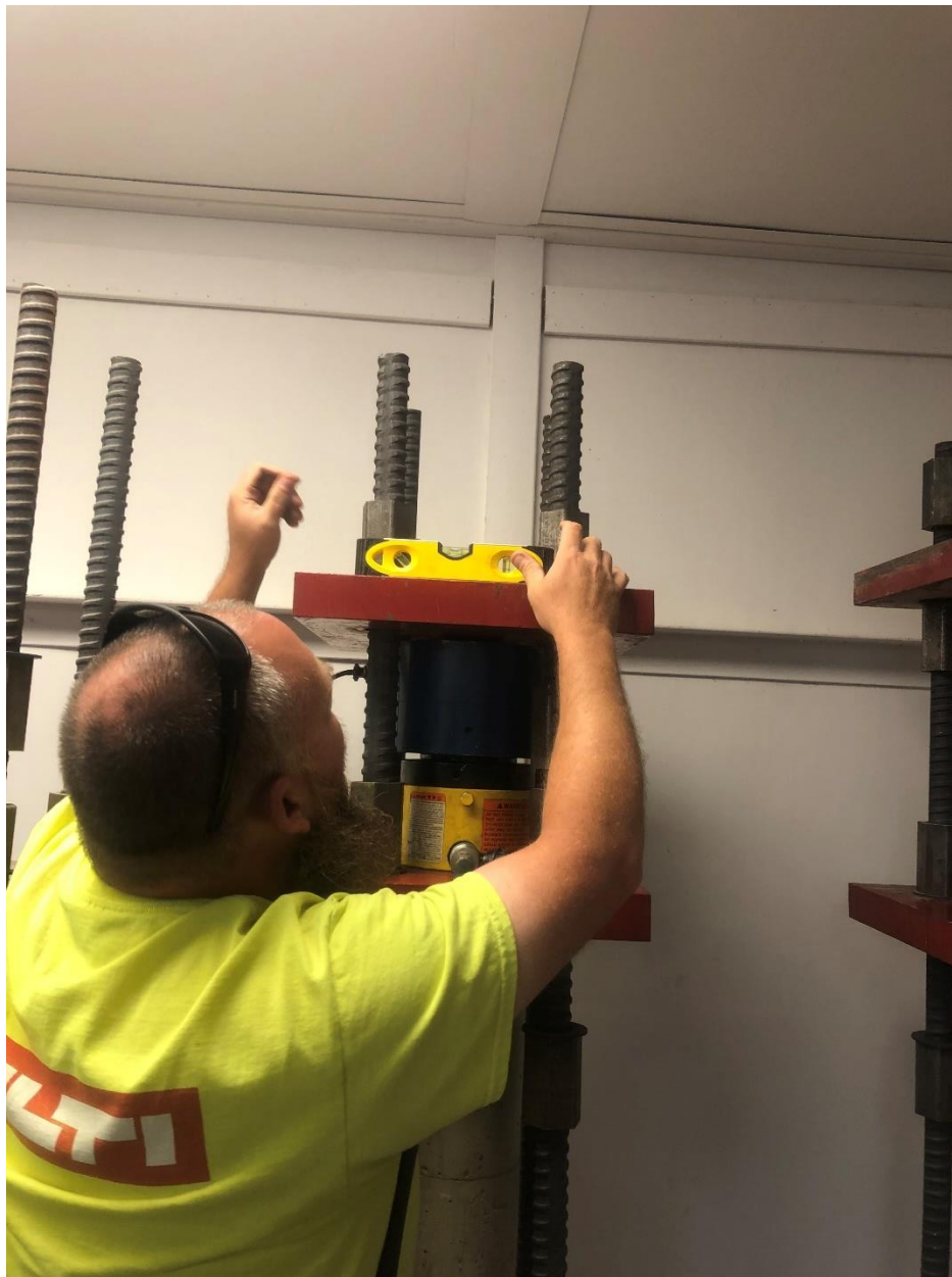
Figure 43: Levelling reaction plates to load creep frames
