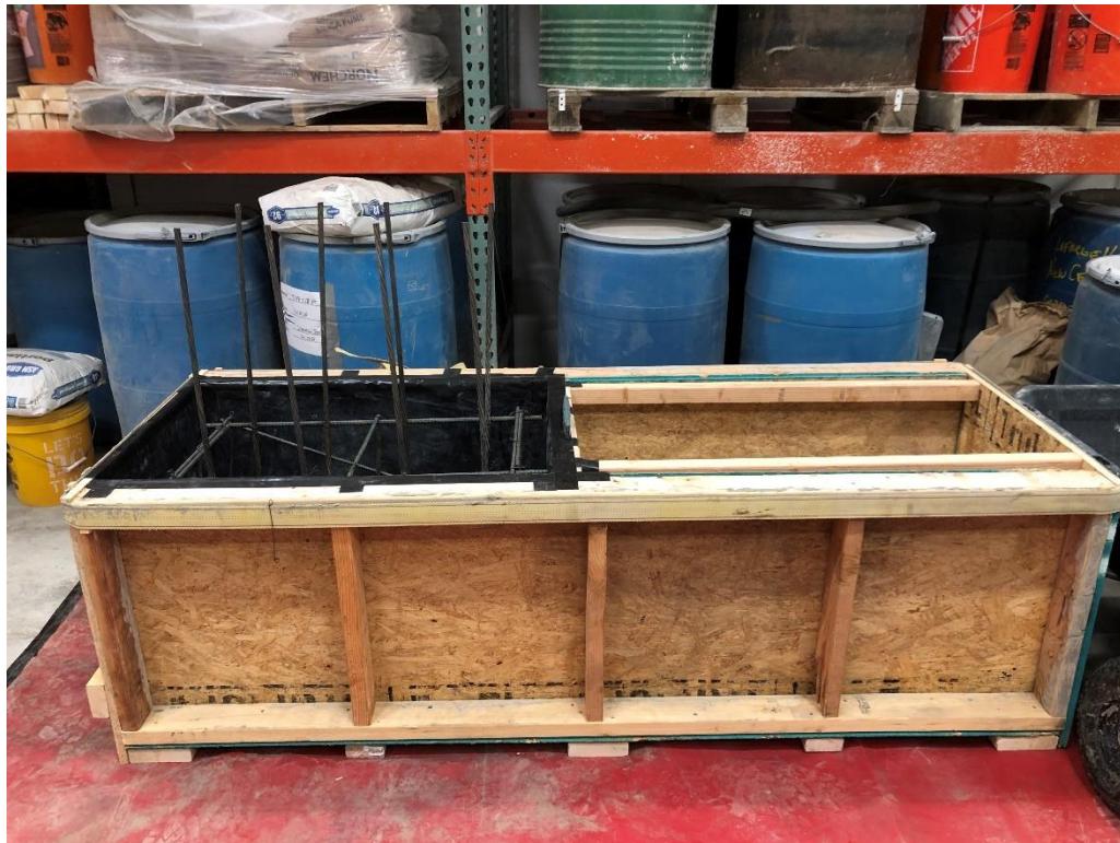
Figure 56: Formwork for half-scale trial LBPT specimen
