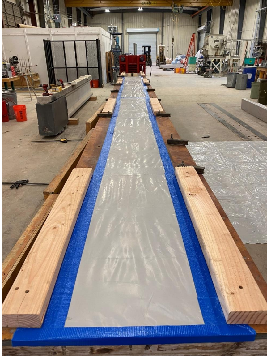
Figure 80: Prestressing bed prepared for form panel placement, looking toward live end abutment
