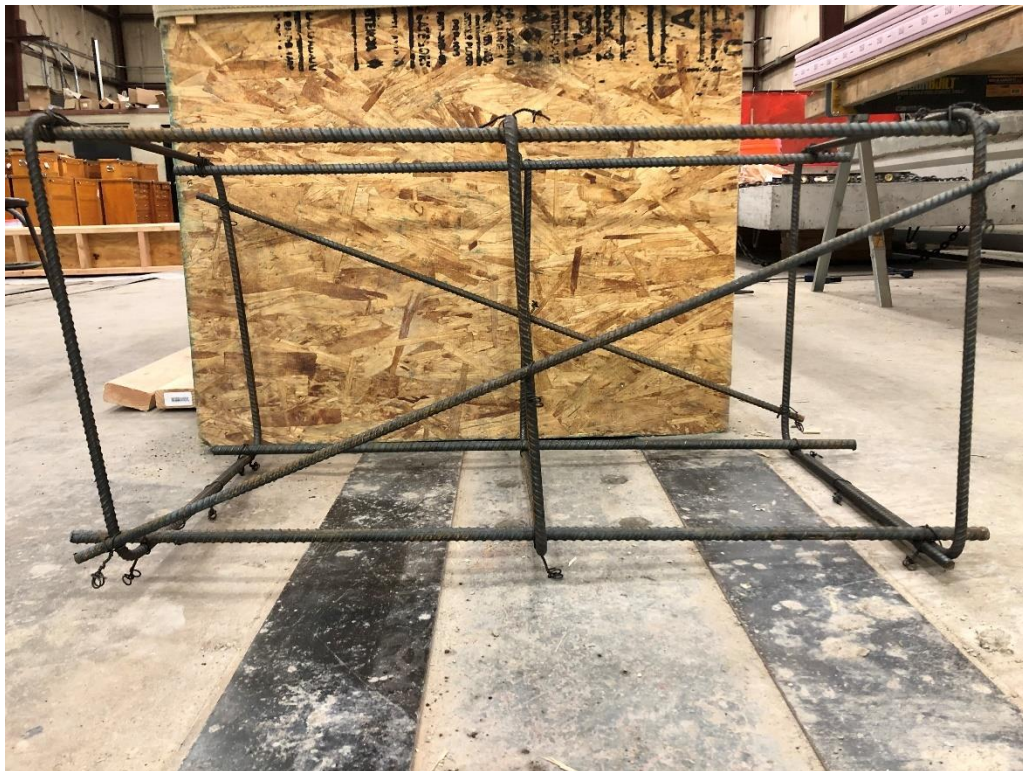
Figure 55: Reinforcement cage for half-scale trial LBPT specimen
