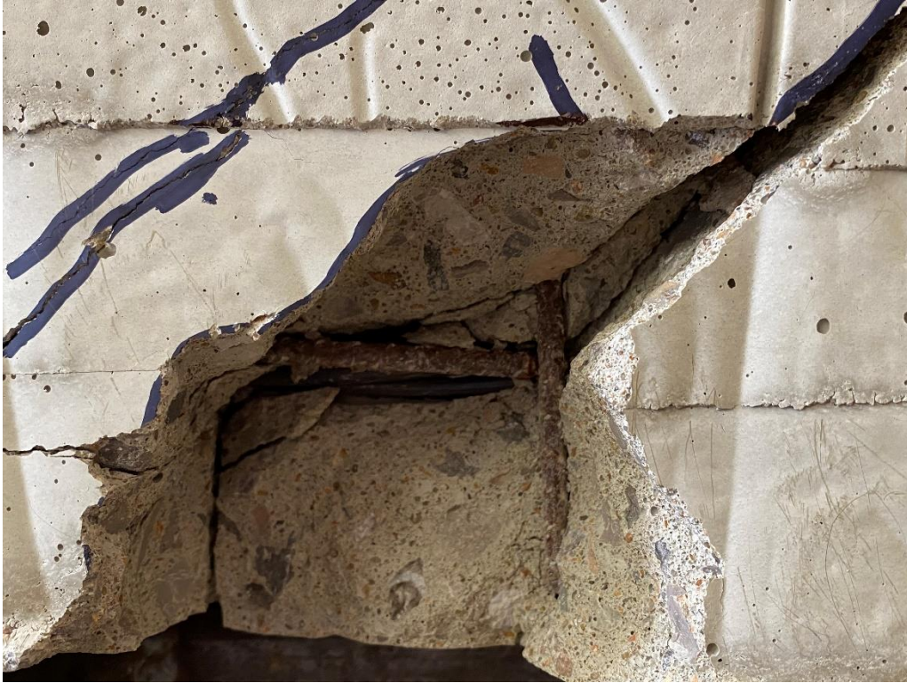
Figure 134: WWR damage from shear failure on test B13-24DV
