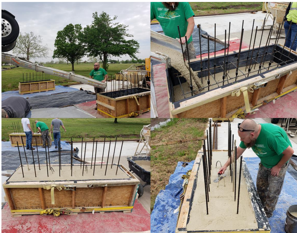
Figure 70: Positioning the mixer truck chute, filling the formwork, finishing the LBPT specimen surface, and a finished specimen (clockwise from top left)
