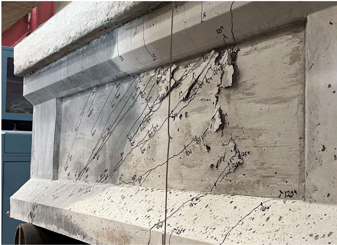
Figure 4.17: Failure of BiFluid hybrid girder no. 3
