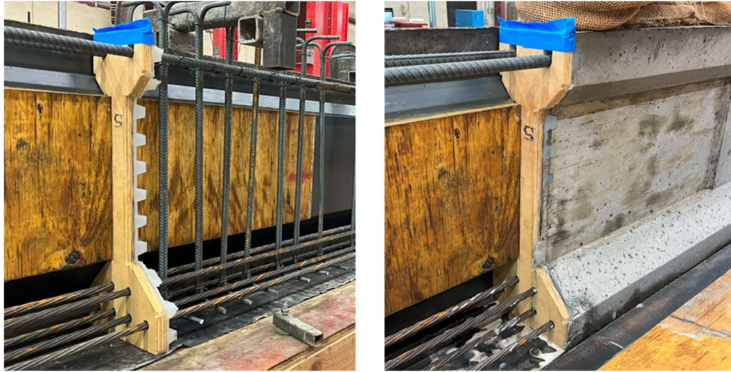
Figure 4.10: Interface texture placement with plywood backerboard before and after casting SCC section of the first 2D Trapezoidal hybrid girder
