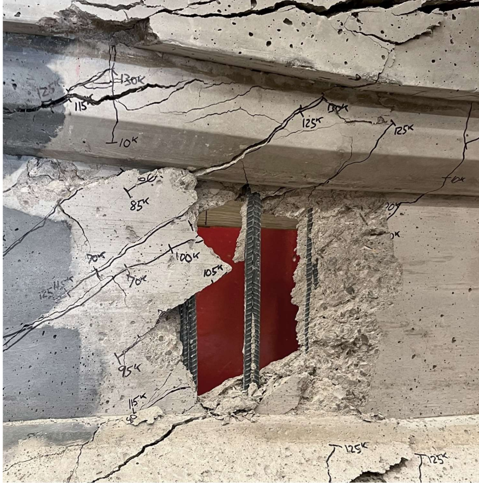
Figure 6.3: BiFluid Girder No. 1 failure after additional displacement featuring a vertical, “V-shaped” failure along the vertical reinforcing in the web.
