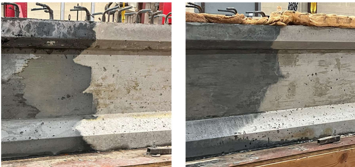
Figure 4.8: Interface alignment of BiFluid girder no. 1 (left) and BiFluid girder no. 3 (right)
