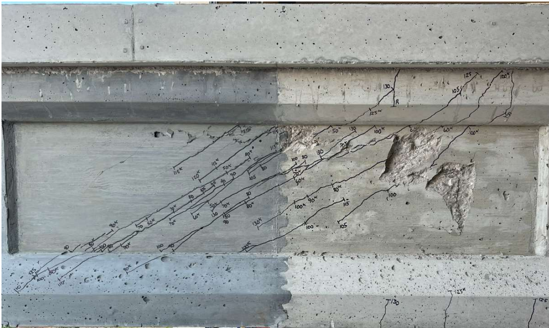
Figure 4.30: Failure of 3D textured hybrid girder no. 2
