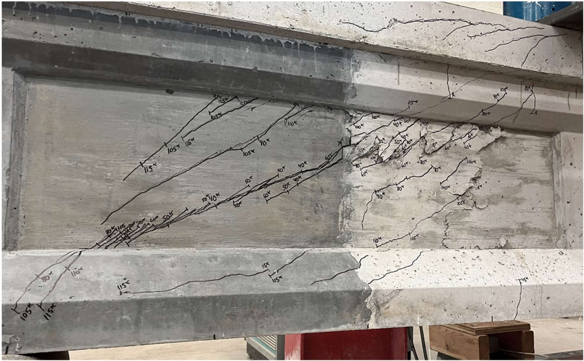
Figure 4.27: Failure of 2D textured hybrid girder no. 2
