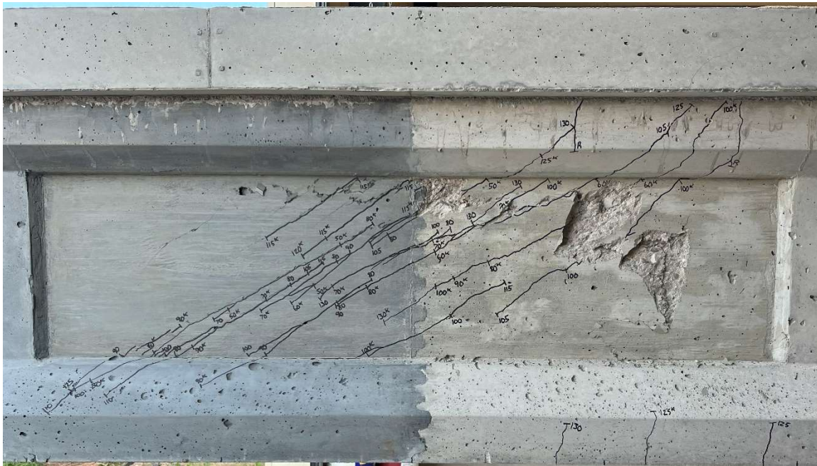
Figure 6.27: Observed, post-testing damage in 3D Trapezoidal Girder No. 2
