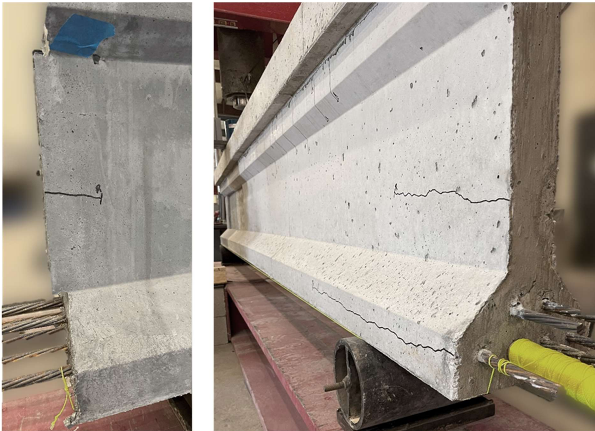
Figure 6.22: Observed cracking due to prestressing forces in 3D Trapezoidal Girder No. 1 (UHPC end (left) and SCC end (right))
