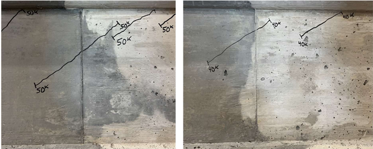
Figure 4.19: First cracks to propagate in BiFluid with Divider girder no. 1 (left) and no. 2 (right)
