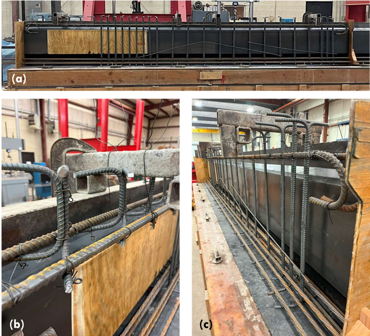
Figure 4.6: Internal reinforcing of hybrid girder before casting, (a) elevation of full hybrid girder reinforcement, (b) short stirrups between the UHPC and deck, and (c) SCC end reinforcement and top bar hooks
