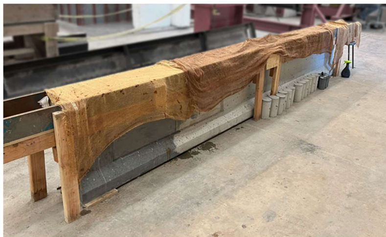
Figure 4.11: Moist curing of deck section of hybrid girder specimen using saturated burlap
