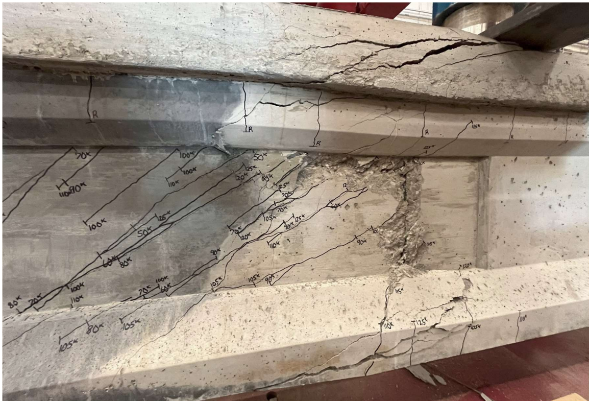
Figure 6.9: Observed, post-testing failure in BiFluid Girder No. 3
