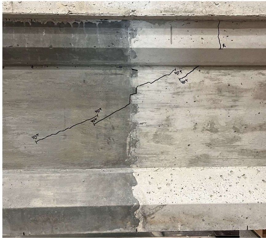
Figure 6.20: Initial cracks observed in 2D Trapezoidal Girder No. 2
