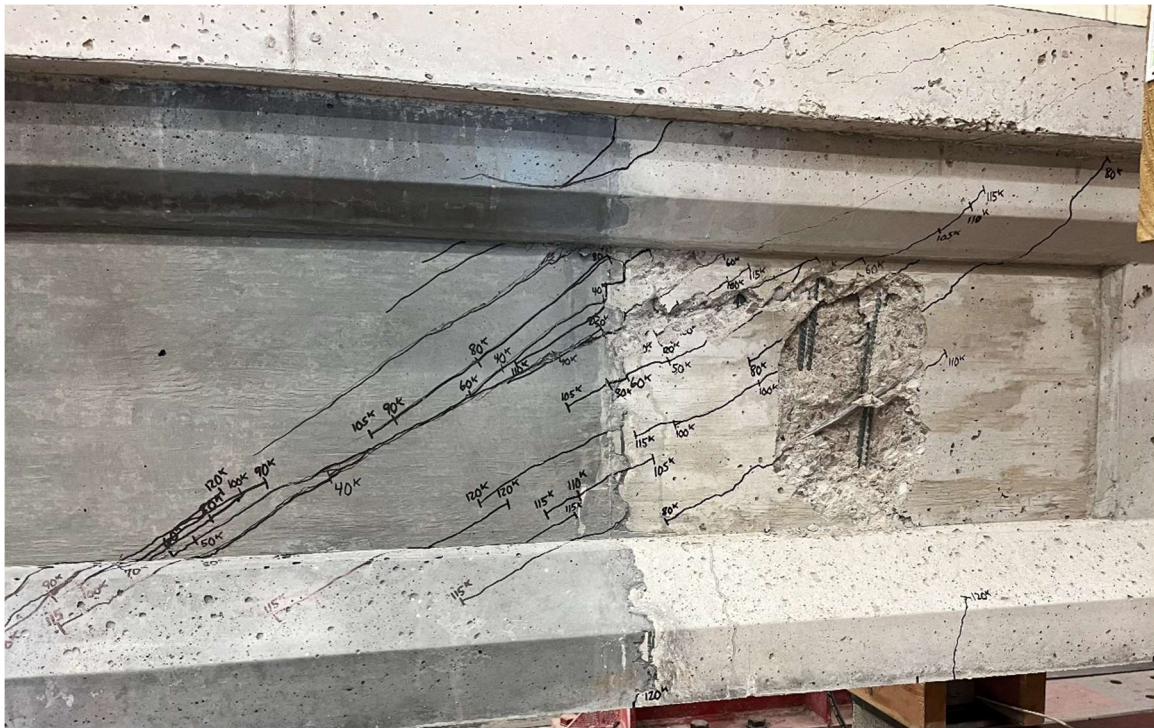
Figure 6.19: Observed, post-testing damage in 2D Trapezoidal Girder No. 1
