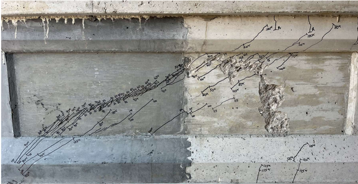
Figure 6.25: Observed, post-testing damage in 3D Trapezoidal Girder No. 1
