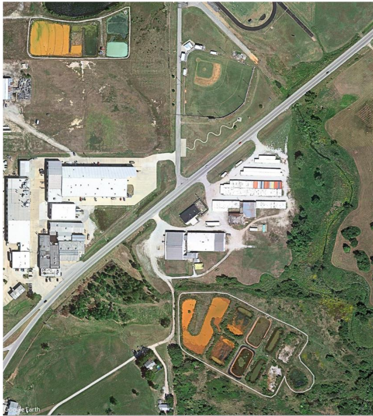
Figure 4-6. Mayer Ranch (bottom right) and Southeast Commerce (top left) passive treatment systems.
