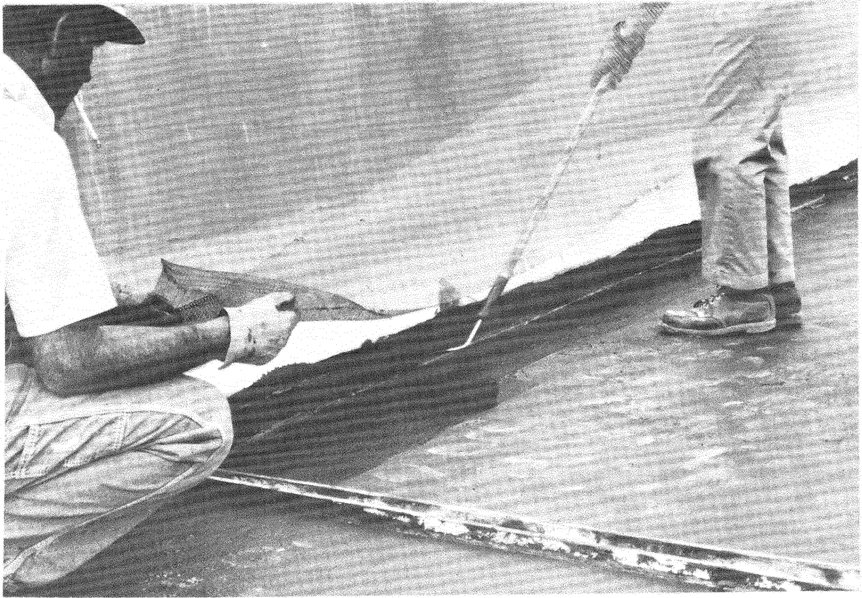
Applying first fabric layer into the second emulsion coat.
