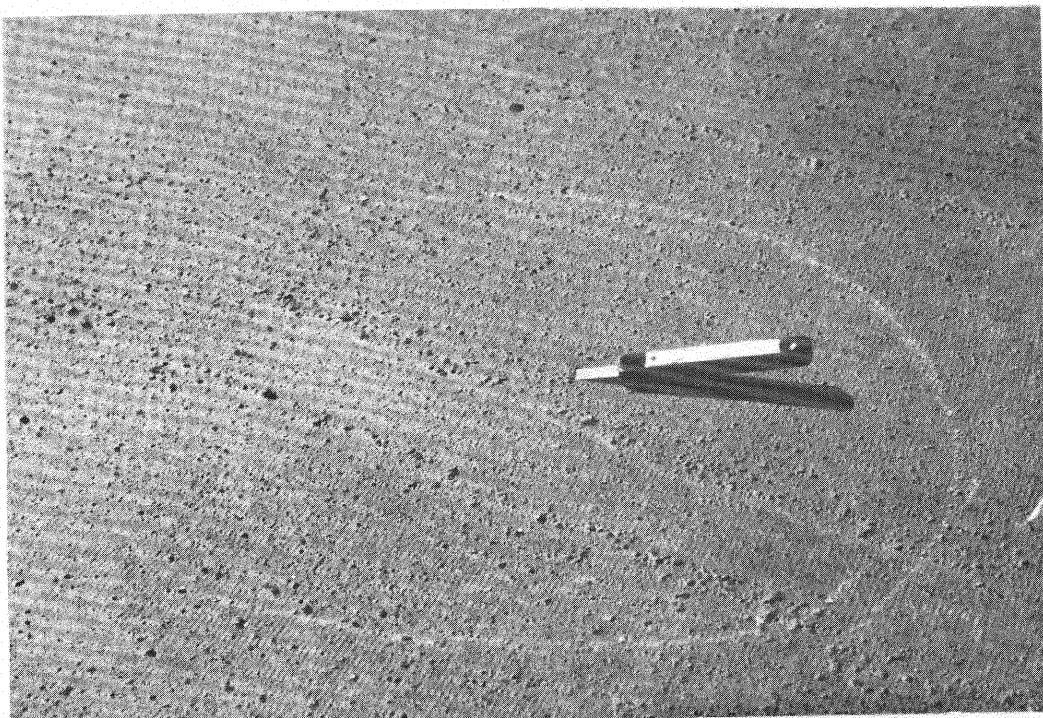
Puncturing and venting blister.
