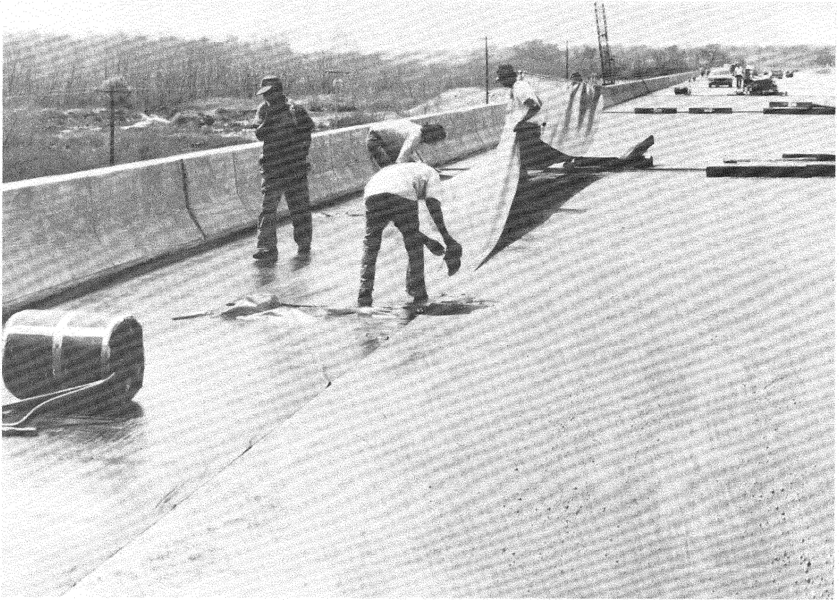
Applying Protecto Wrap to primed surface.
