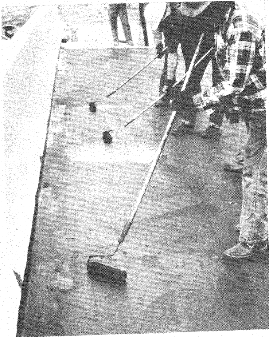
Rolling the fiber glass into the second emulsion coat.
