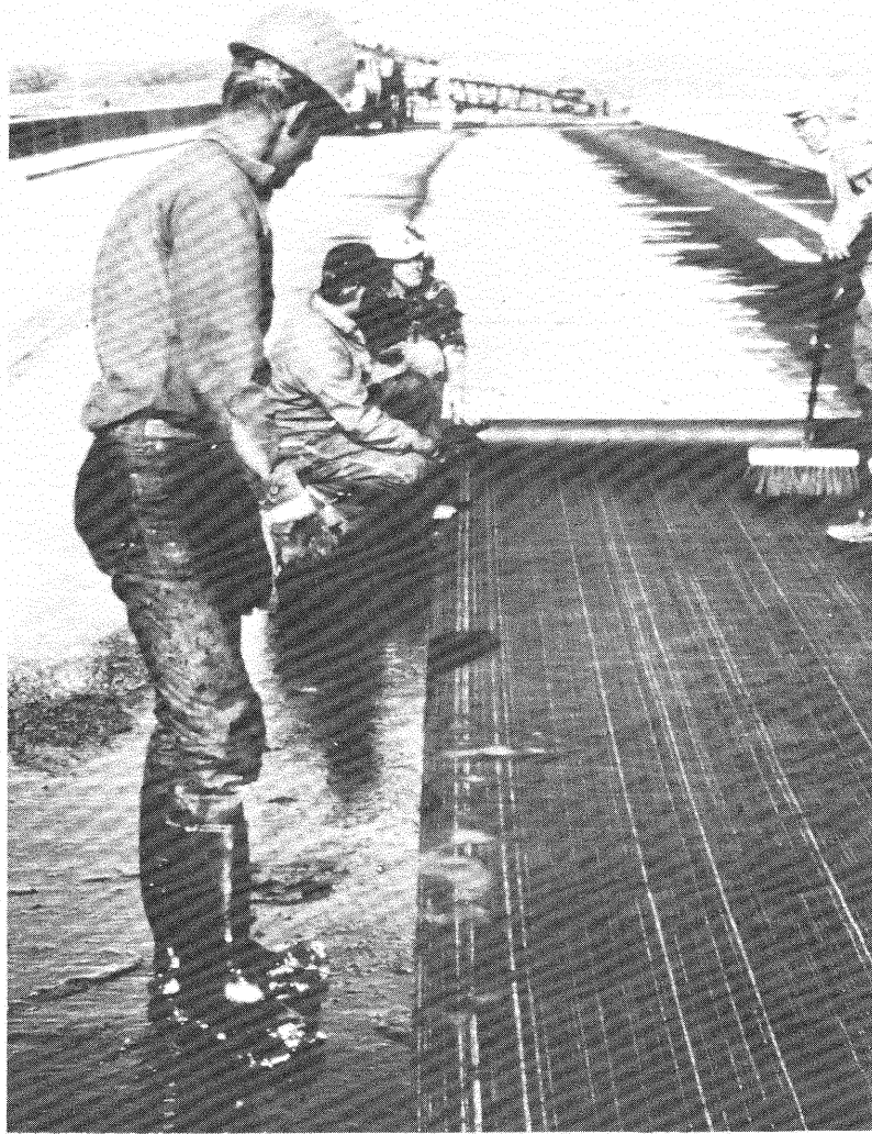
Applying and brooming the Petromat Fabric into the binder.
