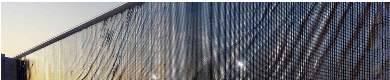
Figure 5. Kinetic membrane of the Brisbane Domestic Terminal Airport Carpark by Ned Kahn. (Terrapin Bright Green, 2014)
