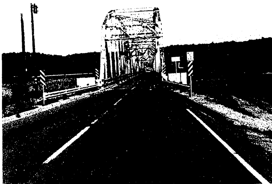
Figure 1. Selected Examples of Bridge Approaches, State of Oklahoma
