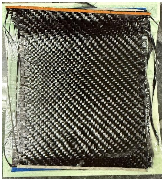
Figure 18: Saturated Carbon Fiber Sheets During Layup
