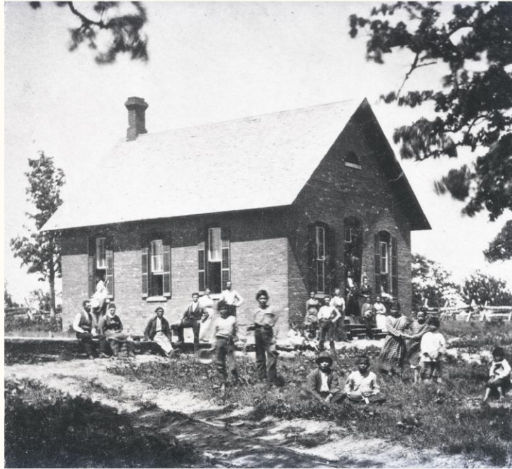
Original school building between 1875 and 1891 (before addition)
