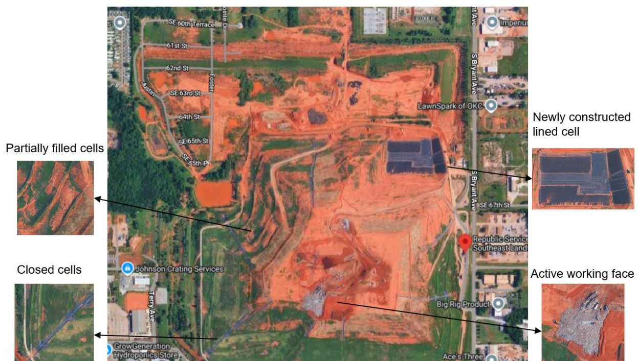
Figure 3.1. Satellite view of Republic Services Southeast Landfill in Oklahoma City.
