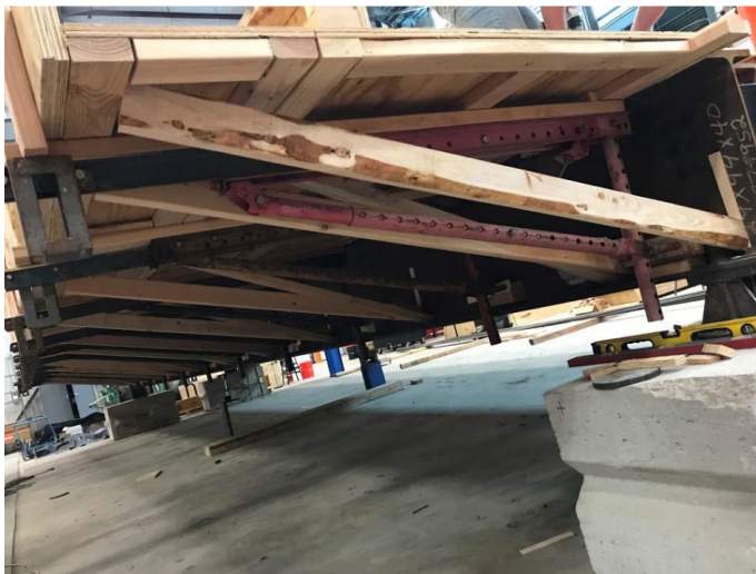
Figure 4.5: Bracing of formwork for the cantilevers. Additional bracing shims were added to help reduce construction deflections.
