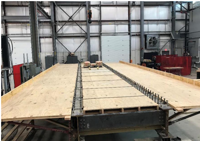
Figure 4.3: Formwork being prepared for casting the bridge deck on the prototype bridge
