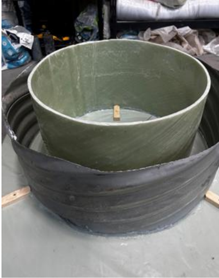
Figure 46: Using GE advanced silicone to seal the inside of the GFRP pipe and outside of the steel pipe
