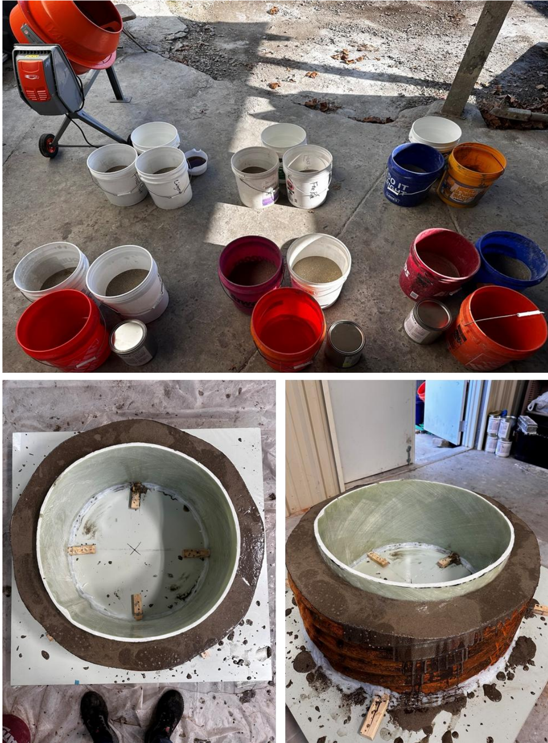
Figure 48: Polymer grout mixing and curing setup, showing prepared grout batches in buckets with the mixer (top) and the slip-lined specimens immediately after polymer grout placement while curing on the support plates (bottom).
