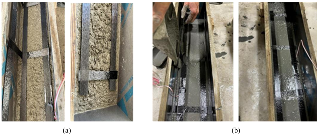
Figure 76: Fabrication of (a) PCC beams and (b) UHPC beams
