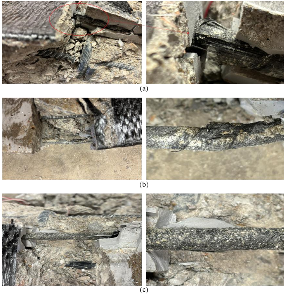
Figure 22: Various failure modes of RC beams strengthened with NSM-CFRP, (a) type NU beams, failed by the CFRP bar rupture, (b) type NSU beams, failed by the CFRP bar rupture, (c) type NSU beams, failed by sudden spilling of the epoxy cover.
