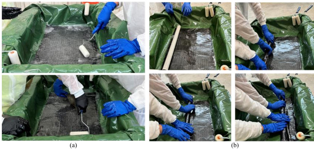
Figure 11: (a) Carbon fiber fabric wetting process for U-wrap. (b) Rolling wet fabric onto plastic pipe for layup on beam.
