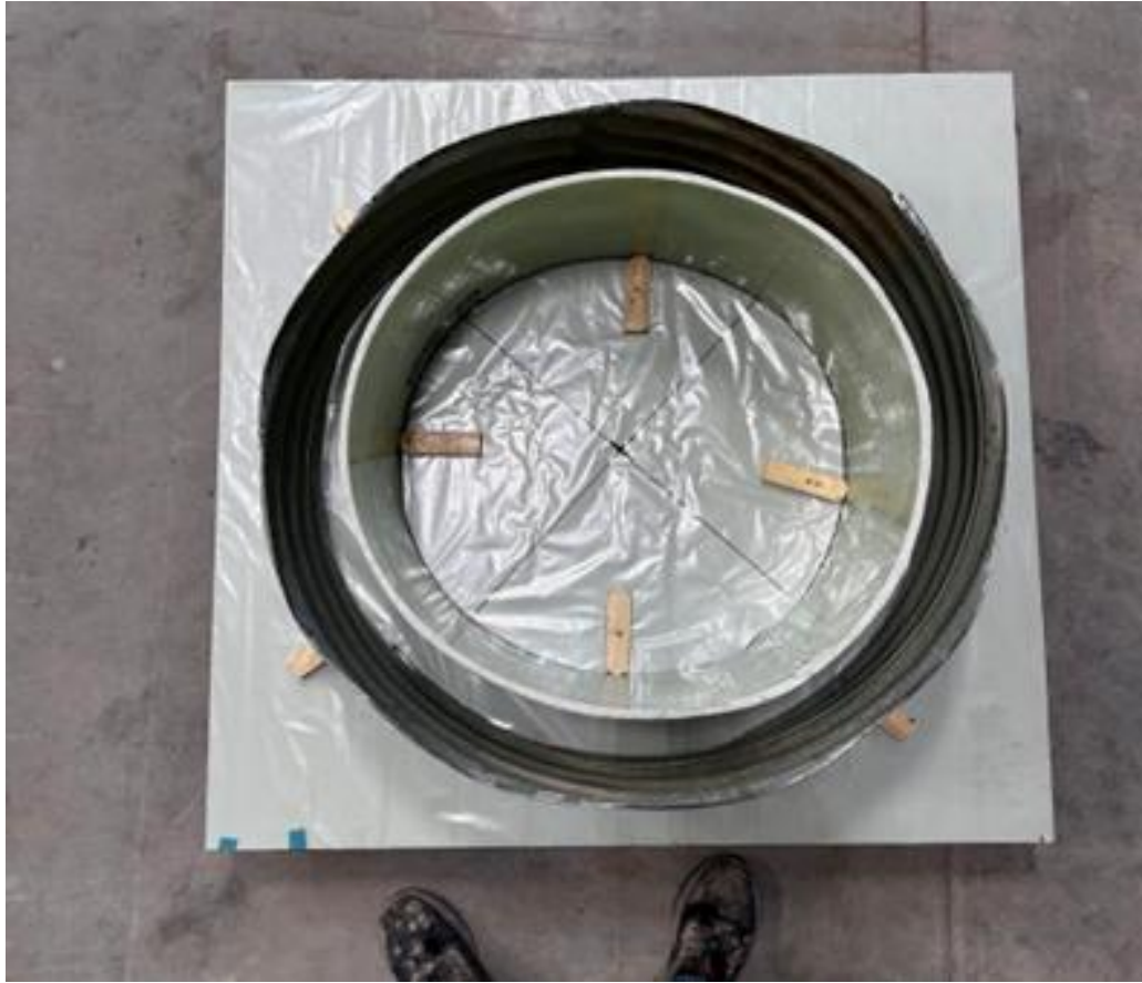
Figure 45: Connecting wood pieces outside the steel pipe and inside the GFRP pipe to hold them in place during casting
