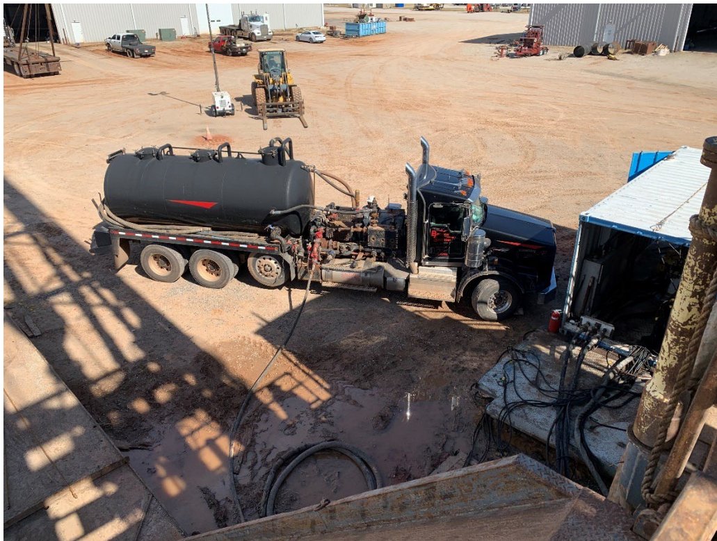
Figure 35. Pump truck used for the pressuring test.
