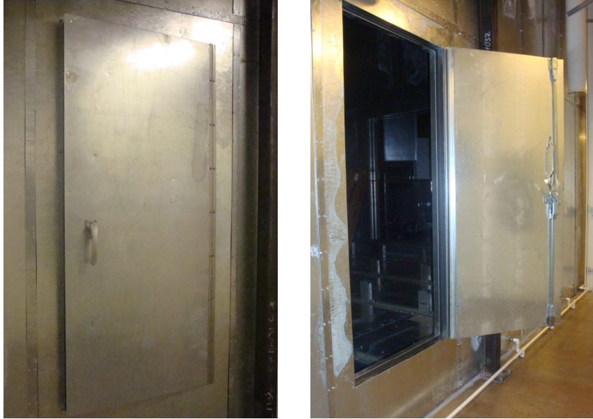
Figure 4.5: Personnel access doors on the west wall
