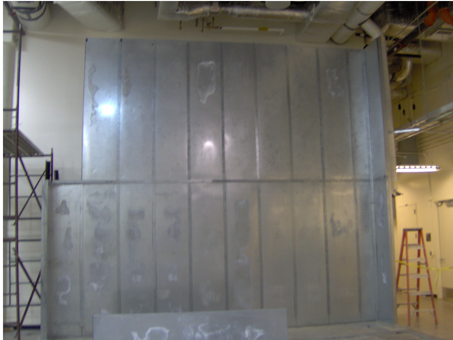
Figure 1.4: Chamber construction begins, erected south wall of chamber
