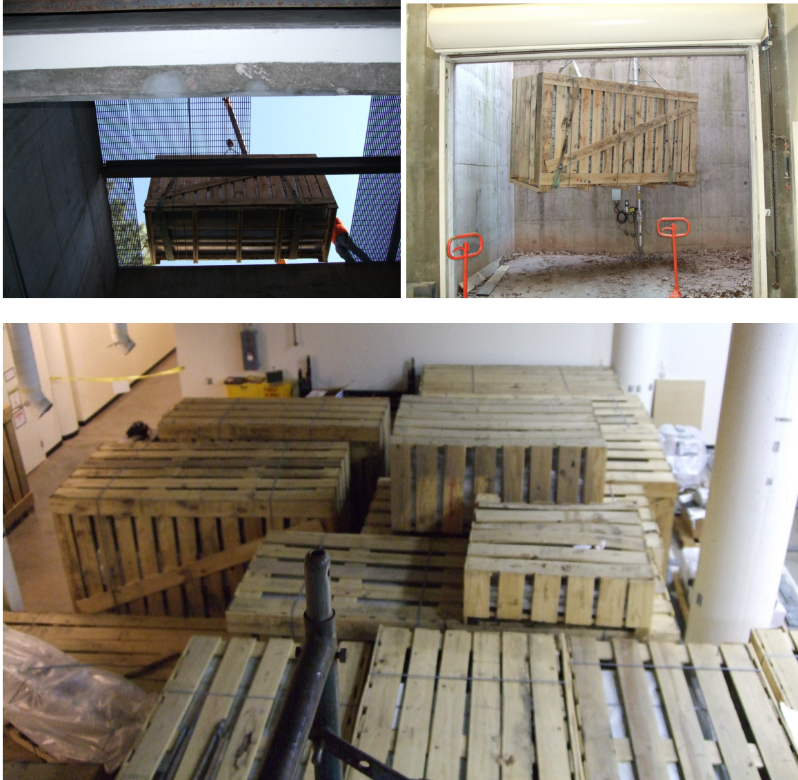
Figure 1.3: Top: lowering the crates into the ATRC basement via the wind tunnel shaft. Bottom: Unopened crates at chamber construction site.
