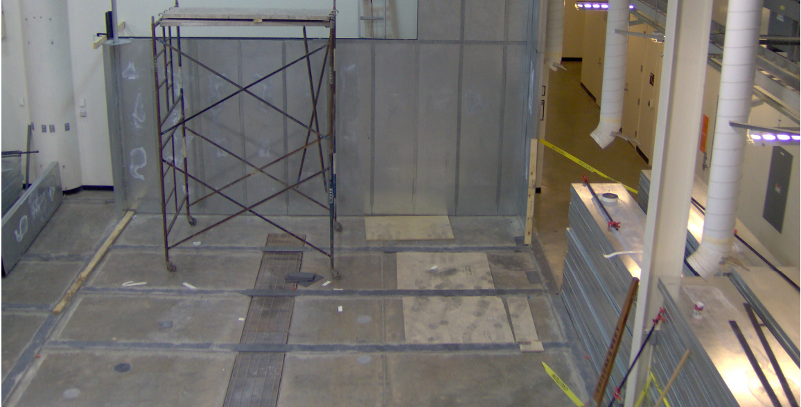
Figure 1.2: Photo showing a portion of the steel floor support for chamber
