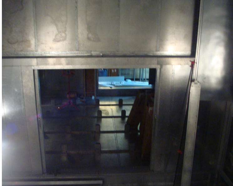
Figure 4.10: Center door – looking from the indoor chamber through the intermediate wall into the outdoor chamber
