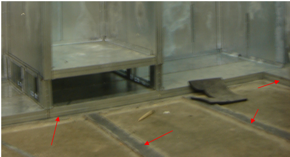
Figure 4.13: Chamber construction on top of base plates; base plates provided level surface for chamber construction
