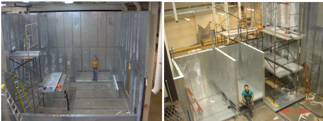
Figure 1.5: Chamber construction. Left: Indoor chamber walls Right: outdoor conditioning loop
