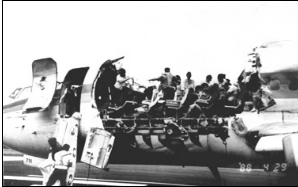
Figure 1 – Aloha Airlines Flight 243, Boeing 737, explosive decompression failure; approximately 18 feet length of cabin lost in flight. Aircraft was safely landed; miraculously only one fatality resulted (28 Apr 1988). [11]
