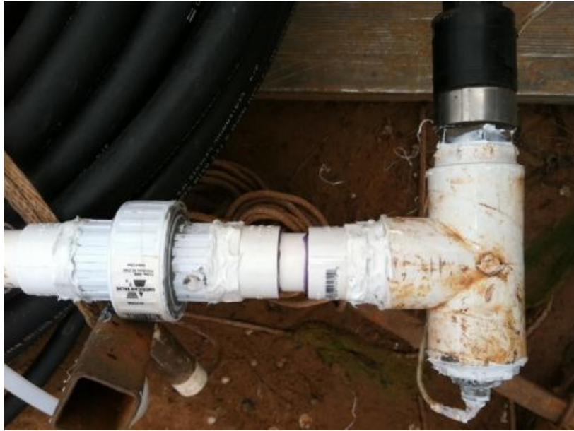
Figure 2-33. PVC Union Coil Connection
