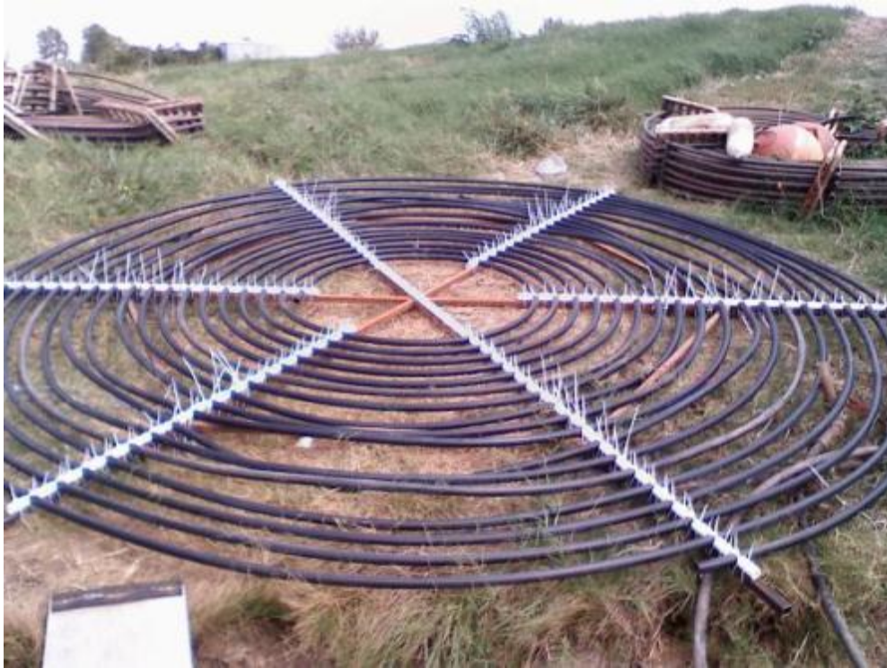
Figure 2-21. Flat-Spiral Coil
