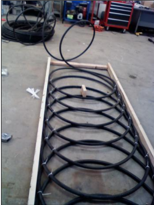
Figure 2-22. Slinky Coil Assembly Guide Rails
