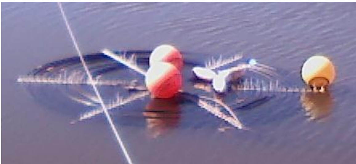
Figure 2-5. Flat-spiral Coil Prior to Submerging
