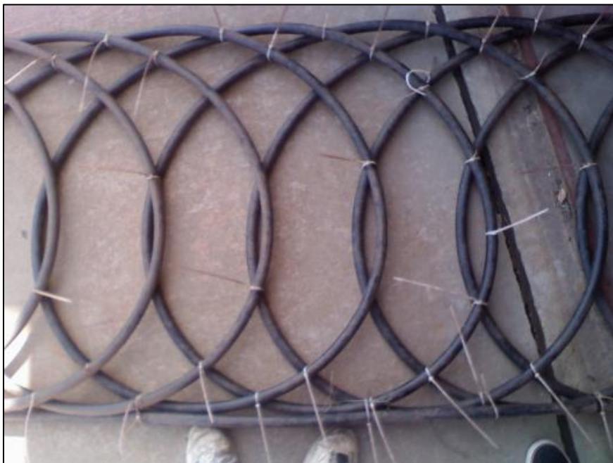
Figure 2-23. Constructed Slinky Coil
