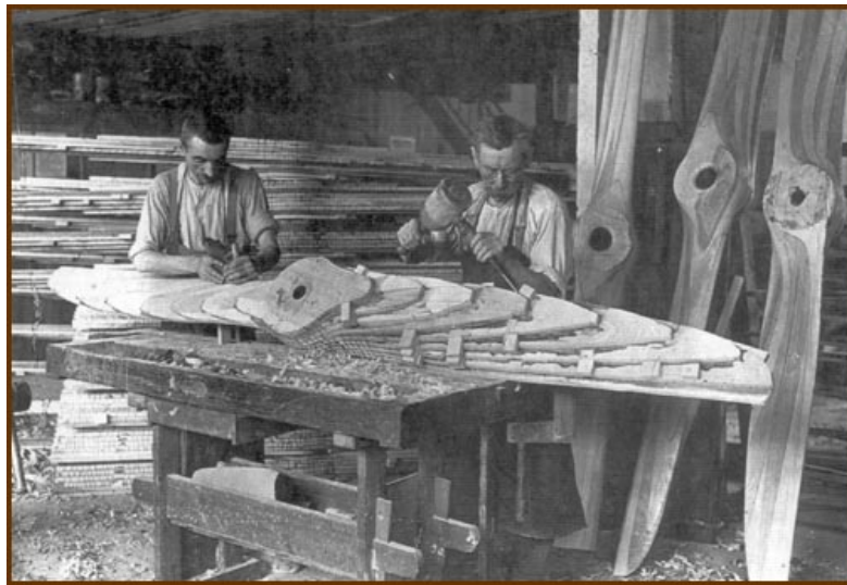
Figure 5 – Wooden laminate with pre-cut layers (Bahnsen 2011)
