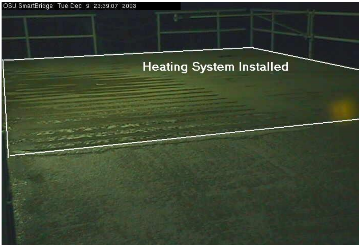
Figure 4-7: Event 1 Bridge Snapshot at 23:39, 12/9/2003 (Snow, +7 hours)
