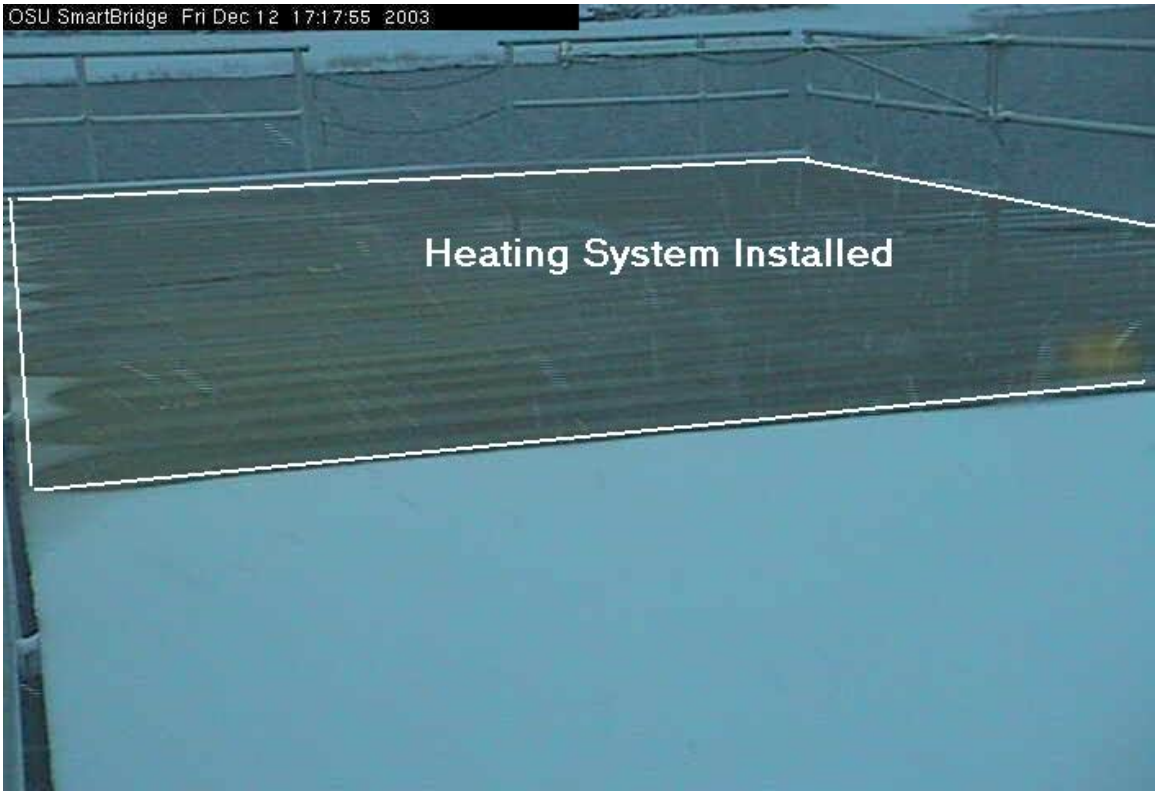
Figure 4-13: Event 2 Bridge Snapshot at 17:17, 12/12/2003 (Snow, +2 hours)
