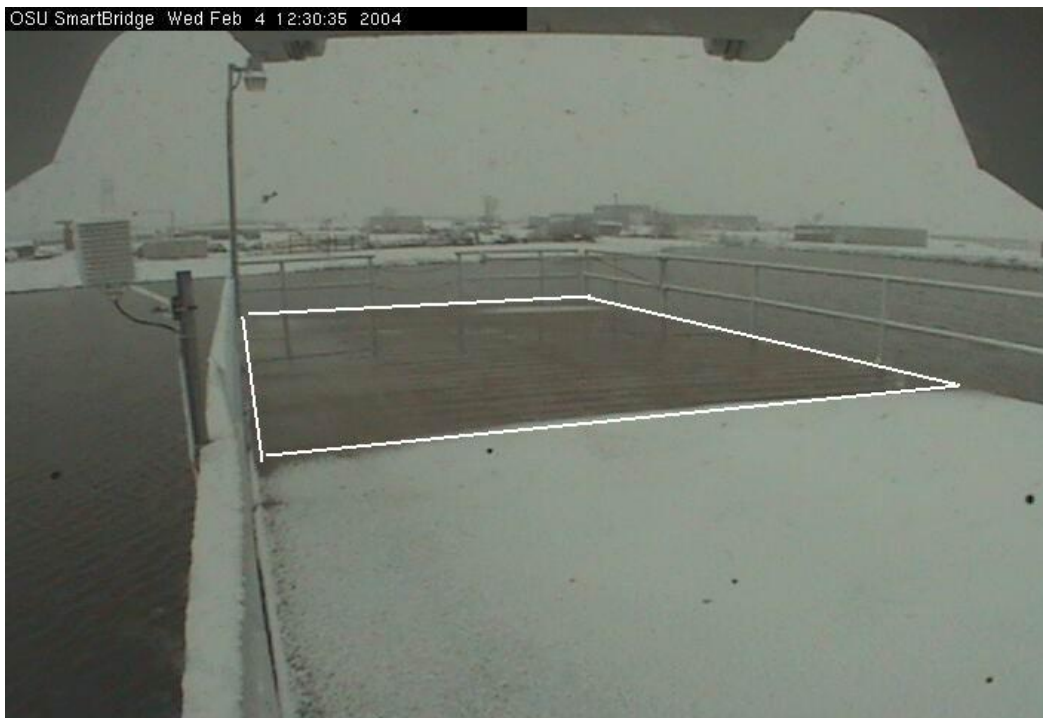
Figure 4-25: Event 4 Bridge Snapshot at 12:30, 2/4/2004 (Snow, +2 hours)
