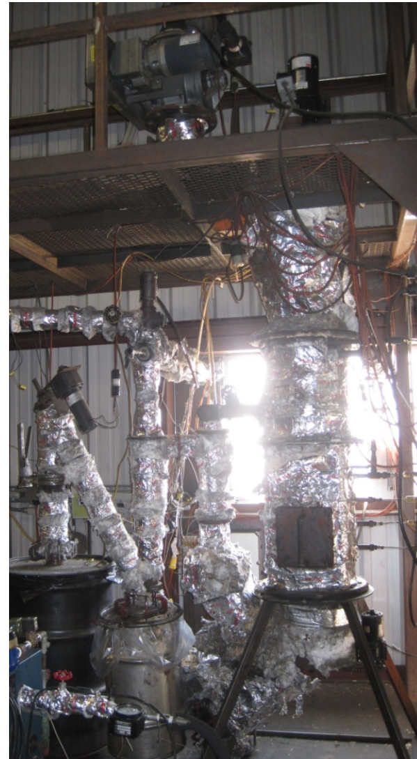
Figure 2.3 Downdraft gasifier system at Oklahoma State University
