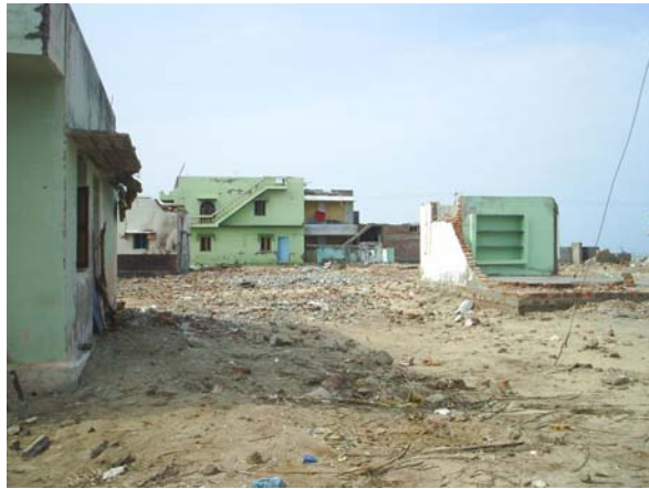
Photo 1: Destruction in Nagapattinam
