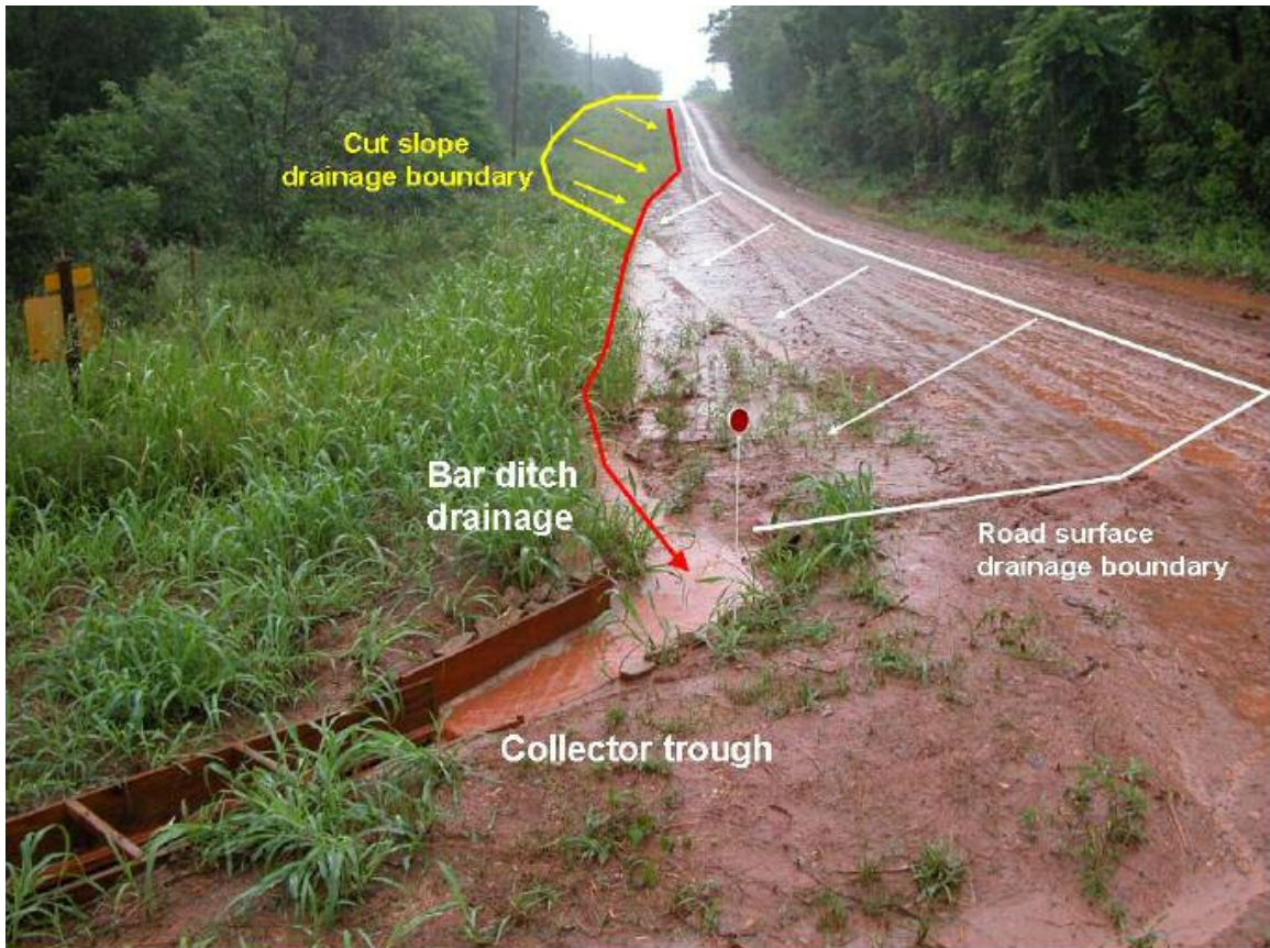
Figure 3. View of westward draining road segment (32 NE) at the 32 nd St. site with drainage boundaries drawn in.
