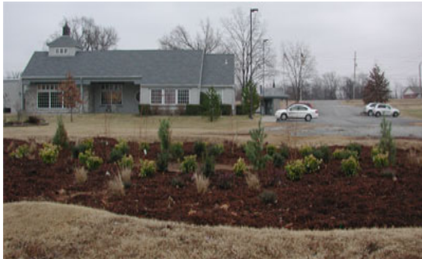
Figure 11: Bioretention cell in Grove, Oklahoma
