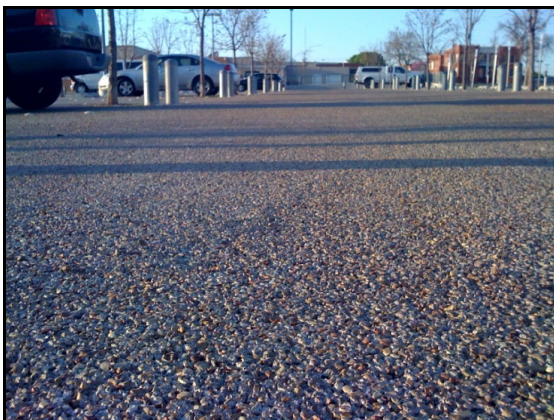
Figure 25: Oklahoma Federal Building pervious parking lot
