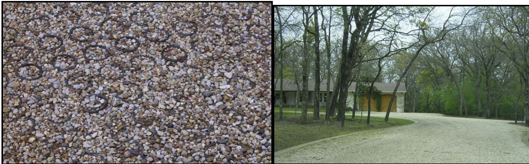
Figure 24: Permeable geogrid system at Silver Tree Interiors in Edmond, OK
