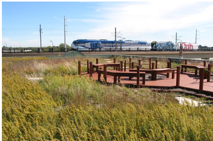
Figure 31: Extensive green roof in Minneapolis, MN Source: ( www.greensroofs.com )
