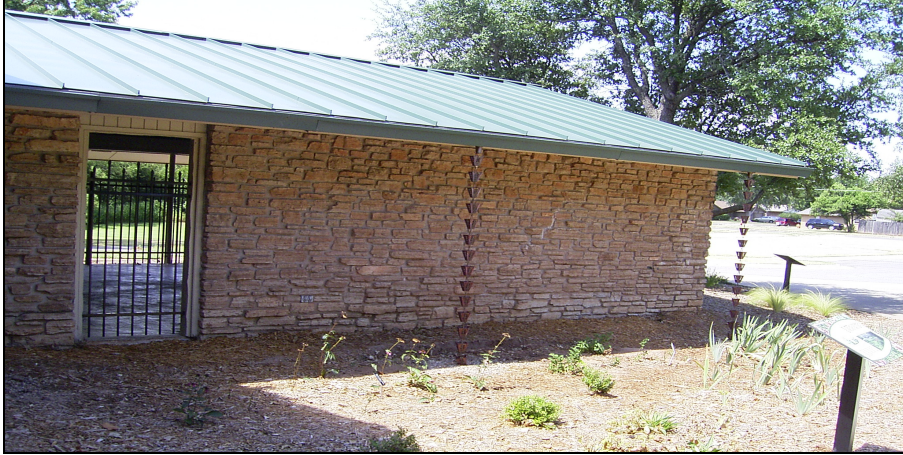
Figure 14: Rain garden at Xeriscape Demonstration Garden in Edmond
