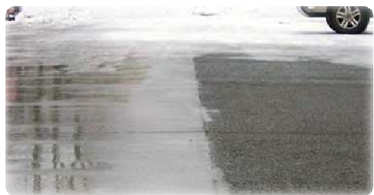
Figure 23. Comparison of standard concrete (left) with pervious concrete (right) after snow plowing ( http://www.go-explore-trans.org ).
