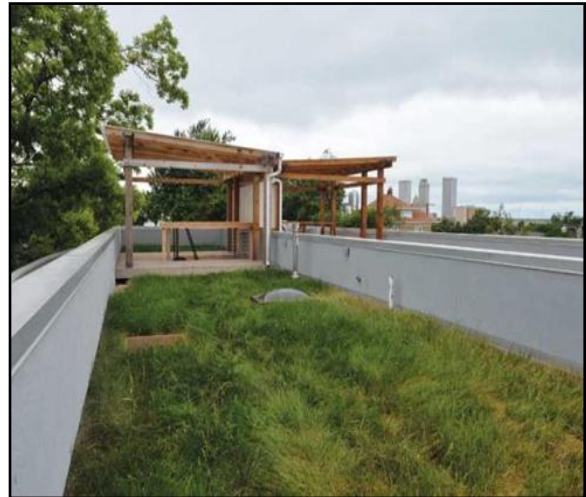
Figure 35. Green roof at Tulsa Lofts in Tulsa, Oklahoma ( http://coolcounter.wordpress.com ).
