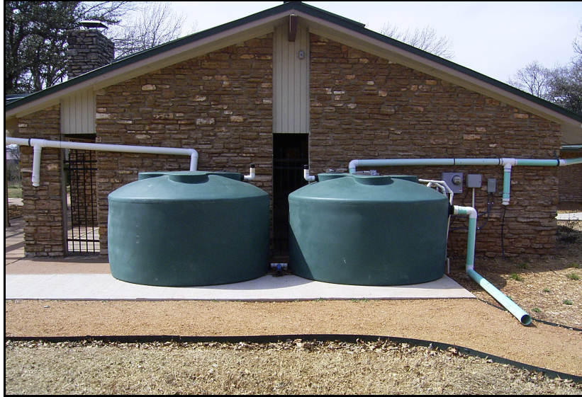
Figure 19: Rainwater harvesting system capable of capturing 2,200 gallons at the Xeriscape Gardens in Edmond, Oklahoma
