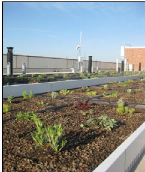
Figure 34: Experimental green roof on the National Weather Center in Norman, Oklahoma (Reid Coffman, University of Oklahoma)
