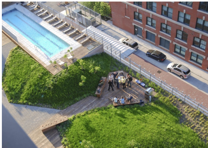
Figure 33: Intensive green roof in Boston, MA Source: ( www.greenroofs.com )
