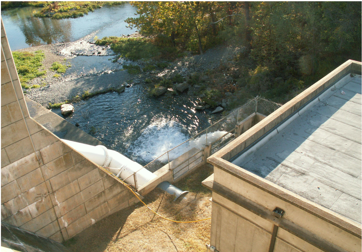
Figure 9: Overflow Pipe at the Spavinaw Dam
